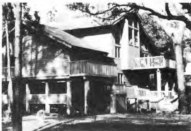
Figure 4.3. Elevation by Posts
