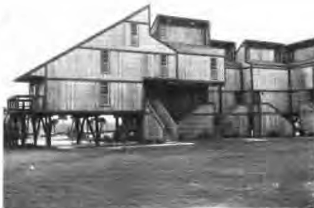
Figure 4.4. Elevation by Posts
