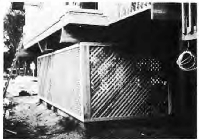
Figure 4.54. Breakaway Walls
