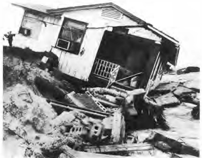
Figure 2.3. Erosion Caused This Foundation to Collapse.
