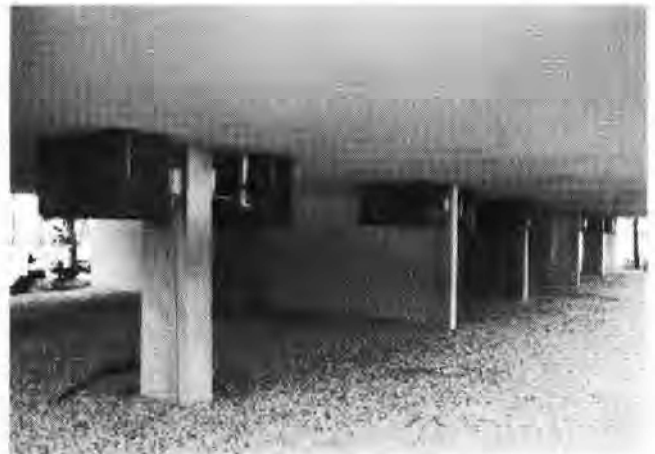
Figure 4.49. Elevated Condenser Units
