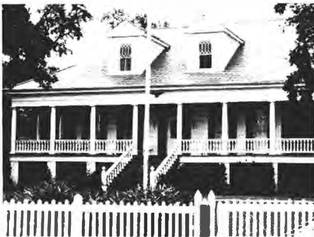
Figure 4.15. Pier Foundations
