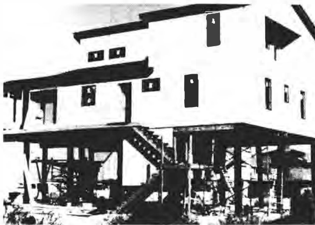
Figure 4.14. Pile Foundations
