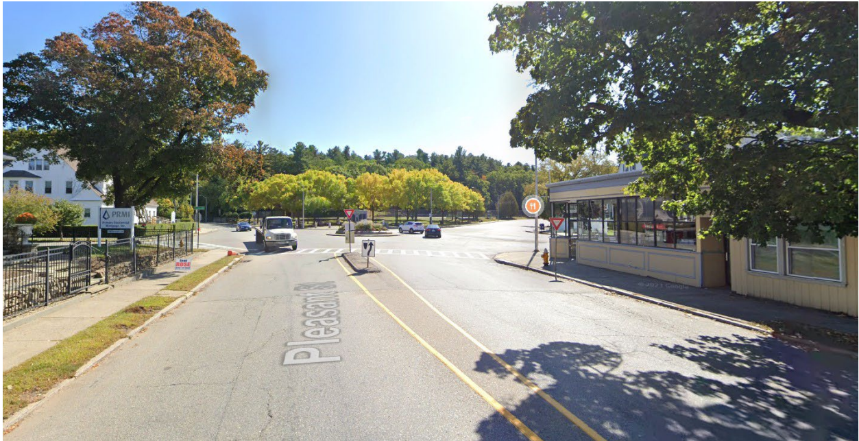
IMAGE 4: Streetview of Pleasant St eastbound approach
