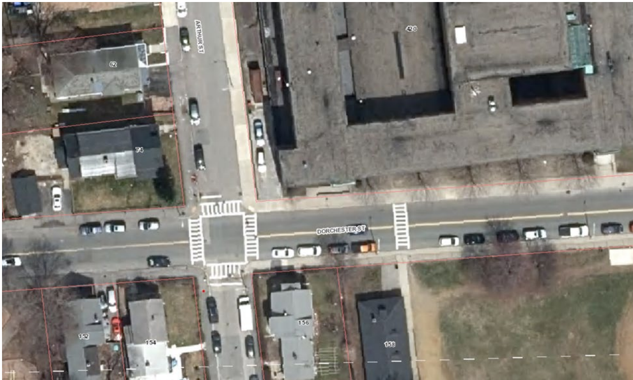
Figure 1: Aerial view of Arthur St-Dorchester St intersection.
