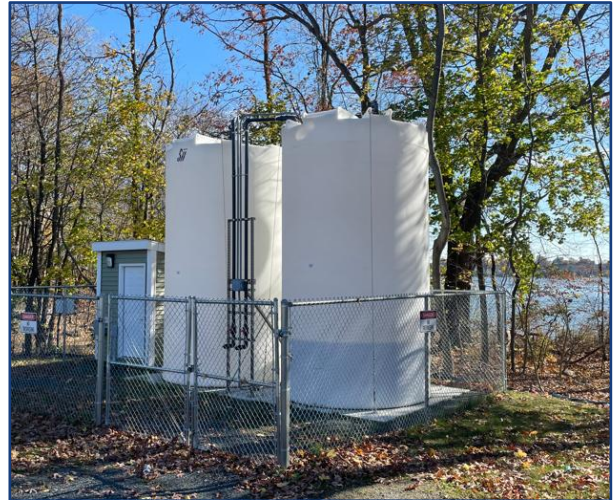
Figure 2 – In 2023, an “Alum Dosing Station” became operational at the lake’s main inlet, Ararat Brook. The station applies small doses of polyaluminum chloride to the mouth of the brook when it rains, immobilizing phosphorous before it enters the lake.
