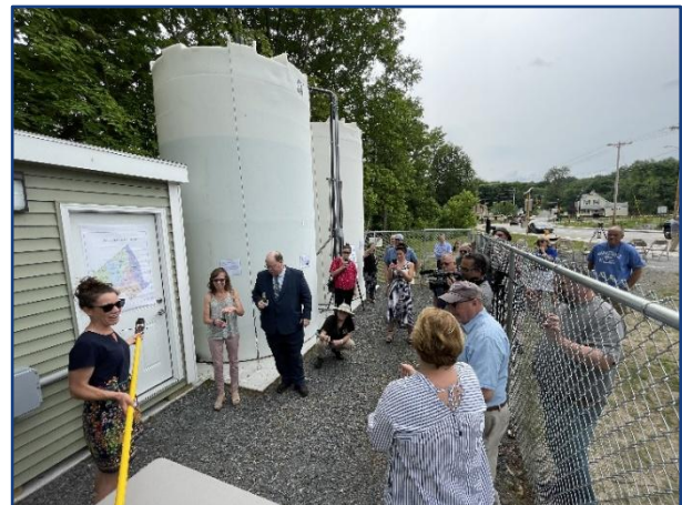
Figure 15 – The Indian Lake Dosing Station became operational in early June of 2023.
