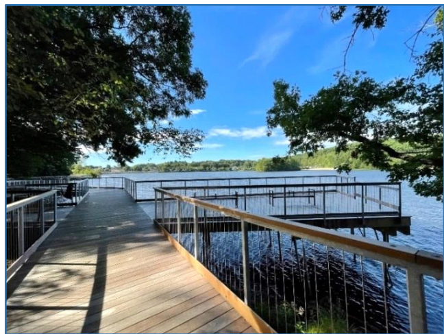
Figure 1 – A newly constructed boardwalk provides universal access to the Eastern shore of Coes Reservoir.
