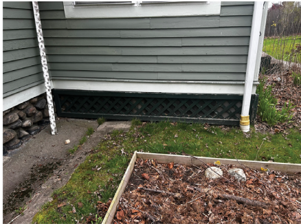
4 BURIED GUTTER AT SE CORNER OF HOUSE
