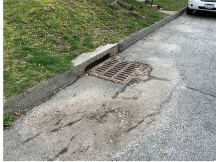
2 CATCH BASIN ALONG VELANDER STREET CAPTURES WATER COMING OFF NORTH EDGE OF PROPERTY
