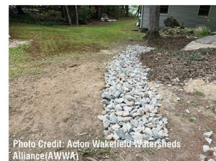
6 INFILTRATION TRENCH
