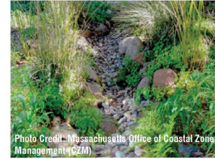
1 VEGETATED CONVEYANCE SWALE
