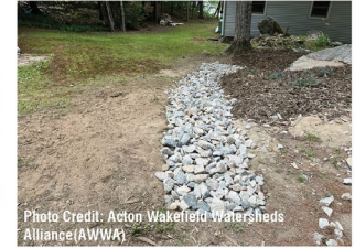
2 INFILTRATION TRENCH
