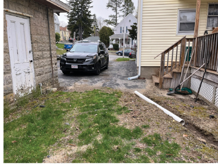
2 HOMEOWNER PLACED PVC & TRENCH FOR DRAINAGE TO BYPASS DECK
