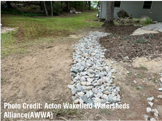
2 INFILTRATION TRENCH
