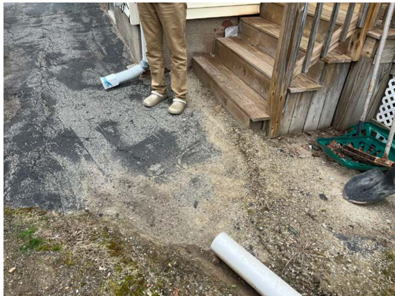
3 EROSION AND WATER DAMAGE AT BASE OF DECK
