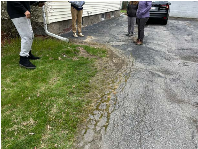
1 WATER POOLING AT DRIVEWAY
