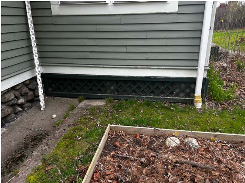
4 BURIED GUTTER AT SE CORNER OF HOUSE
