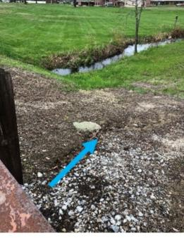
Photo 7-2: Edge of roadway erosion channel.
