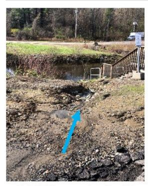
Photo 3-1: Severe erosion adjacent to water access point.
