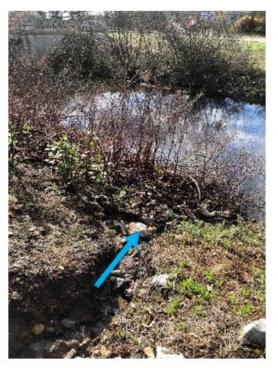
Photo 3-3: Severe erosion adjacent to water access point.
