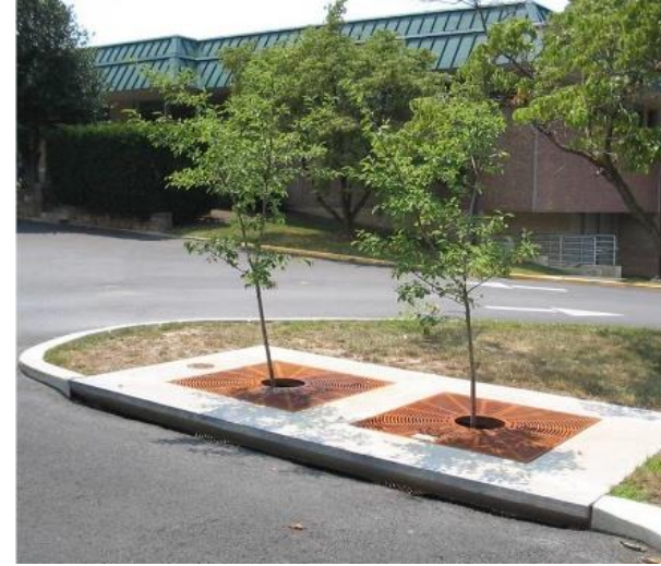
Examples of tree pit filters installed
