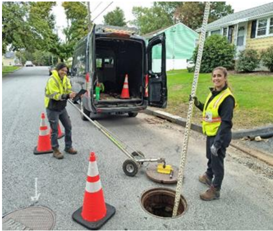
Figure ES-3: Topside Drain Manhole Inspections
