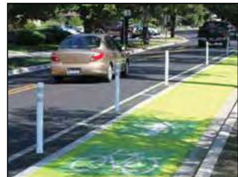
Bike lane and pedestrian walkways
