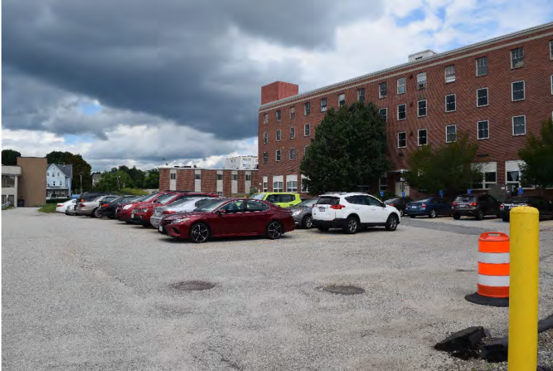
Photo 9: View of the rear of the building complex (1956 addition, first floor in use), looking northeast.
