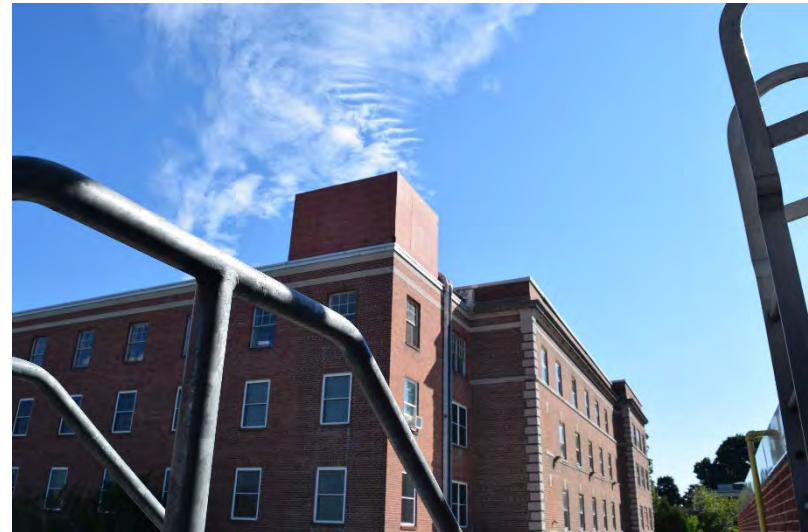
Photo 32: View of Verizon tower on roof of 1956 addition, looking east. Parapet walls along edge of roof.
