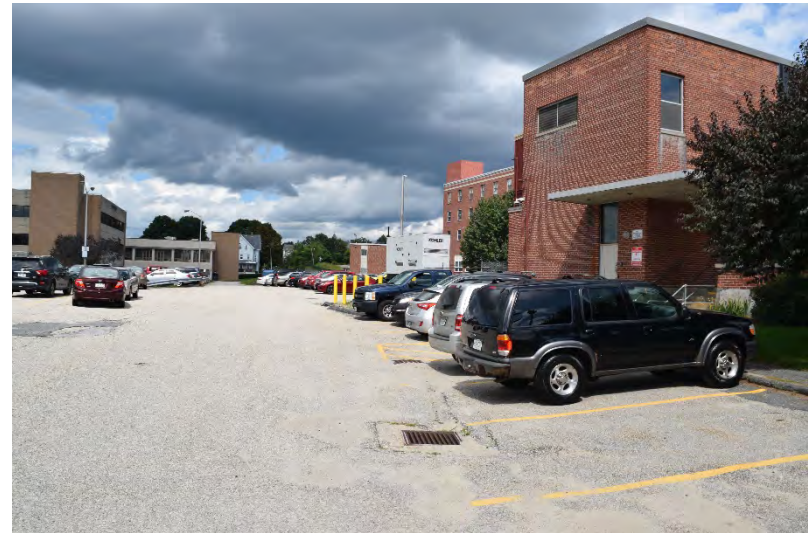
Photo 8: View of the rear of the Senior Center, looking northeast.
