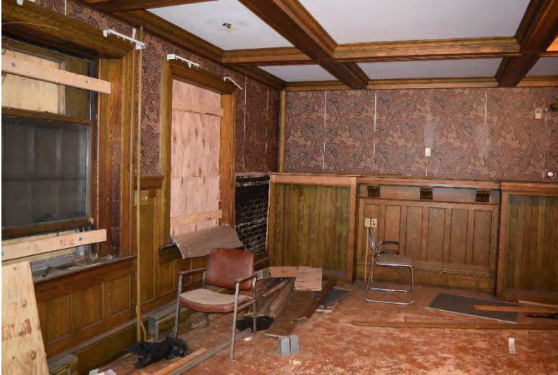
Photo 25: Office room on second floor.
