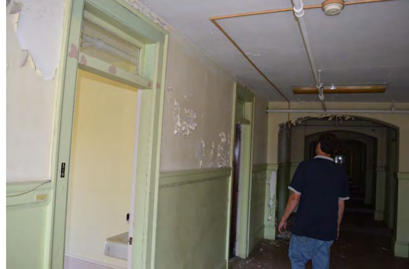
Photo 30: One of the upper floor hallways.
