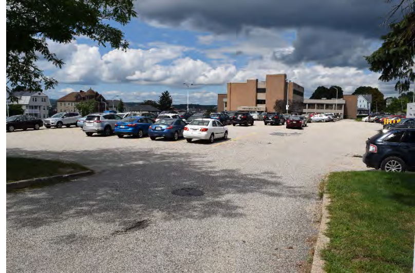
Photo 6: View of the Vernon Medical Center buildings and parking lot for the Worcester Senior Center located immediately west of the subject building.
