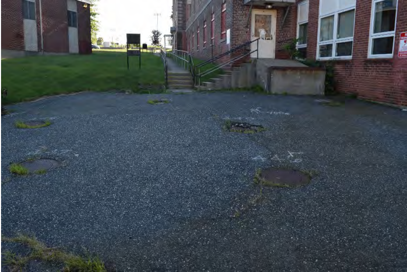
Photo 13: View of the seven manhole covers over the former coal pit, looking east.
