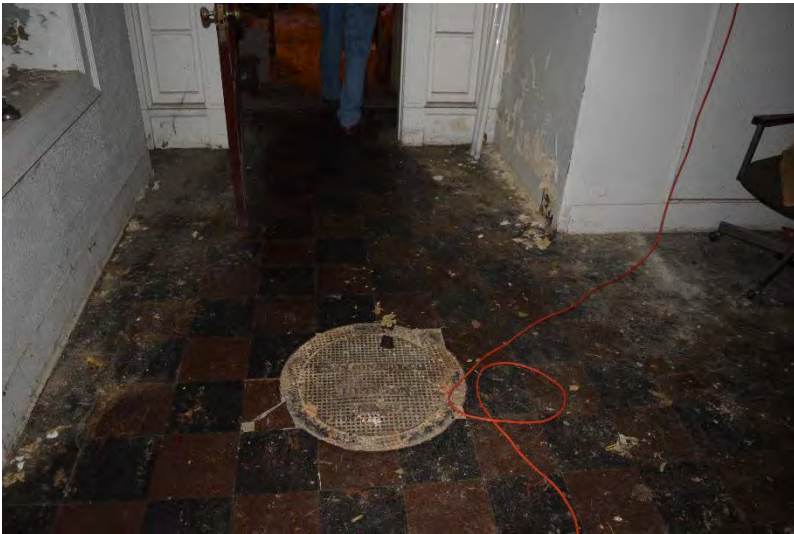
Photo 15: Manhole cover on first floor over utility tunnel.
