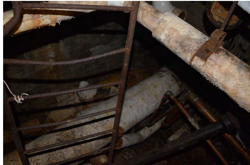
Photo 16: Inside utility tunnel beneath first floor.
