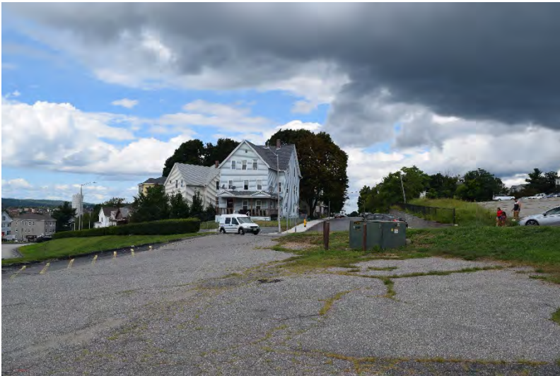
Photo 11: View of Winthrop Street and pad-mounted transformer.
