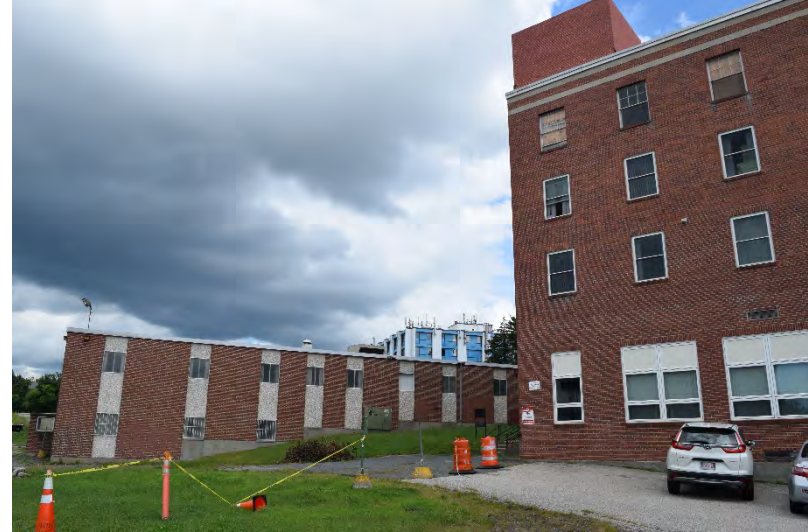
Photo 10: View of the adjacent former Anderson Building and pad-mounted transformer, looking northeast.
