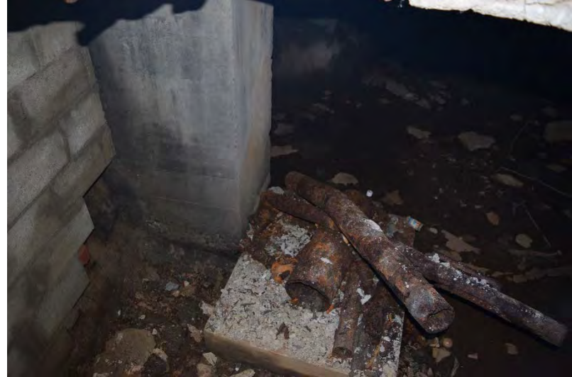
Photo 14: Inside the former coal pit.
