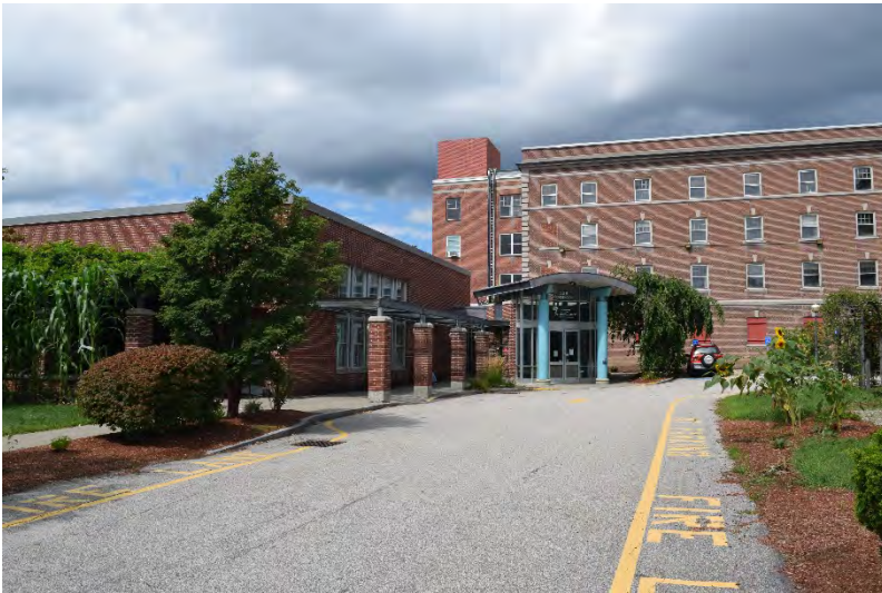
Photo 7: View of the entrance to the Senior Center, looking north.
