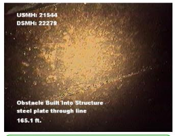
Distance:165.1 ft.Grade:2Condition:Obstacle Built Into StructureRemarks:steel plate through line
