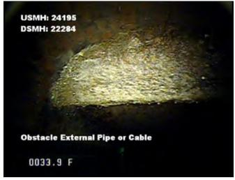
Distance:33.9 ft.Grade:3Condition:Obstacle External Pipe or Cable
