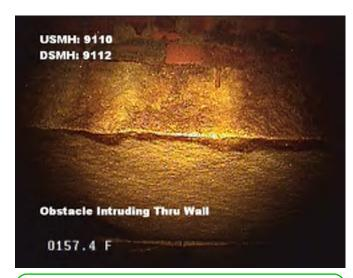
Distance: 157.4 ft. Grade: Condition: Obstacle Intruding Thru Wall
