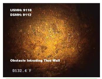
**Distance:** 132.4 ft. **Grade:** 2 **Condition:** Obstacle Intruding Thru Wall
