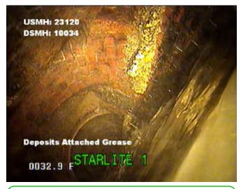
Distance: 32.9 ft. Grade: Condition: **Deposits Attached Grease**
