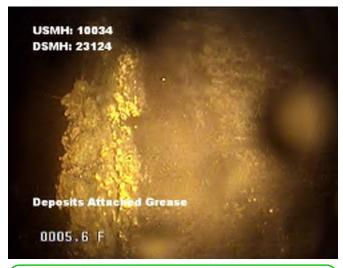
**Distance**: 5.6 ft. **Grade**: 2 **Condition**: Deposits Attached Grease
