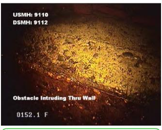
Distance: Grade: Condition: Obstacle Intruding Thru Wall
