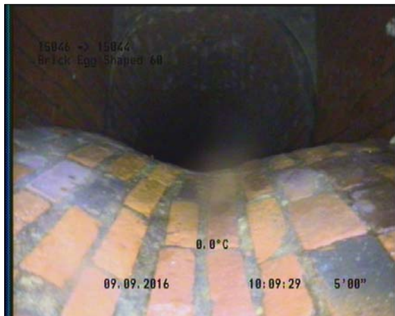
Photo: 15046-15044_09092016_LU_4.9989_101128_A.JPG 5FT, Alignment Up, 25 %
