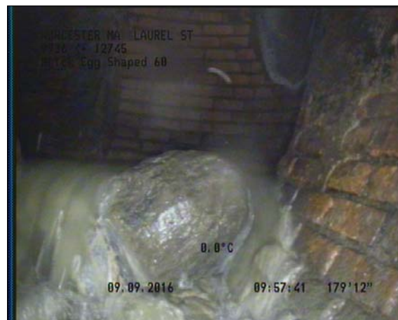
Photo: 12745-9936_09092016_MGO_179.9596_095941_A.JPG 179.96FT, General Observation
