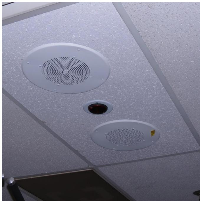
Fig 2 – Bogen 70/25V Recessed Speaker (Mounted)
