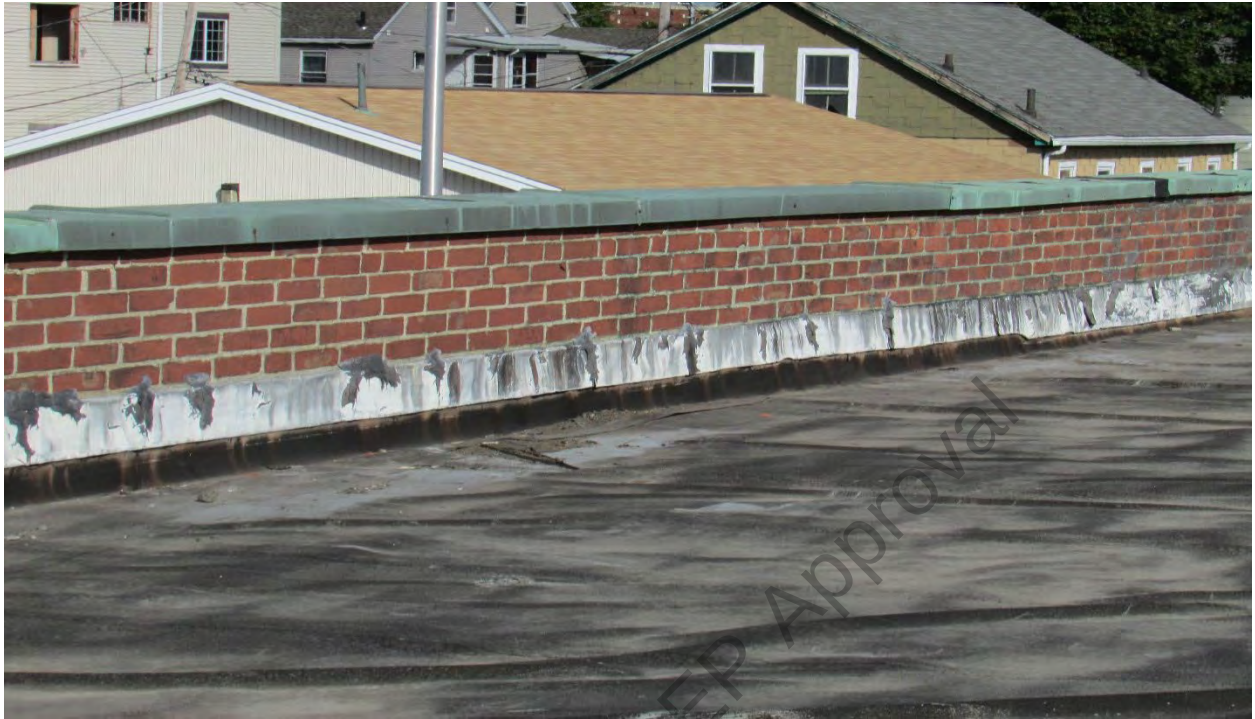
Photo #11 A-Roof Parapet Wall
