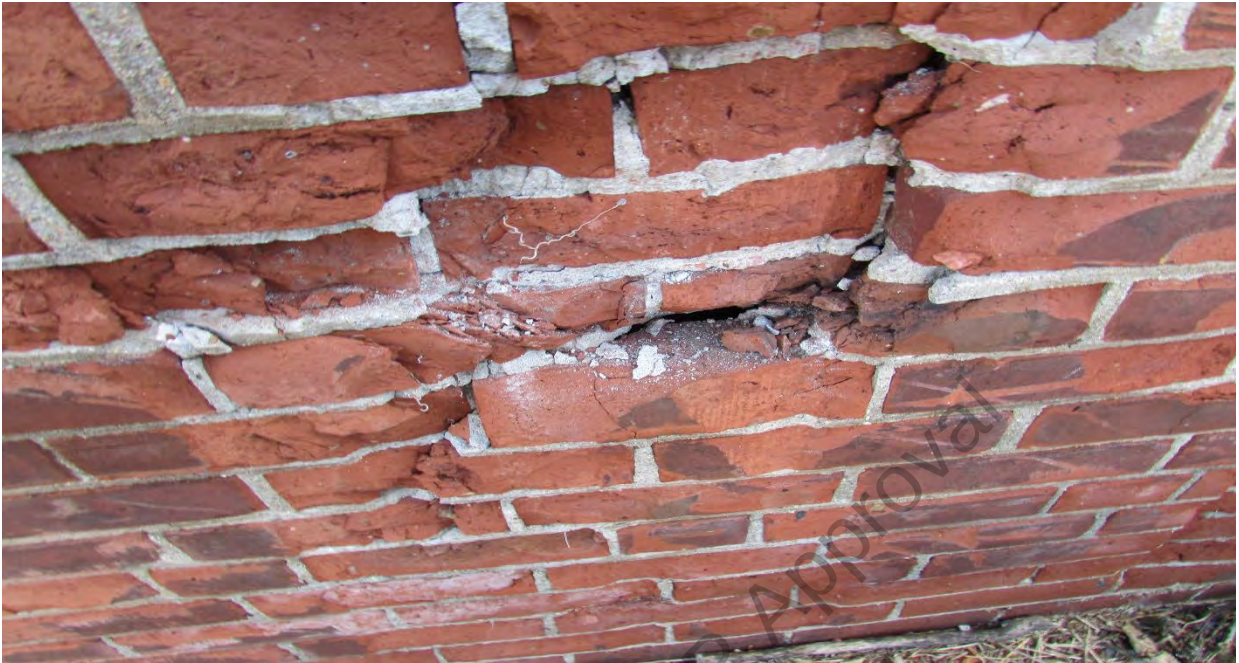
Photo #5 DPW Brick Wall (North Side)
