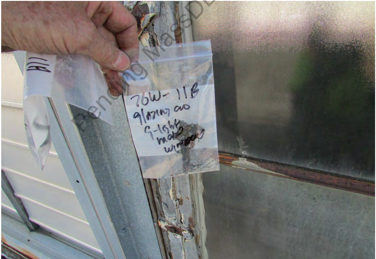
Photo #18 Sample 11A&B Glazing on 9-Light Metal Window (B Roof) (Positive)
