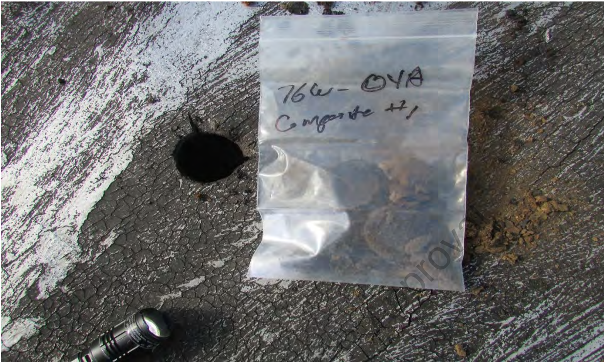
Photo #7 Sample 04A Roof Composite #1 A-Roof
