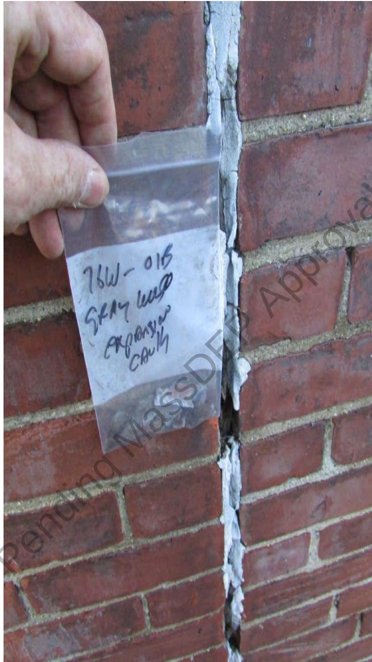
Figure 1- Brick Wall Expansion Caulk
