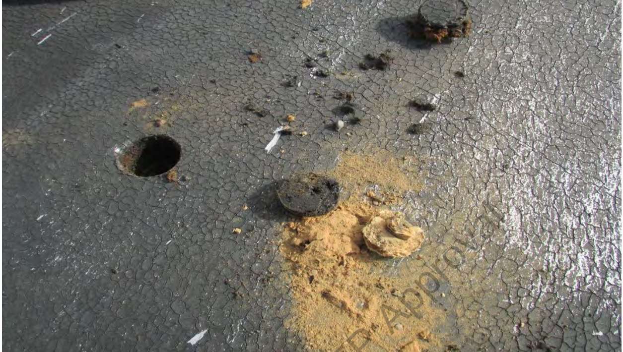
Photo #13 A-Roof Material
