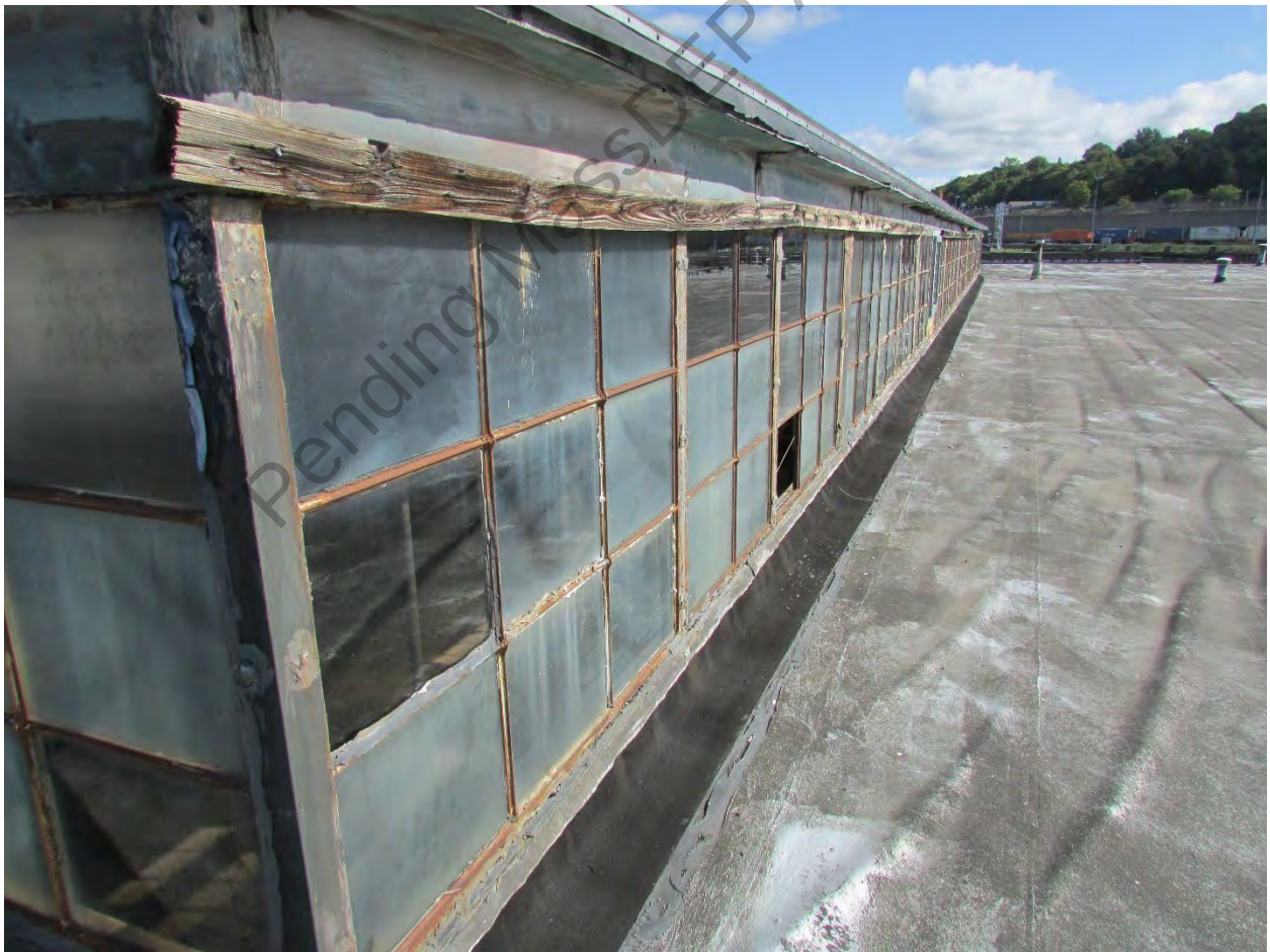
Photo #27 B-Roof West Side
