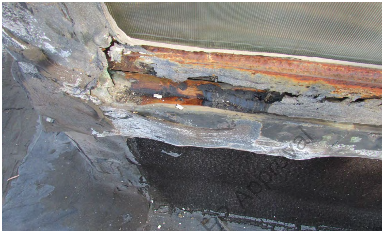
Photo #23 Sample 13A-C Gray Coat on 9-Light Window Frame (Positive)
