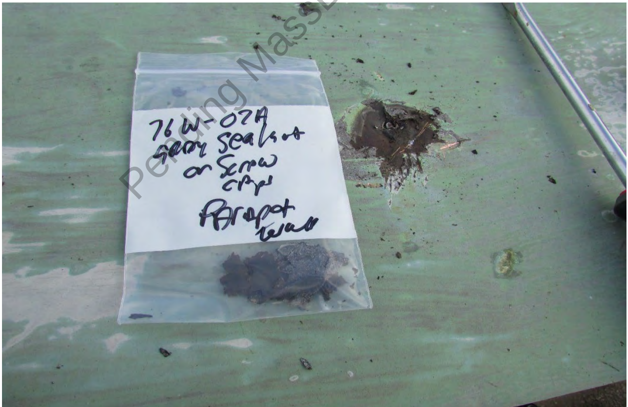
Photo #14 Sample #07A&B Gray Sealant on Screw Caps (Parapet Wall) (Positive)
