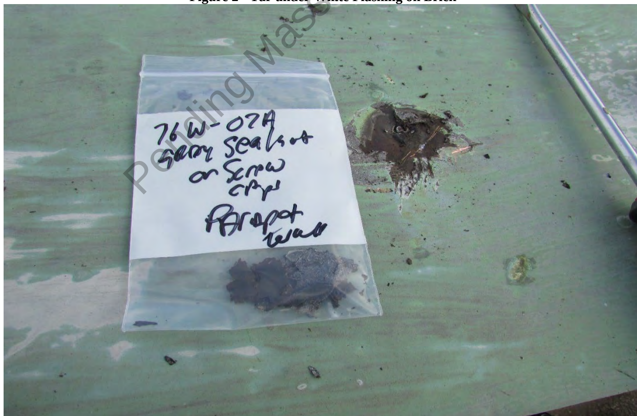
Figure 3 - Gray Sealant on Screw Caps (Parapet Wall)
