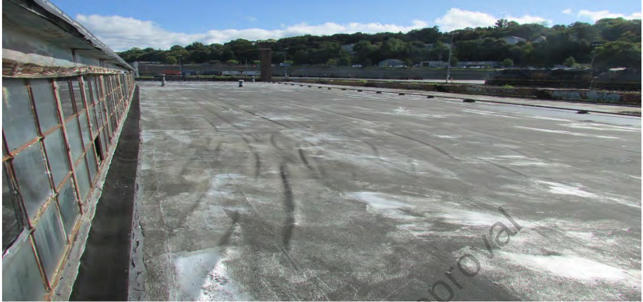
Photo#26 A-Roof West
