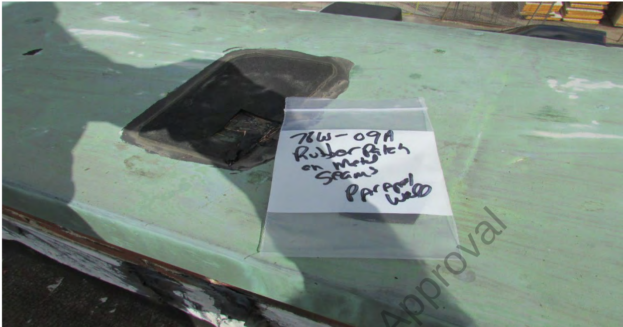
Photo #15 Sample #09A&B Rubber Patch on Parapet Wall Seam
