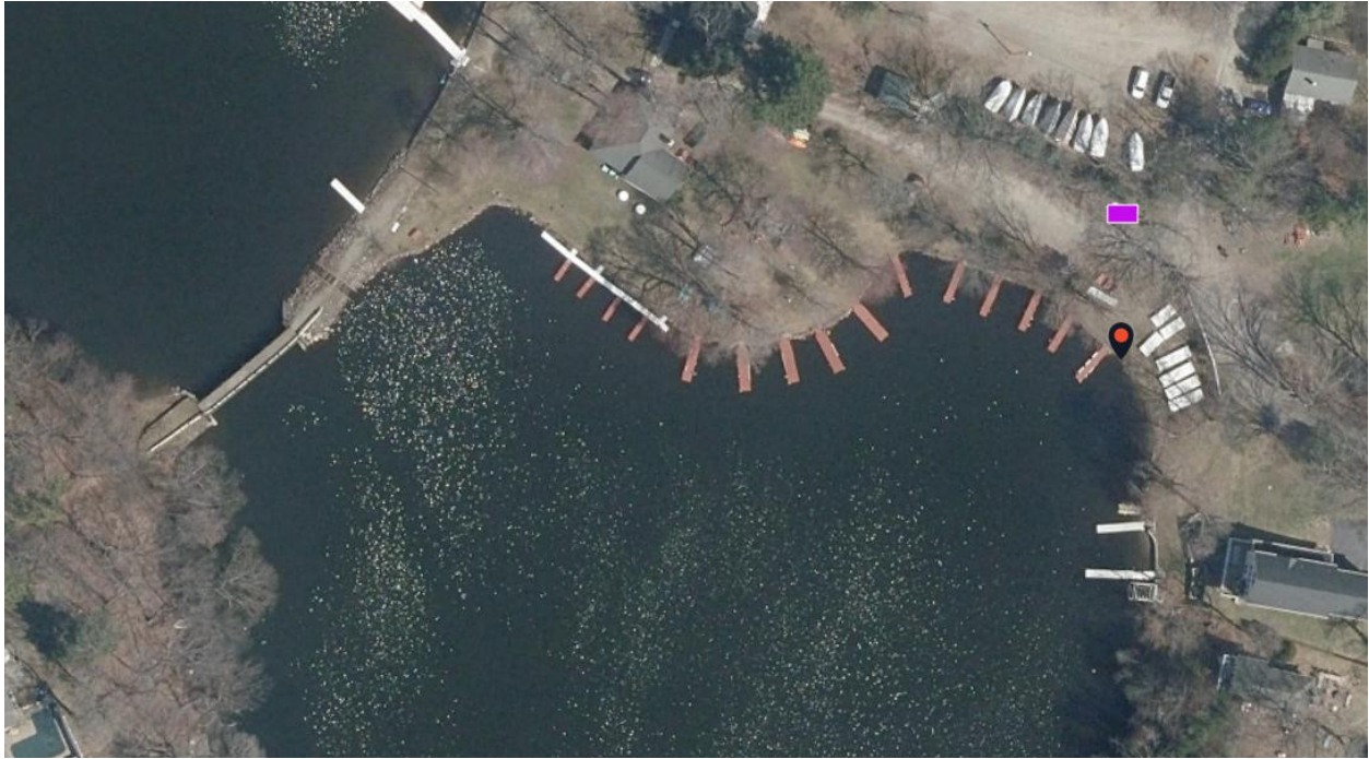
Figure 3. Proposed container location and equipment docking.
