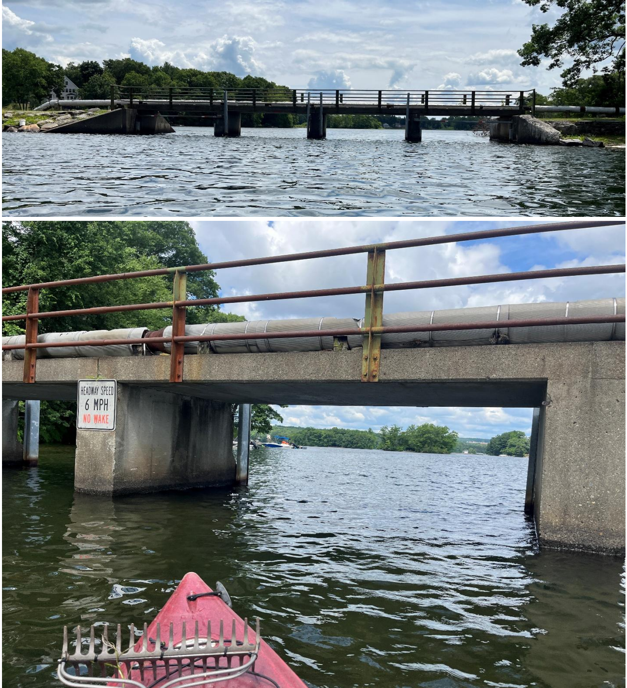
Figure 4. Stringer Dam and approximate air gap.
