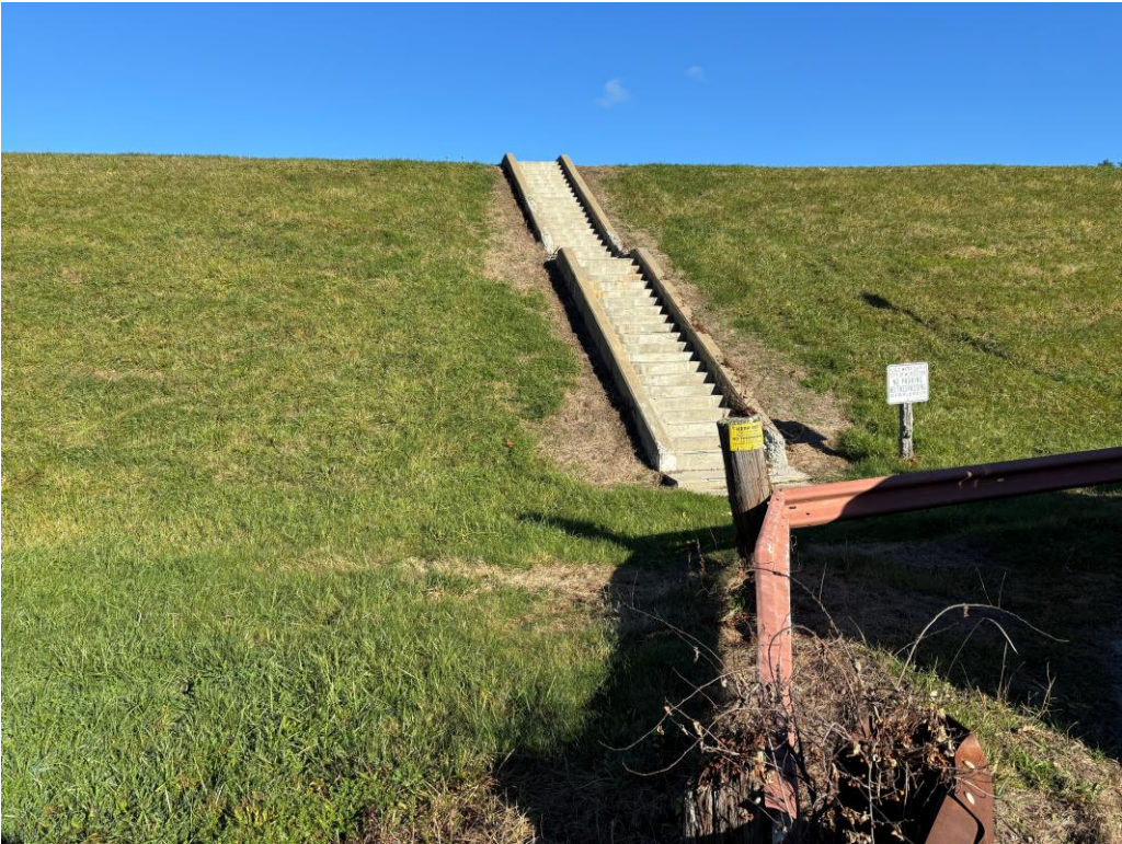
General Condition from Stone House Hill Road
