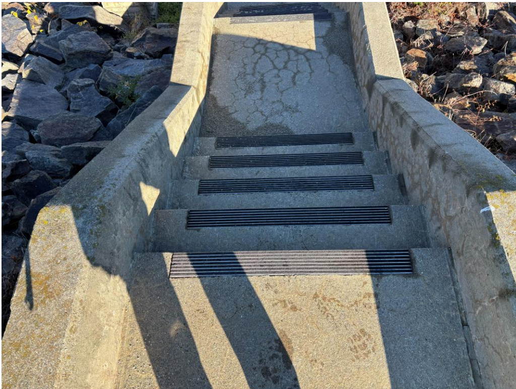
General Condition of Stairs on Reservoir Side
