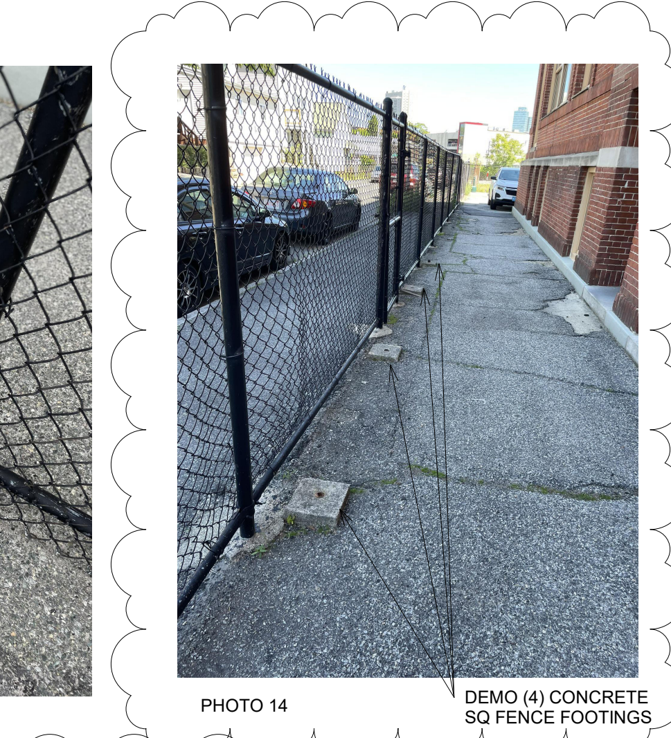
PHOTO 14 DEMO (4) CONCRETE SQ FENCE FOOTINGS
