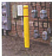
Picture of Bollard cover, use for when Bollards can not be painted.
