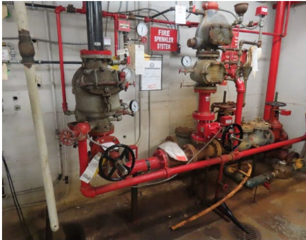
Wet Sprinkler System
