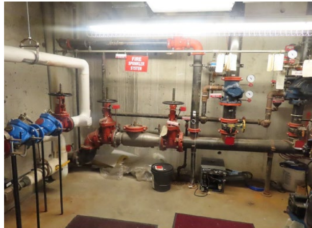
Wet Sprinkler System
