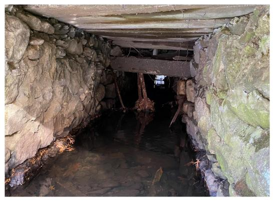
**Photo 3:** Inside of culvert looking upstream with rock and mortar walls and concrete cap.
