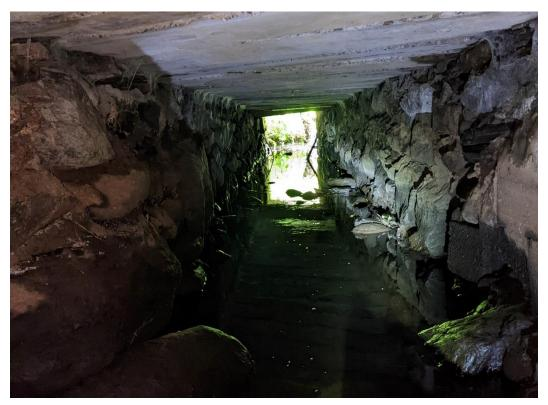
**Photo 4:** Inside of culvert looking downstream with rock and mortar walls and concrete cap.
