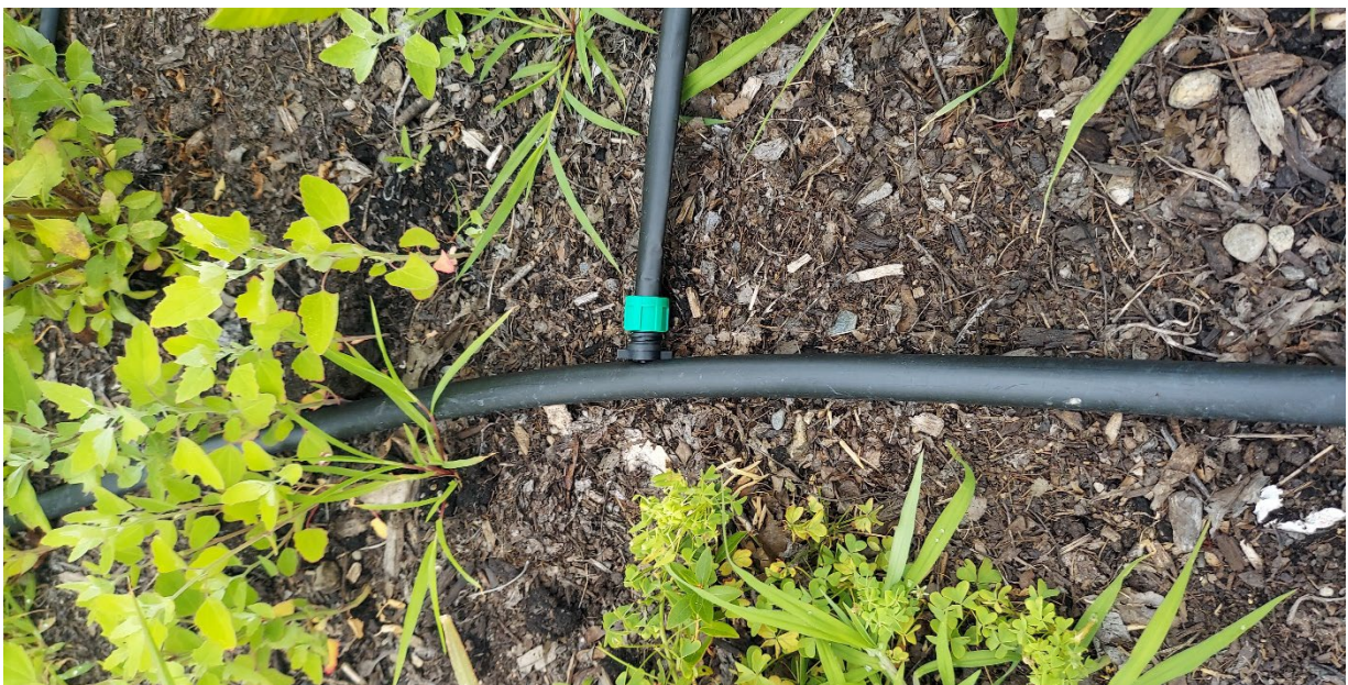
Figure 5: Distribution Line & Drip Connector
