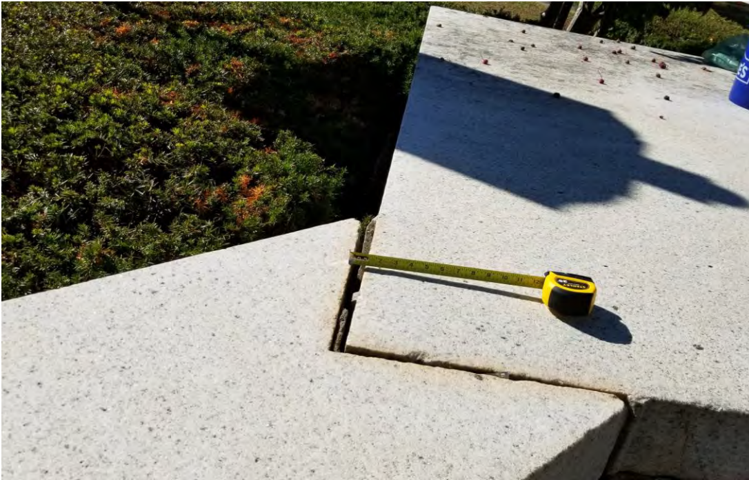
Photo No. 6: Displaced wall stone (knee high wall).
