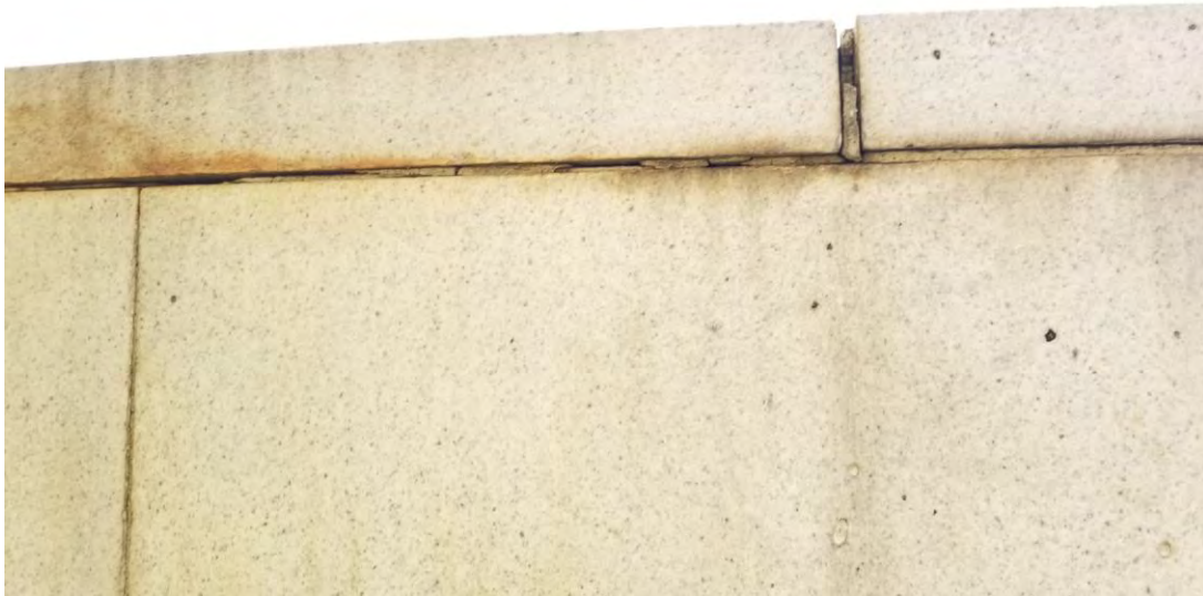
Photo No. 19: Displaced stone (whisper wall).
