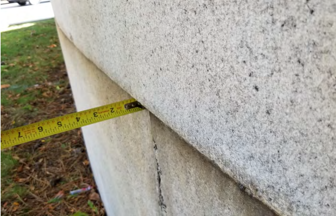
Photo No. 17: Displaced stone (whisper wall).
