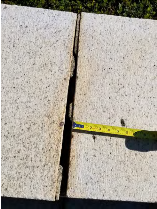
Photo No. 9: Filled and displaced wall stone (knee high wall).
