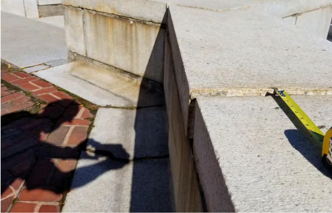
Photo No. 11: Displaced wall stones (knee high wall).
