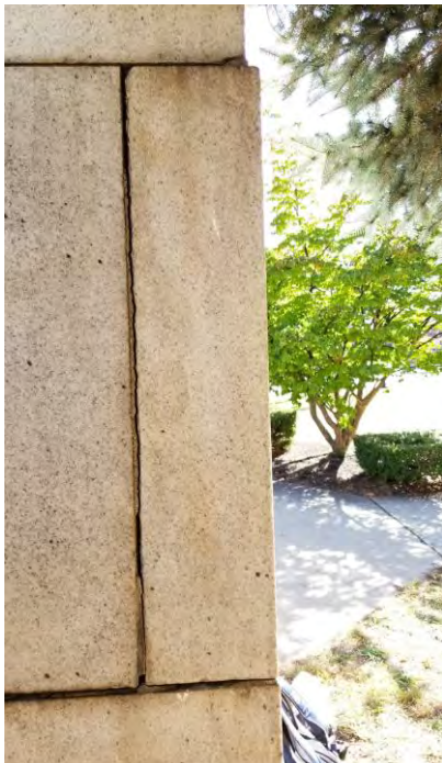
Photo No. 20: Displaced stone (whisper wall).
