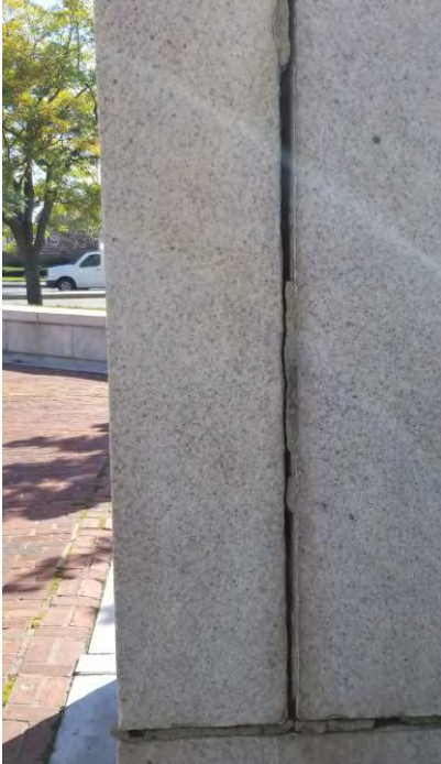
Photo No. 21: Displaced stone (whisper wall).
