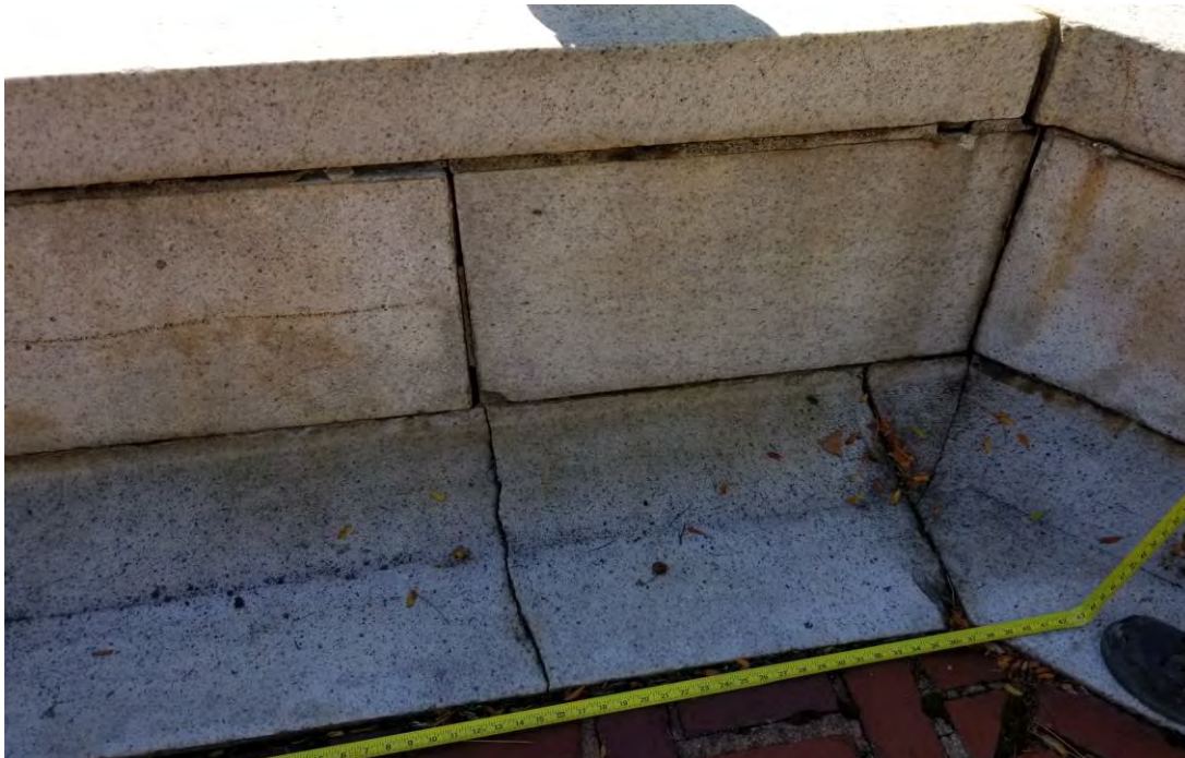
Photo No. 2: Crack in ground stone and displaced wall stones.
