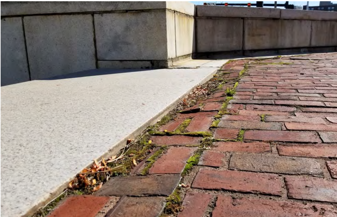
Photo No. 12: Depression in brick pavers at interface with stairs.
