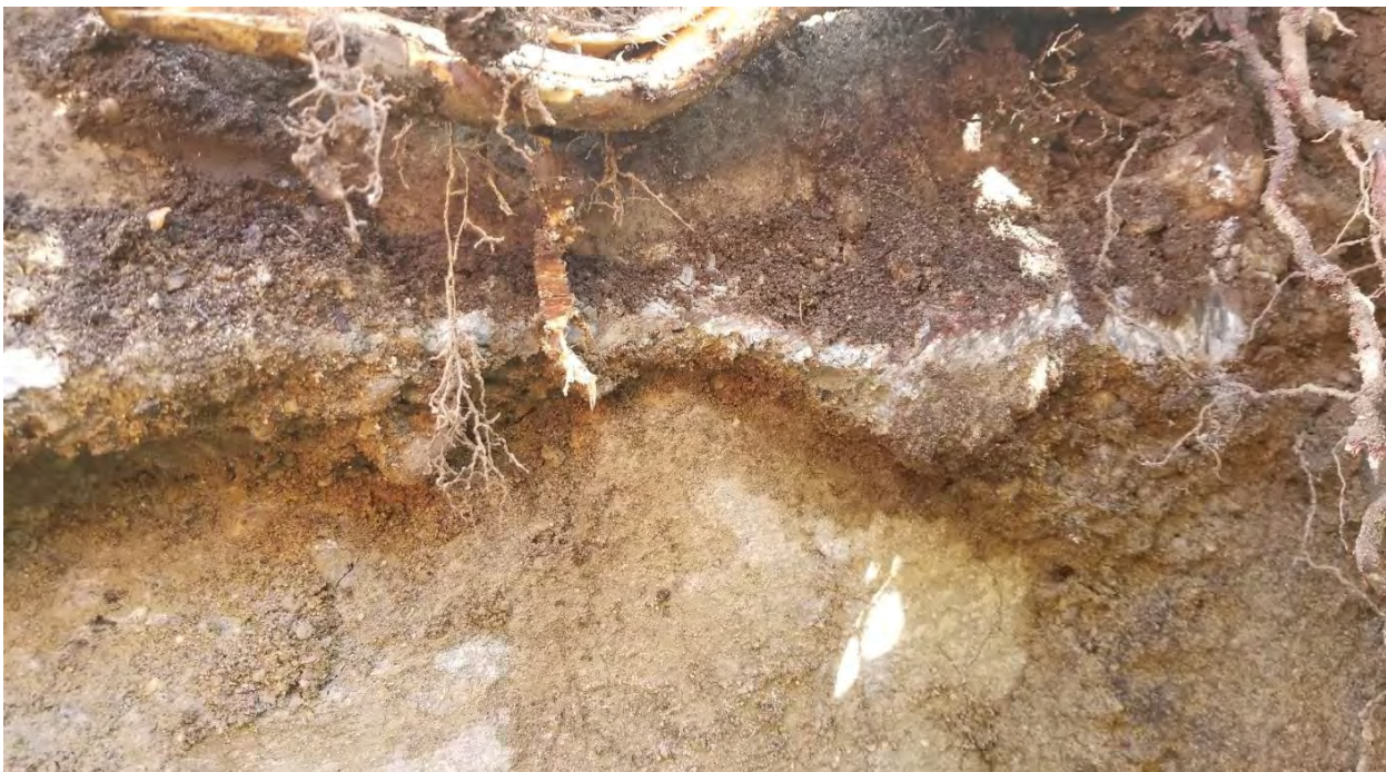
Photo 4 - TP_1 - Seam of soil between foundation and leveling pad
