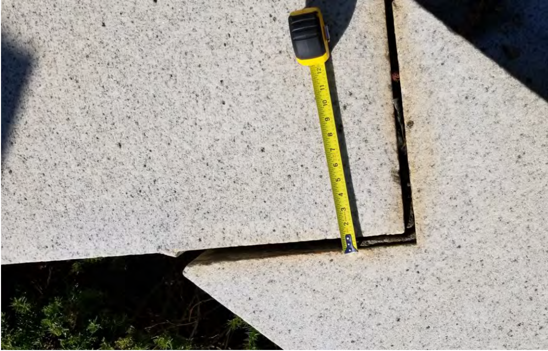
Photo No. 5: Displaced wall stone (knee high wall).
