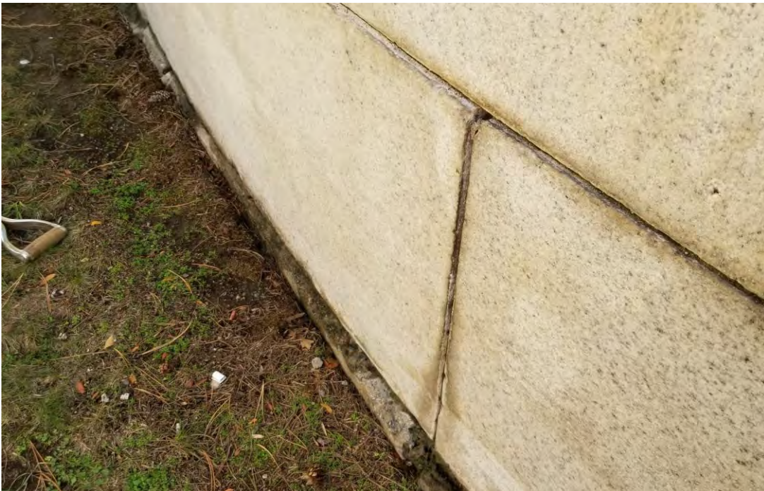
Photo No. 18: Displaced stone (whisper wall).
