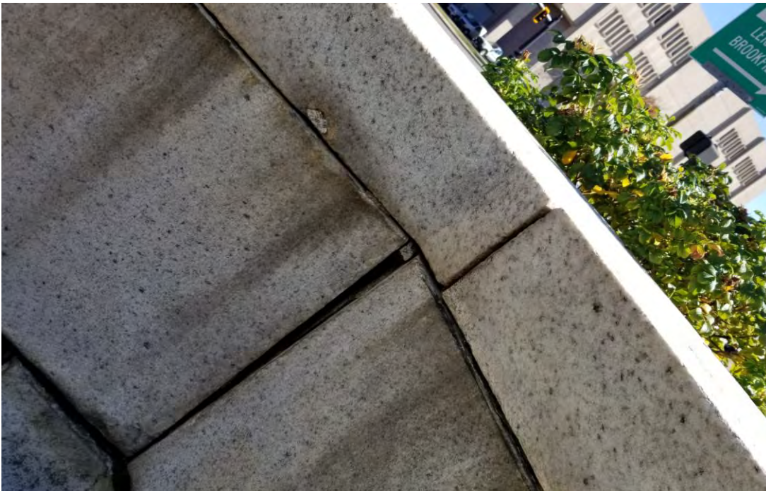
Photo No. 8: Filled wall stones (knee high wall).
