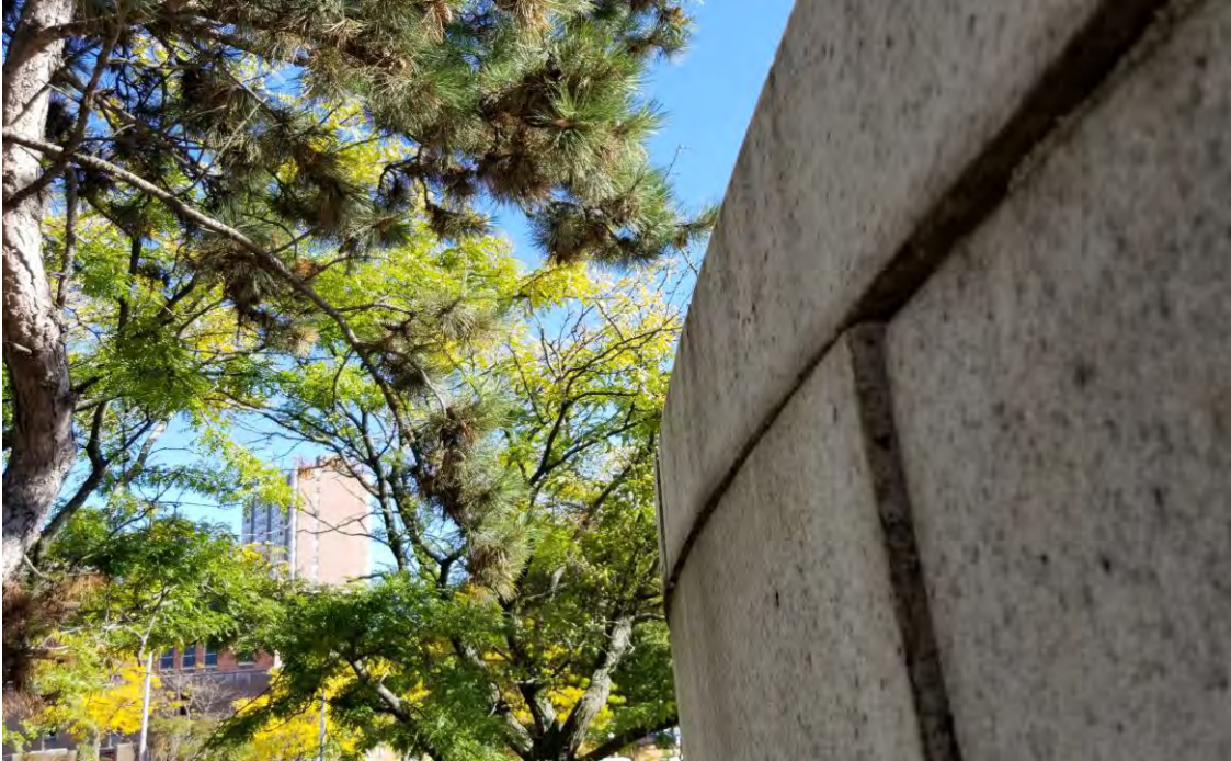
Photo No. 15: Displaced stone (whisper wall).
