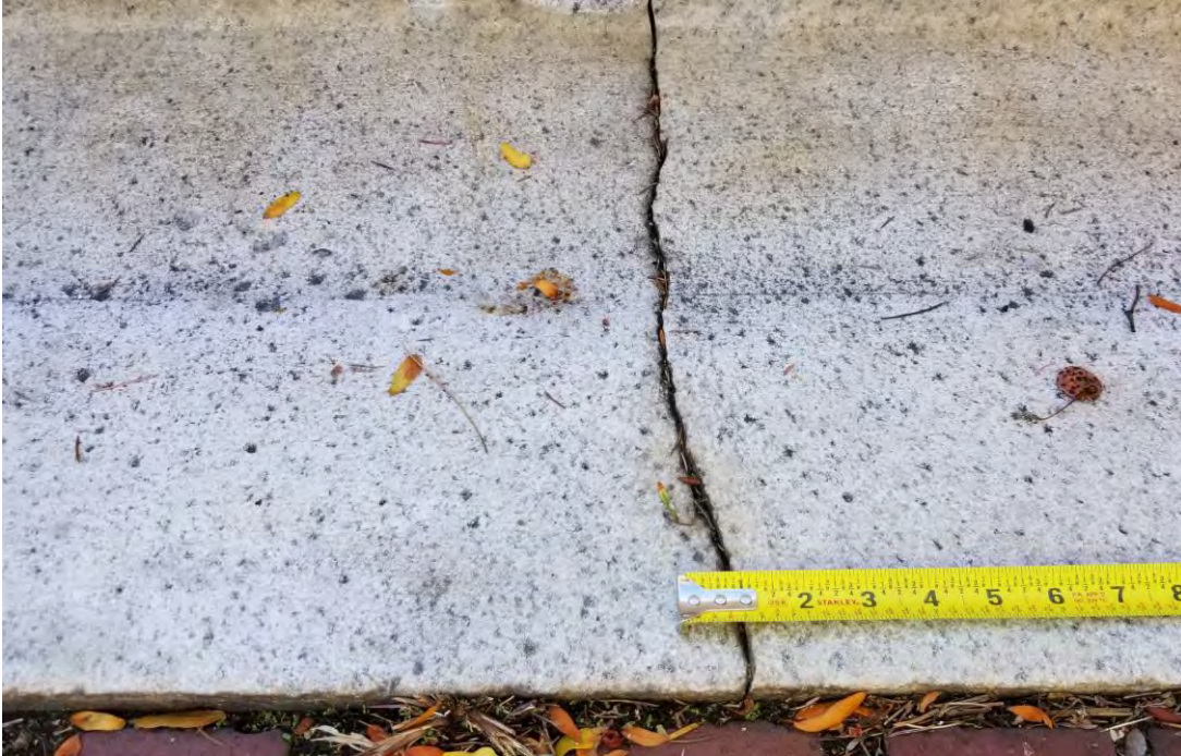
Photo No. 3: Crack in ground stone.
