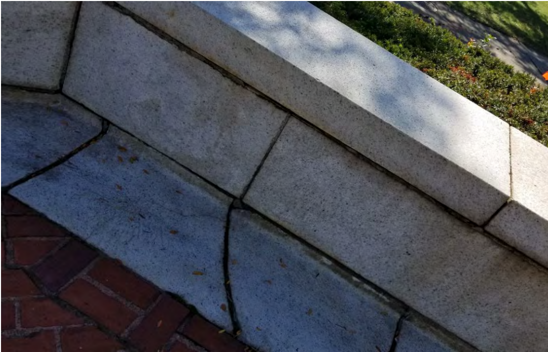
Photo No. 7: Crack in ground stone and displaced wall stones (knee high wall).
