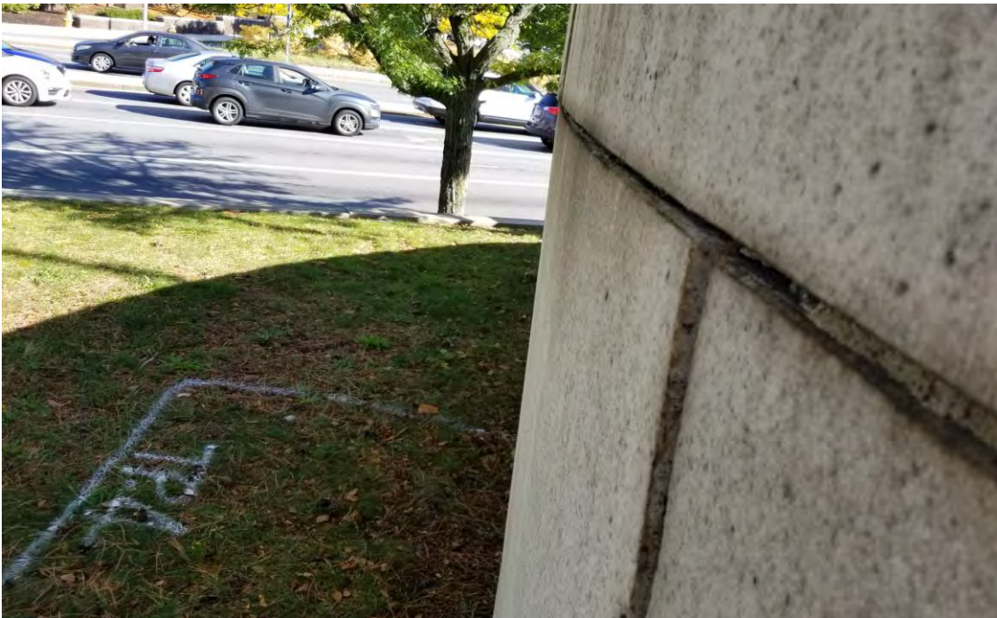
Photo No. 16: Displaced stone (whisper wall).
