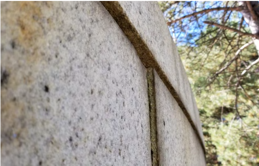
Photo No. 14: Displaced stone (whisper wall).
