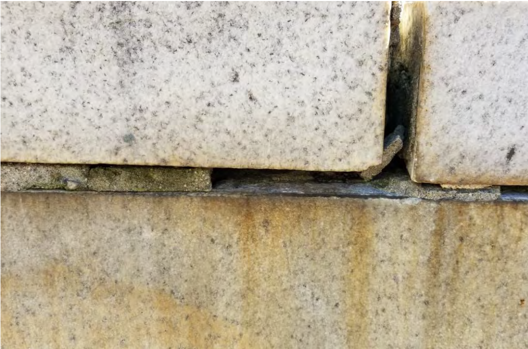
Photo No. 10: Displaced wall stones (knee high wall).
