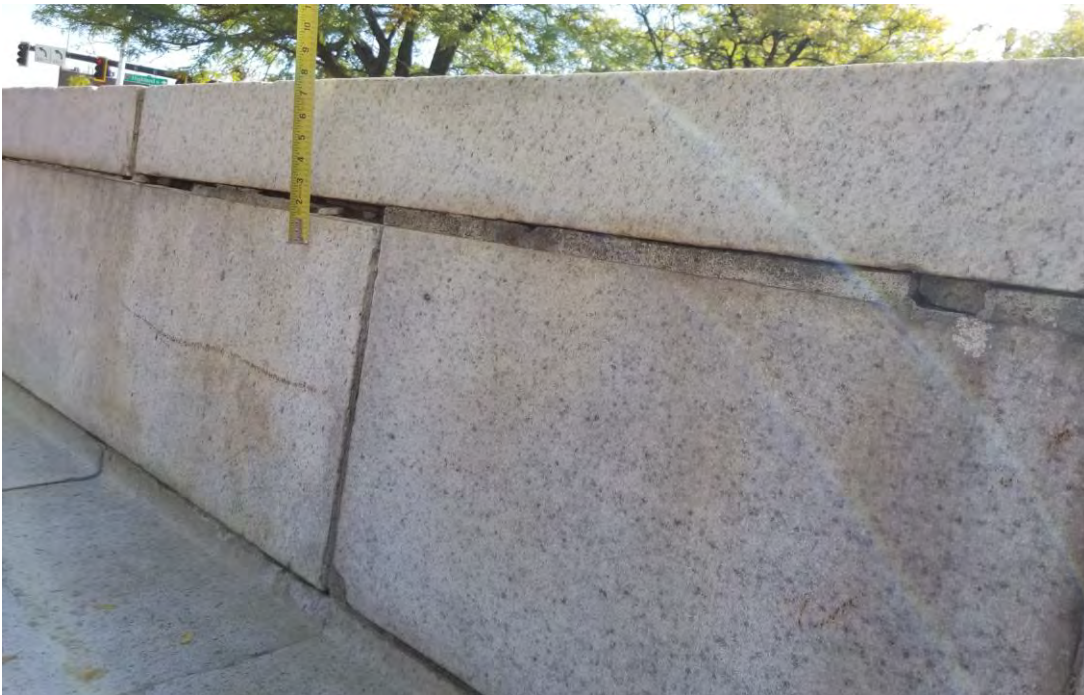
Photo No. 4: Displaced wall stone (knee high wall).
