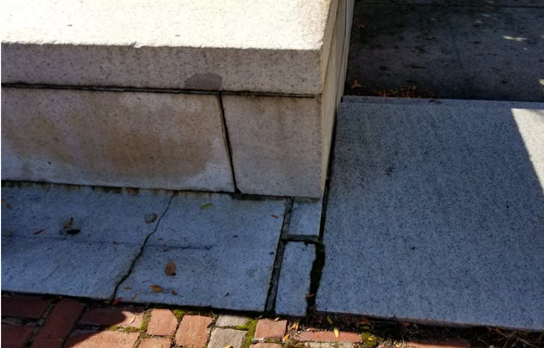
Photo No. 1: Crack in ground stone and displaced wall stones.
