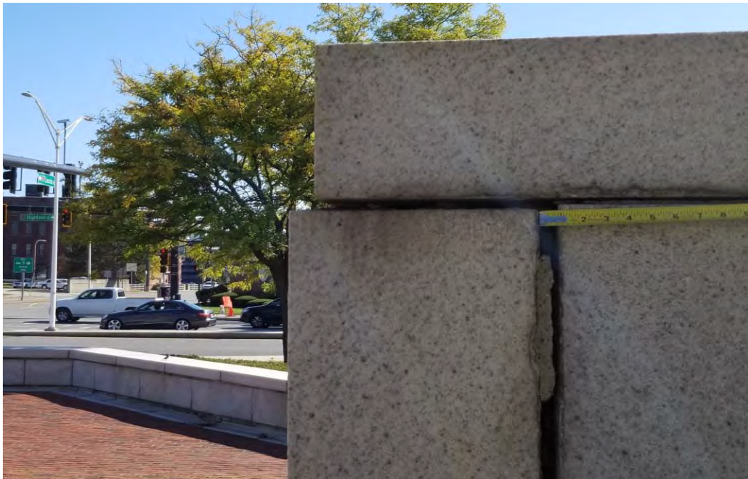
Photo No. 22: Displaced stone (whisper wall).
