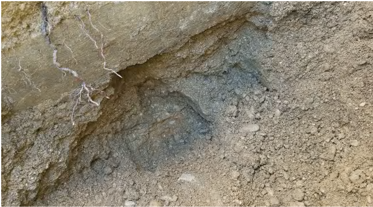
Photo 3 - TP-1 - Existing Fill under foundation
