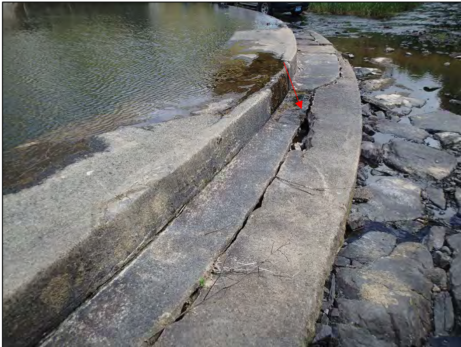
Photo No. 28.: End sill of the spillway with settled cracks and water penetrating the cracks.
