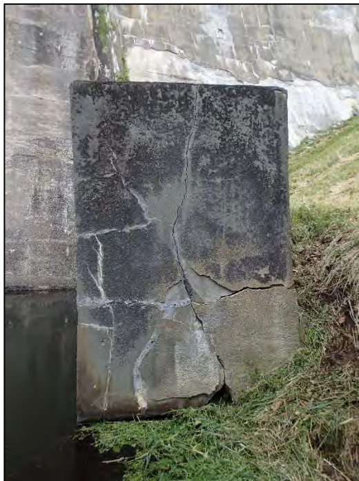
Photo No. 32.: Downstream end of the left training wall. Note cracking and potential misalignment.
