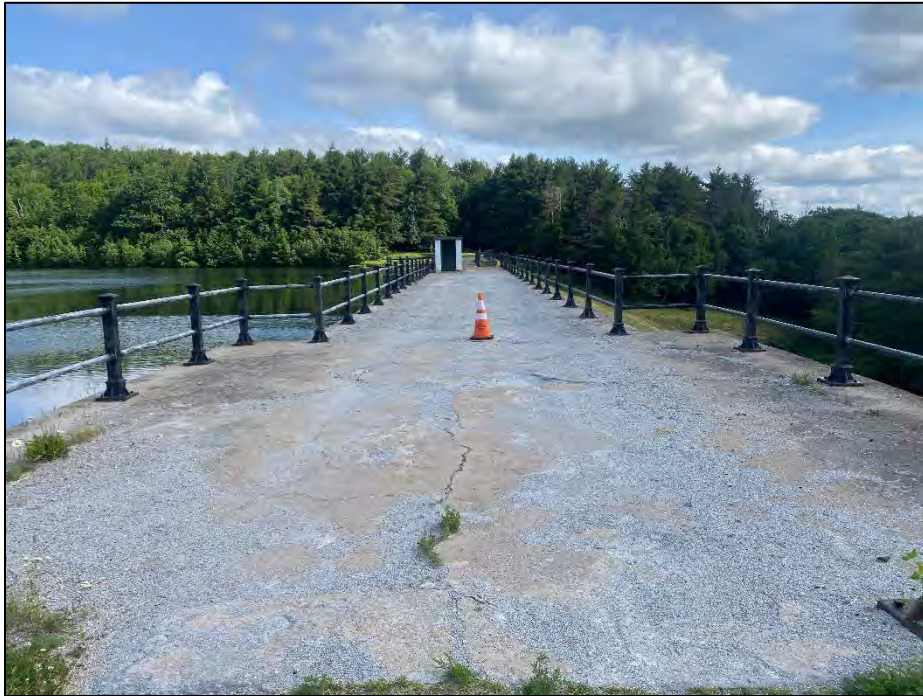
Photo No. 11.: Crest from STA 1+75 looking left. Note deterioration and cracking of the concrete.
