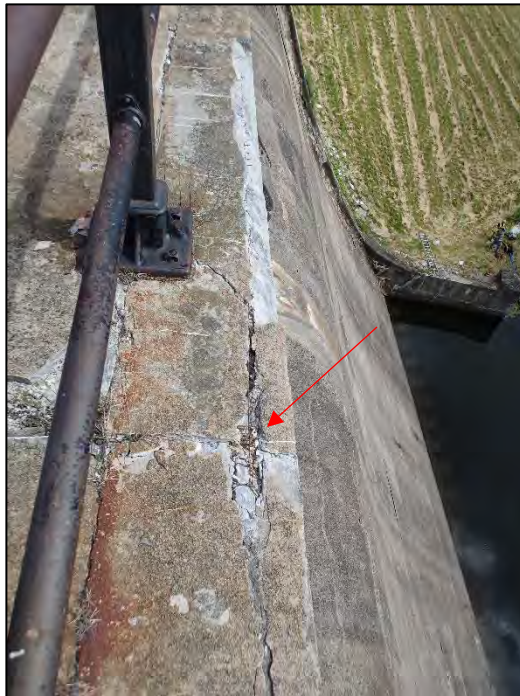
Photo No. 13.: Crack on the downstream edge of the crest. Note missing concrete and exposed steel mesh.
