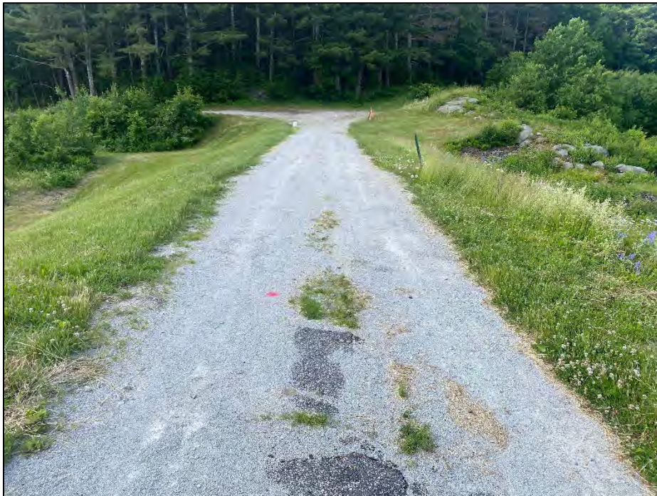
Photo No. 10.: Crest from STA 1+75 looking right. Note deterioration of the asphalt.
