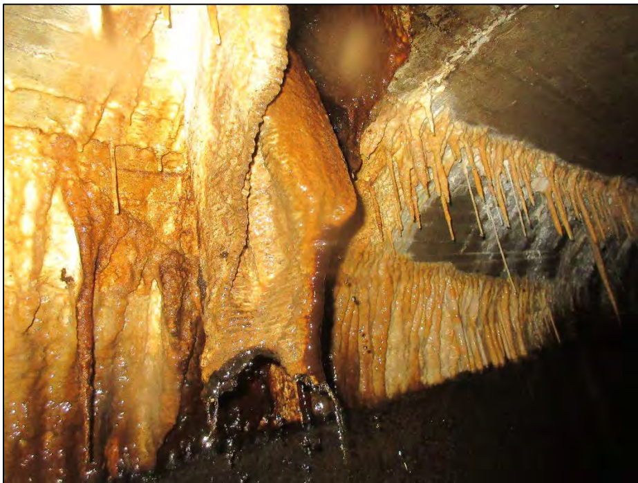
Photo No. 44.: Seepage gallery drain with iron oxide staining, flow, and calcification.
