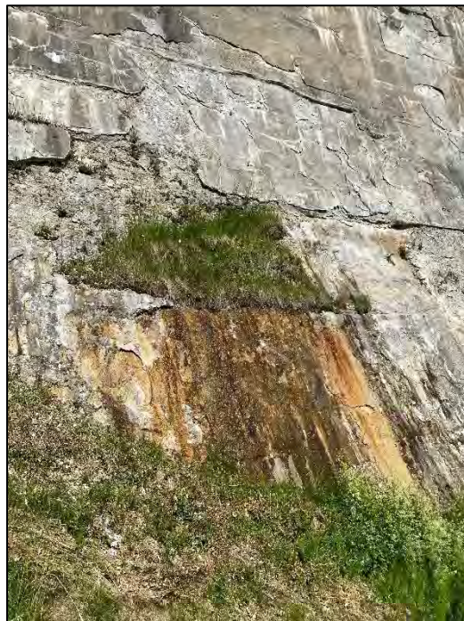
Photo No. 20.: Seepage area approximately 60 feet from the right side of the spillway. Note vegetation developing immediately above the seepage and iron oxide staining.
