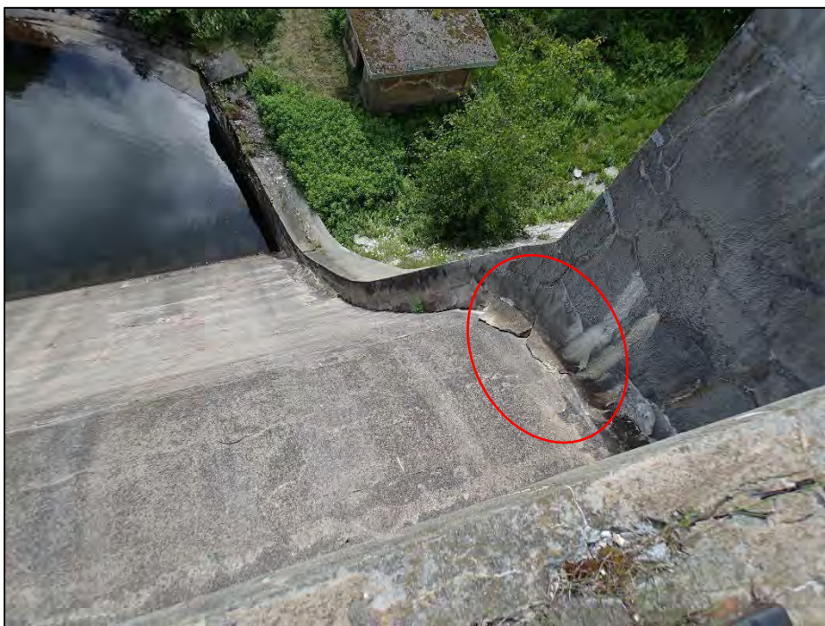
Photo No. 29.: Right training wall and spillway. Note delamination and cracking of concrete at the intersection of the two.
