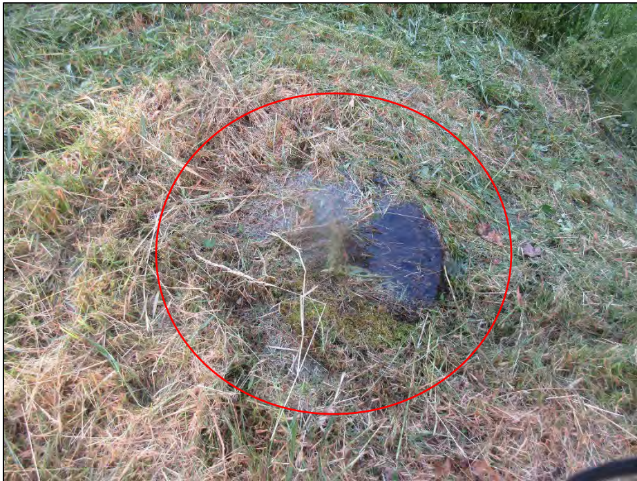
Photo No. 40.: Manhole to the seepage gallery in the downstream area to the left of the spillway. Note the seepage gallery is filled with water and leaking from the manhole.
