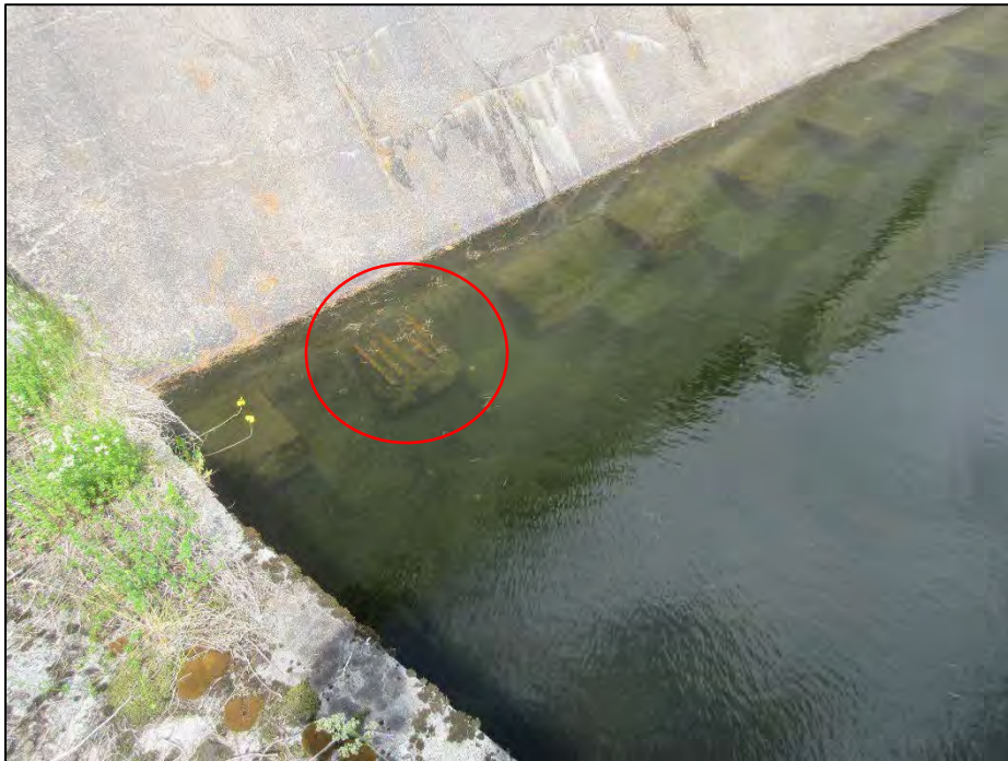
Photo No. 34.: Baffle block with exposed rebar in the top row of the baffle blocks.
