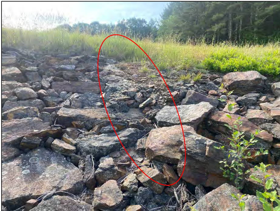
Photo No. 2.: Area of erosion and soil movement at the bend of the upstream riprap near STA 0+90.
