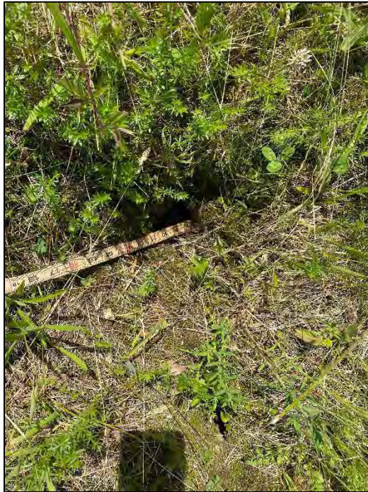
Photo No. 17.: Typical animal burrow observed on the downstream slope.
