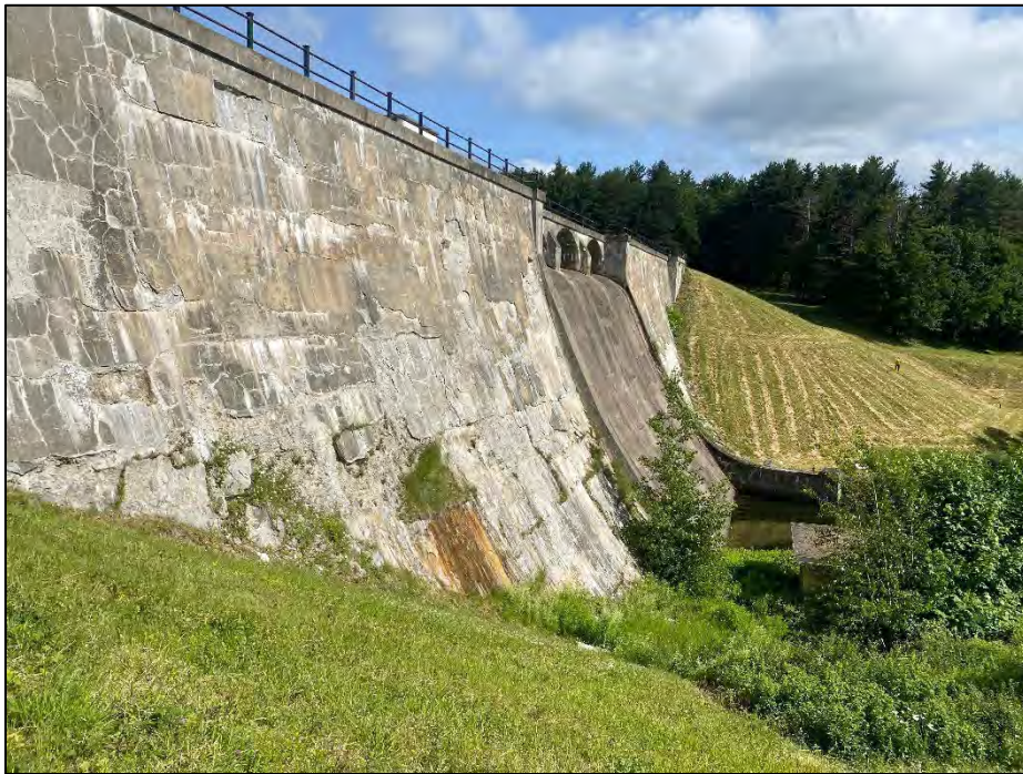
Photo No. 19.: Downstream face from the right end looking left. Note delamination, spalls, and vegetation developing on the wall.
