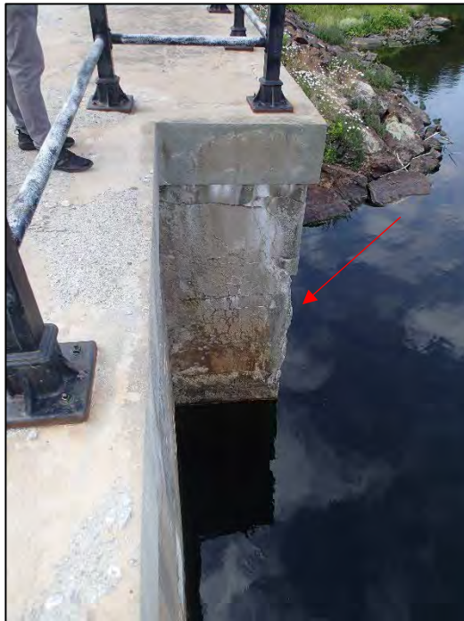
Photo No. 5.: Spalled and cracked concrete on the upstream face near STA 2+00.
