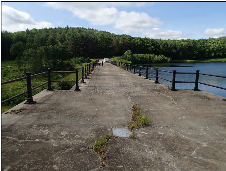
Photo No. 14.: Crest from STA 5+50 looking right. Note cracking and developing vegetation within cracks.
