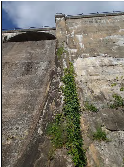
Photo No. 31.: Left training wall of the spillway. Note developing vegetation and cracking.
