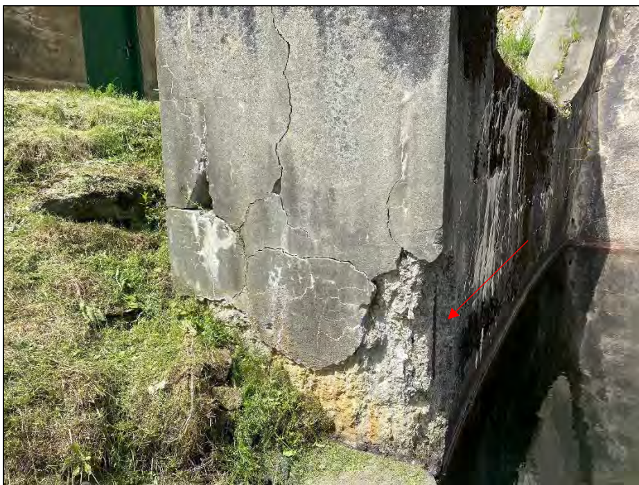
Photo No. 30.: End of the right training wall with exposed rebar and delamination.
