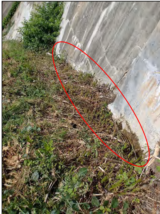
Photo No. 22.: Seepage where the downstream face meets the embankment slope near STA 5+15.
