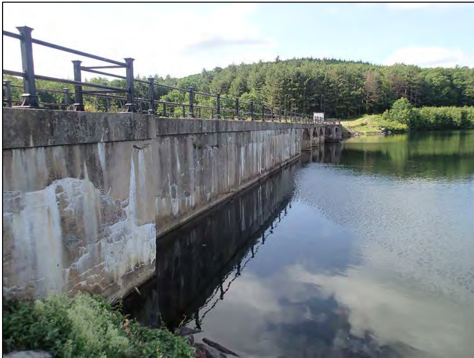
Photo No. 6.: Upstream face from near STA 5+50 looking right. Note cracking and efflorescent staining throughout.
