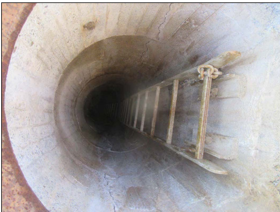
Photo No. 41.: Interior of the access to the gatehouse from the manhole on the crest near STA 2+05.
