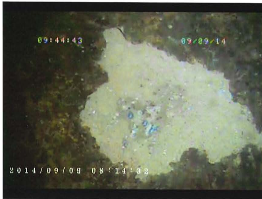
Photograph 5. Typical Concrete Condition with 1/8" to 1/4" Soft Concrete (Station 1 + 15 Shown)
