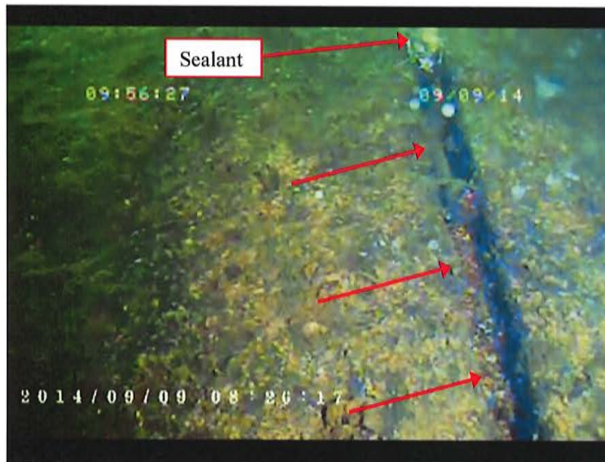
Photograph 4. Typical Open Construction Joint (Station 1 + 28 Shown. Note Sealant Intact at Top)
