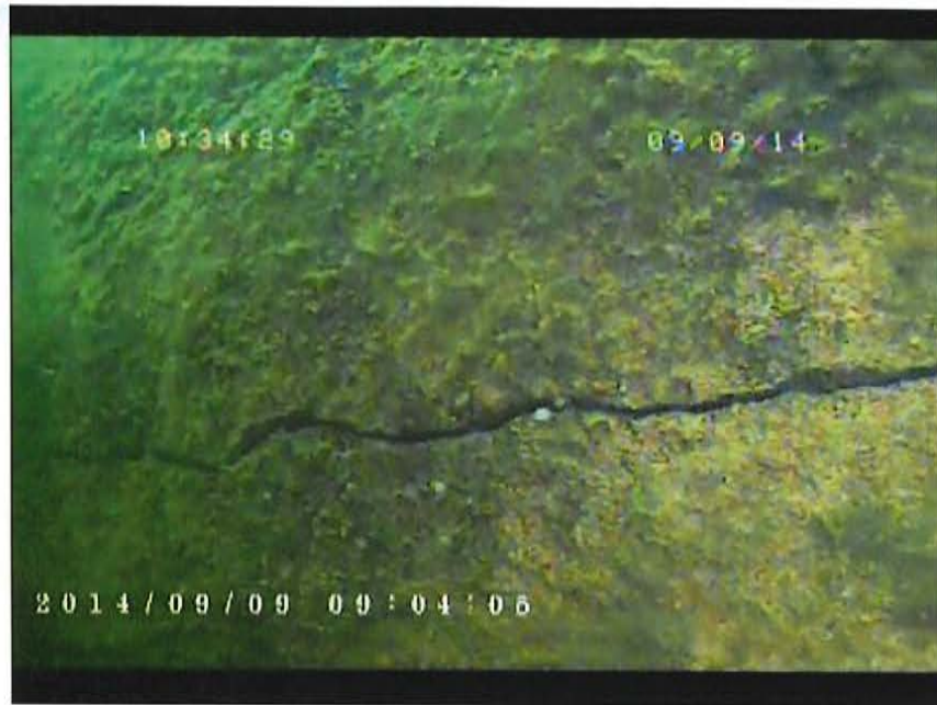
Photograph 3. Typical Horizontal Crack (Station 1 + 80 shown).
