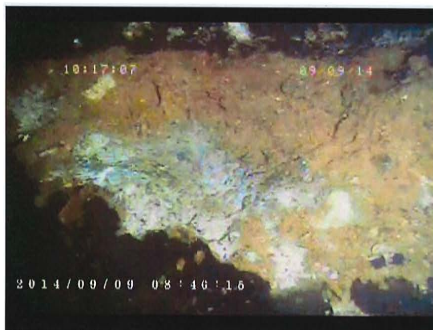
Photograph 6. Concrete Degradation With 2-3" of Soft Concrete (Station 1 + 50 shown).
