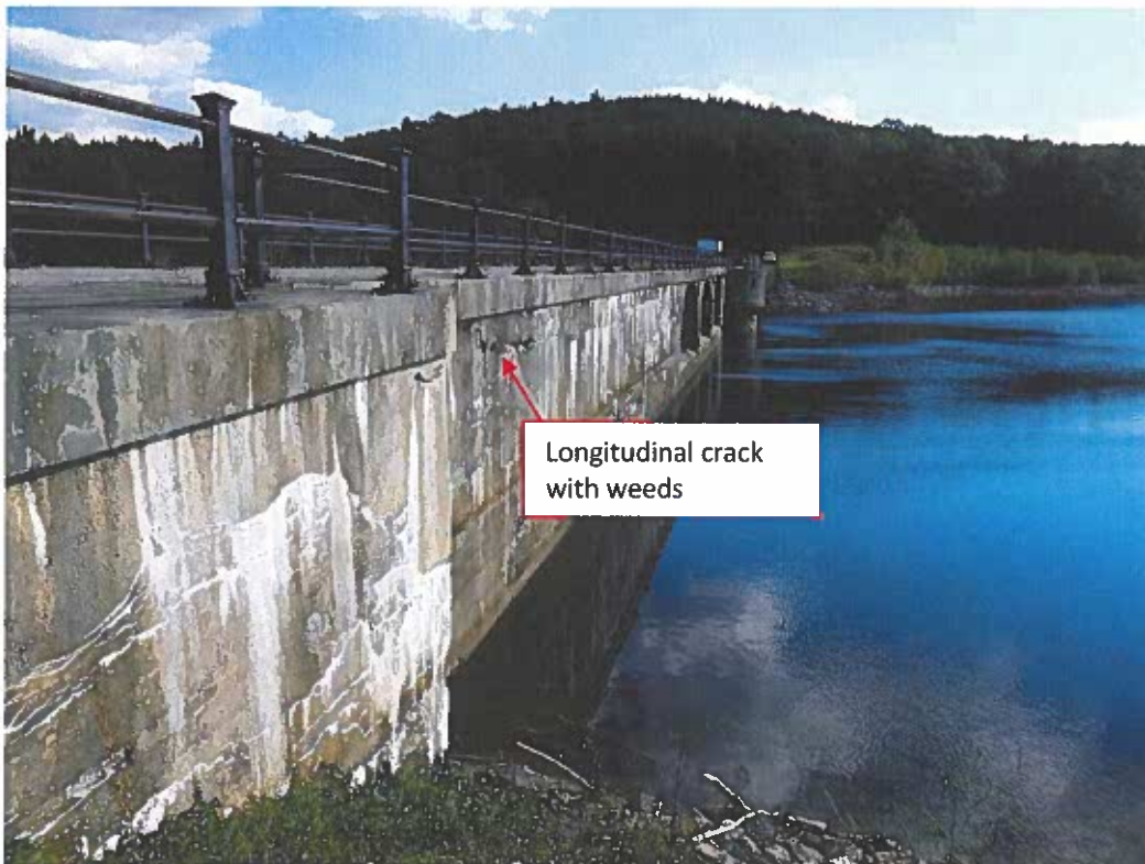
Photo No. 18: Cracks and efflorescence on upstream face of dam. Note that some weeds are growing in the cracks.
