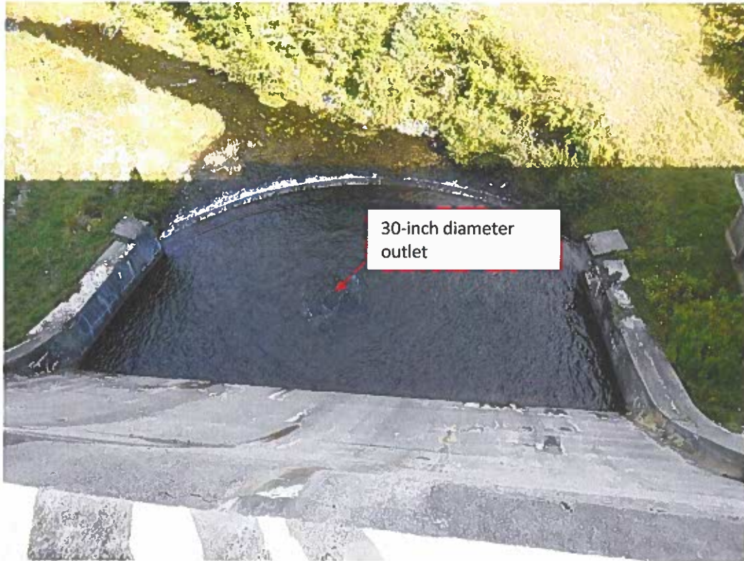
Photo No. 11: Overview of stilling basin looking downstream from the crest. Note variation in elevation of the top of the downstream basin overflow weir. Also note trees along channel.
