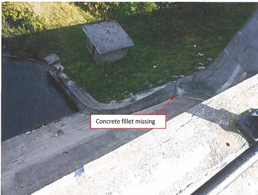
Photo No. 8: Overview of right downstream spillway training wall. Note part of concrete fillet is missing and cracks and efflorescence are present.
