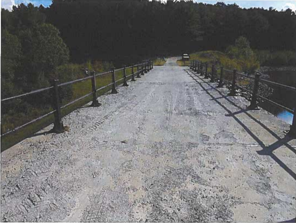
Photo No. 21: Concrete spalled and cracked on right crest (looking towards right abutment).
