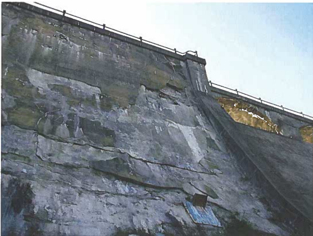
Photo No. 24: A large piece of shotcrete spalled next to the right training wall on the right downstream face. Note weeds growing in the cracks.
