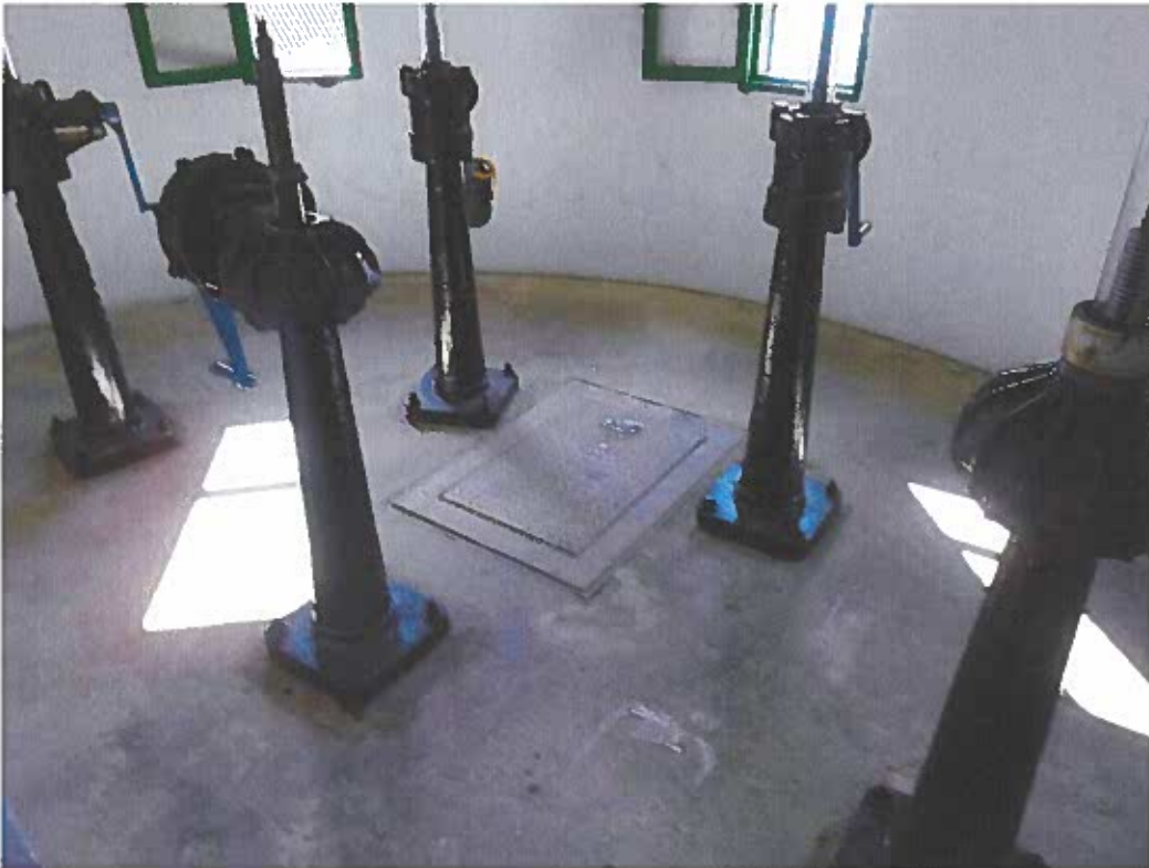
Photo No. 13: Overview of upper gatehouse interior and gate operators – mudgate, 24" x 26" sluice gate low-level outlet, 3 different level gates at reservoir.
