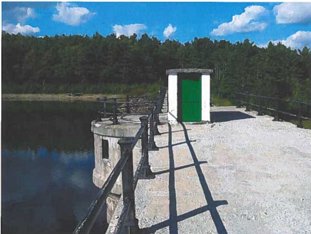
Photo No. 12: Overview of upper gatehouse exterior. Note cracking, spalling, and puddling along concrete deck.
