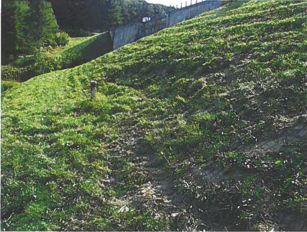
Photo No. 37: Tractor ruts and bare spots on left embankment downstream slope from mowing. Eroded zone remnant from monitoring well installation.
