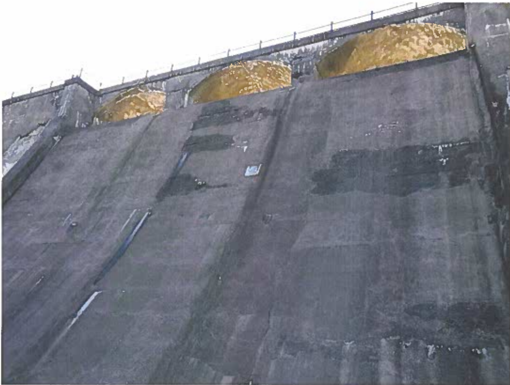
Photo No. 22: Cracks/spalling and efflorescence on the spillway surface (view from downstream).
