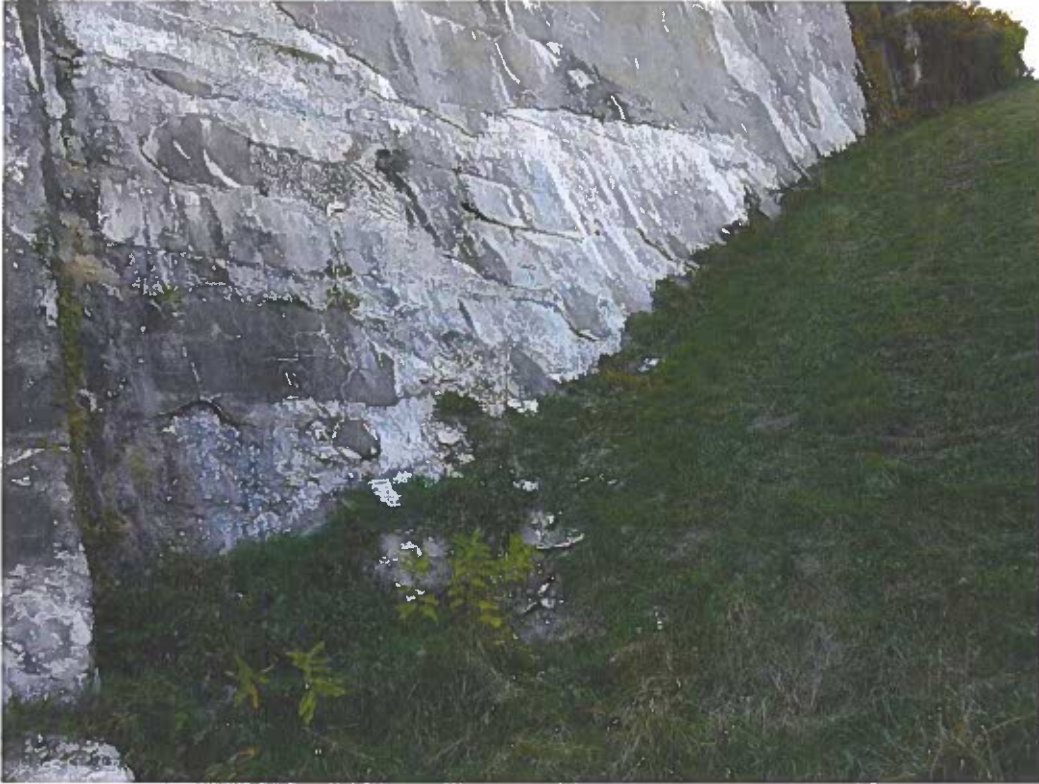
Photo No. 25: Spalling of shotcrete left of the spillway (downstream face). Note calcium deposits forming to the left of the left training wall.
