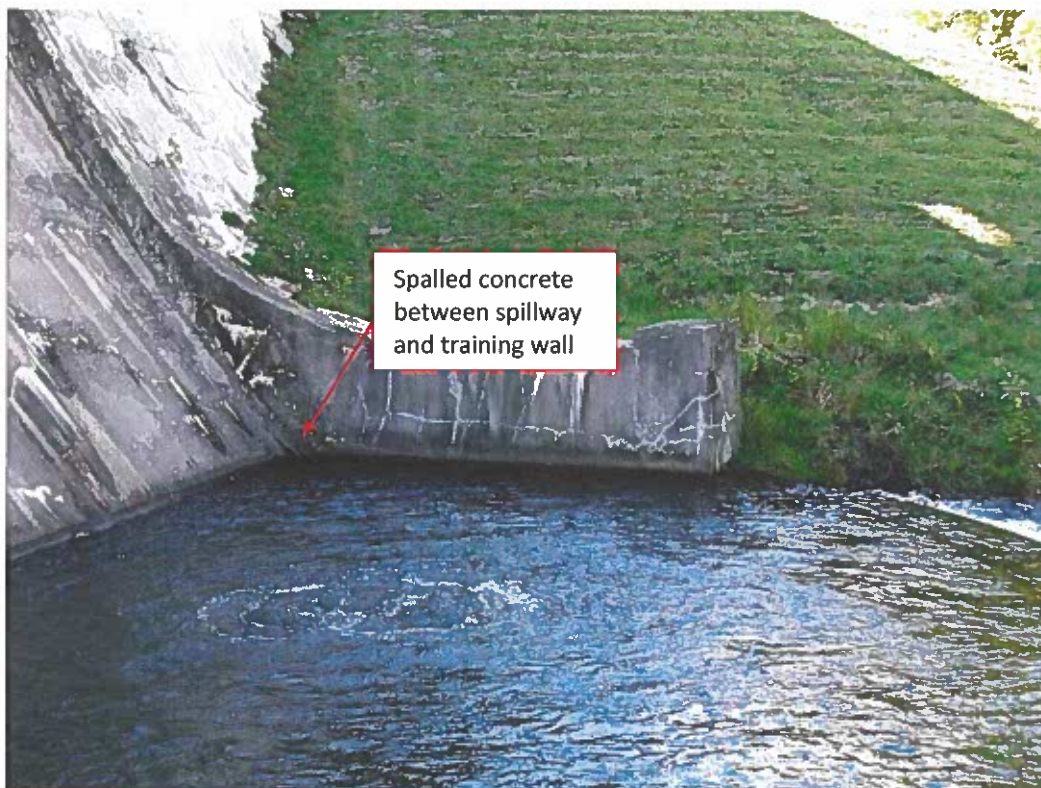
Photo No. 36: Concrete spalled between spillway and training wall at stilling basin. Cracking, spalling, and efflorescence on left training wall.
