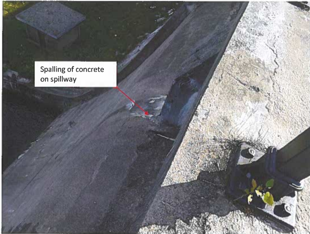
Photo No. 23: Spalling on the spillway surface (view from the crest).
