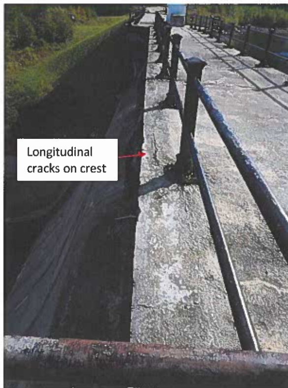
Photo No. 38: Longitudinal cracks along railing. Spalling, cracking, and efflorescence on concrete arch bridge over spillway. Weeds growing in cracks.
