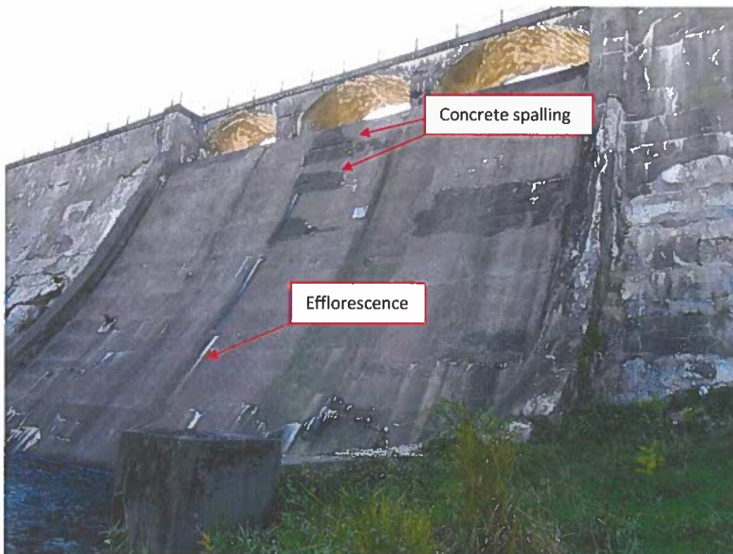
Photo No. 10: Overview of spillway from downstream. Note spalled sections of concrete and efflorescence on spillway weir.
