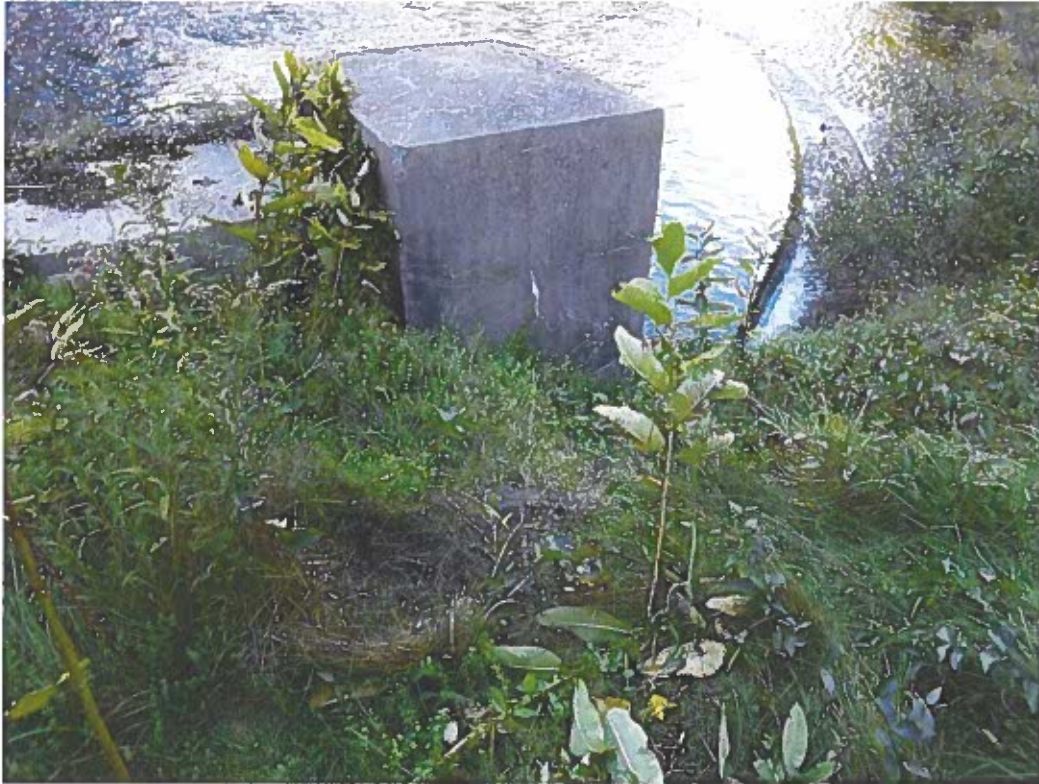
Photo No. 35: Manhole at the right downstream toe of the dam.
