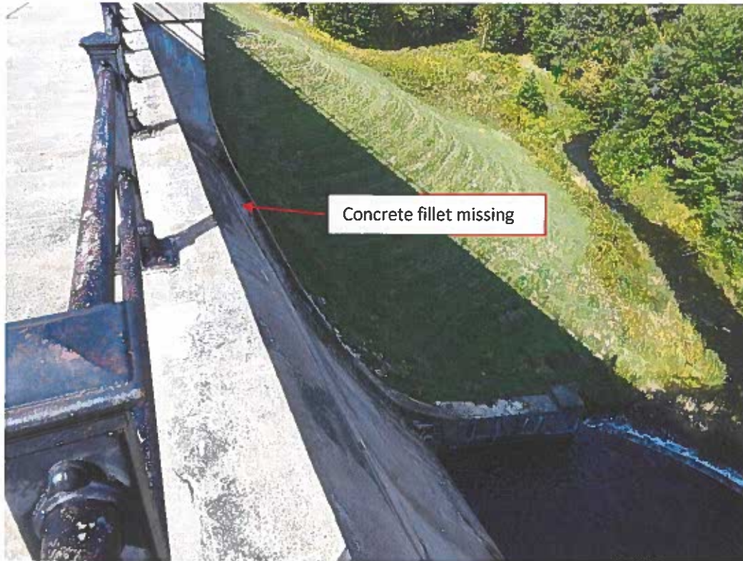
Photo No. 9: Overview of left downstream spillway training wall. Note part of concrete fillet is missing and cracking and efflorescence are present on the wall.
