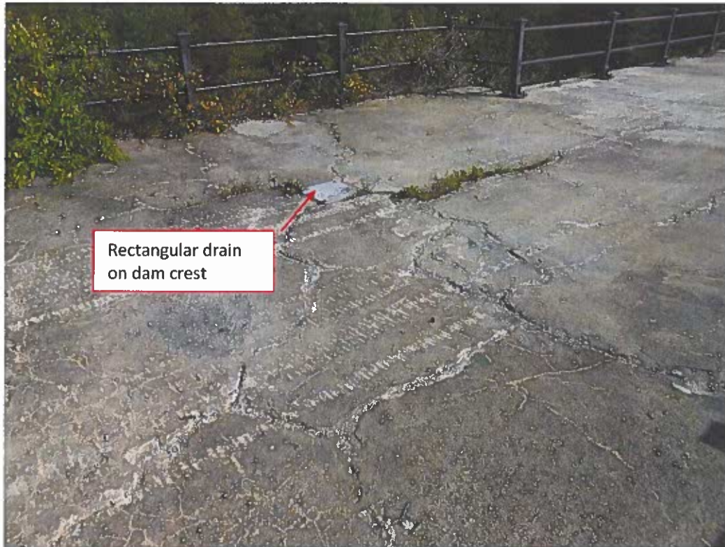
Photo No. 19: Cracks on crest near left embankment. Note minor weeds and moss growing in the cracks. Rectangular drain leads directly to left-most inspection gallery drainage well.
