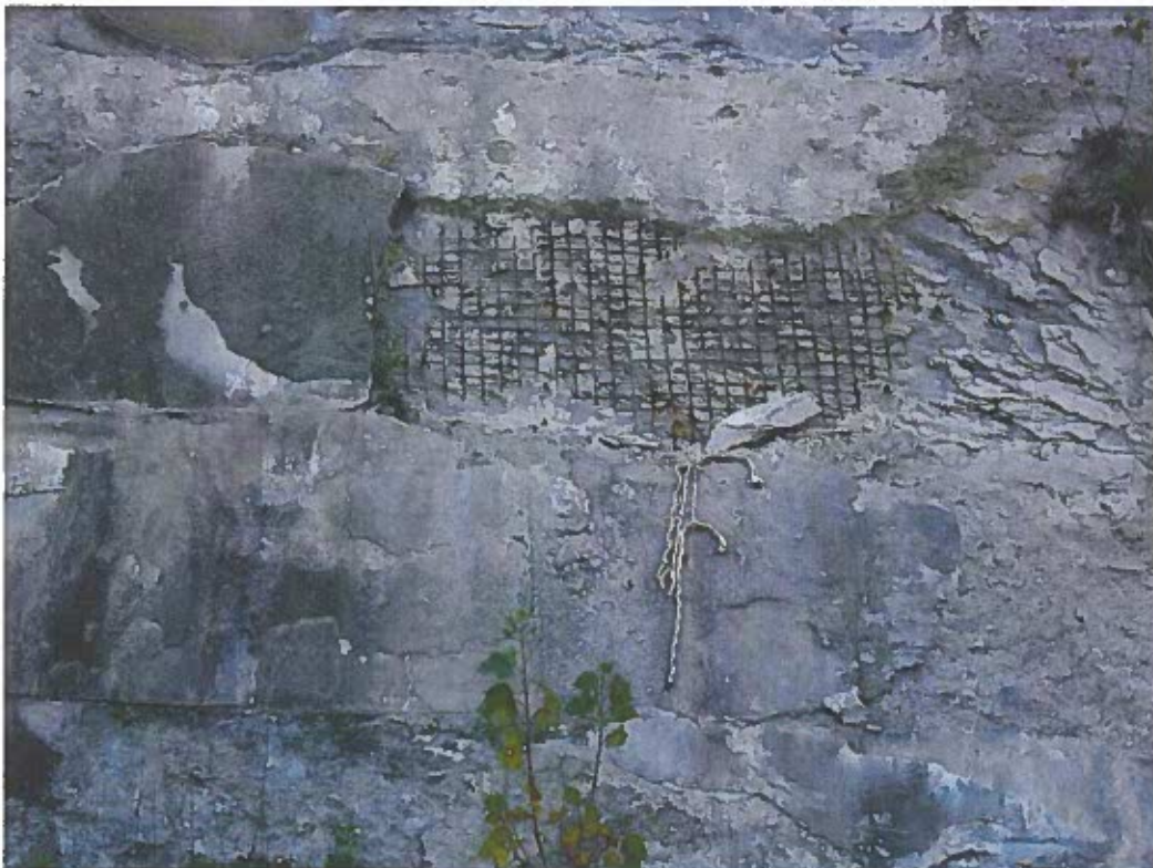
Photo No. 26: A large section of shotcrete spalled exposing wire mesh on the downstream face of dam next to left training wall.
