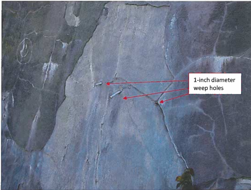
Photo No. 31: PVC weep holes on the downstream face of the dam to left of spillway. Weep holes were installed when dam face was sandblasted and shotcrete-covered in 1981 to 1982.
