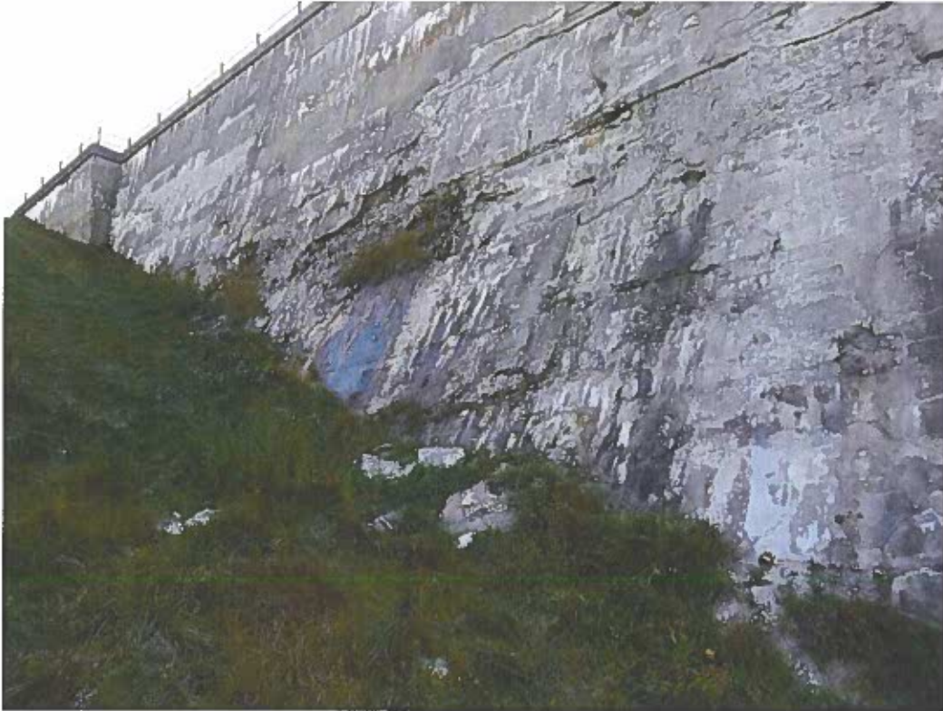
Photo No. 29: Efflorescence, cracking, spalling and weeds growing in the cracks on the downstream face of the dam to right of spillway.
