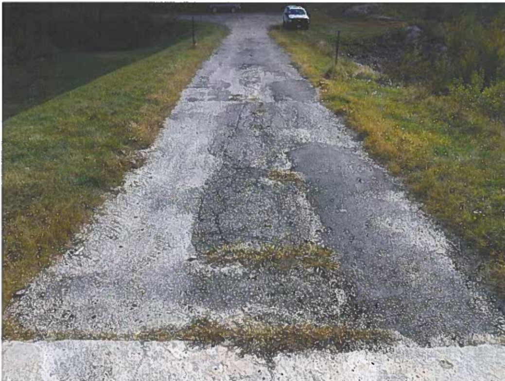
Photo No. 20: Pavement eroded, rutted, and cracked on right crest (looking towards right abutment).
