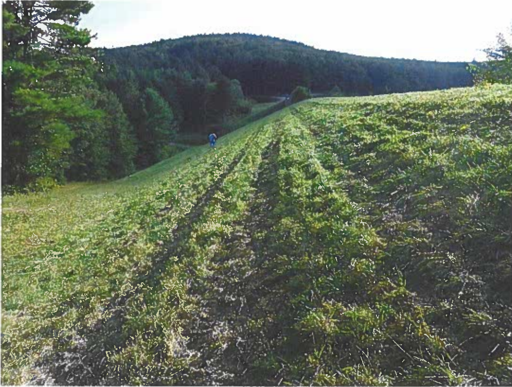
Photo No. 7: Overview of downstream slope from left abutment. Note ruts in grass due to mowing equipment.
