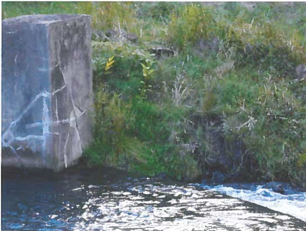
Photo No. 34: Downstream manhole access to drainage gallery. Note that water draining from the top of the drainage gallery manhole is causing erosion of the downstream bank.
