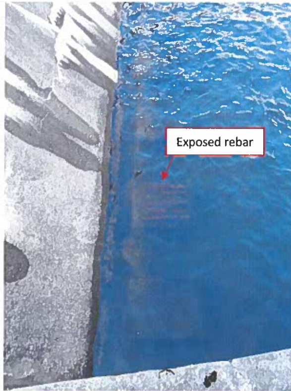
Photo No. 39: Exposed rebar on baffle blocks in stilling basin.
