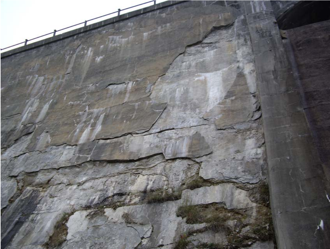
Photo No. 21: A large piece of shotcrete spalled next to the right training wall. Note weeds growing in the cracks.
