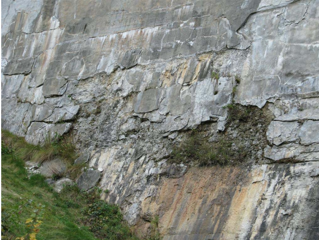
Photo No. 27: Efflorescence, cracking, spalling and weeds growing in the cracks on the downstream face of the dam to right of spillway.
