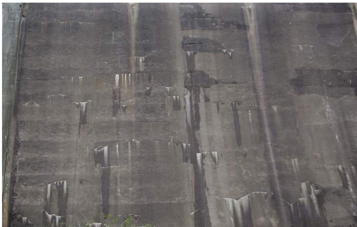
Photo No. 20: Cracks and efflorescence on the spillway surface (View from downstream).
