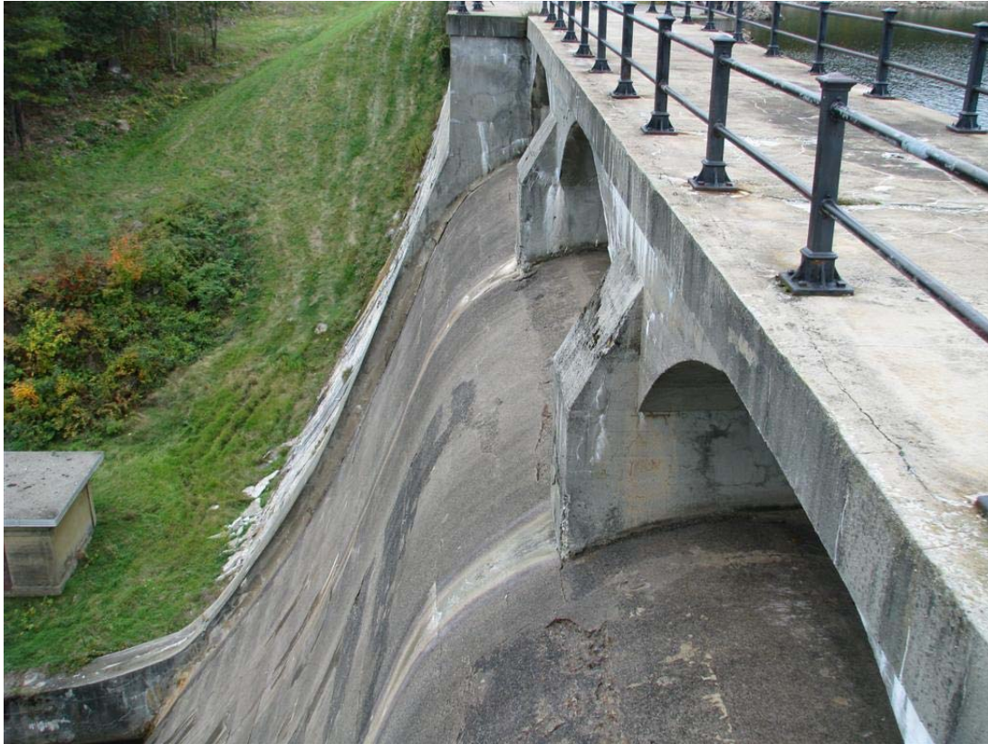
Photo No. 35: Longitudinal cracks along railing. Spalling, cracking, and efflorescence on concrete arch bridge over spillway. Weeds growing in cracks.
