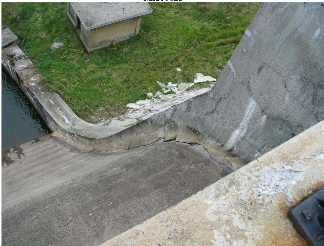
Photo No. 9: Overview of right downstream spillway training wall. Note part of concrete fillet is missing.
