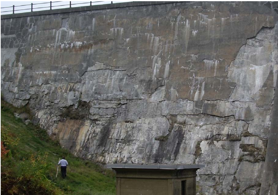
Photo No. 24: Large areas of spalling on downstream face of the dam to the right of the spillway.
