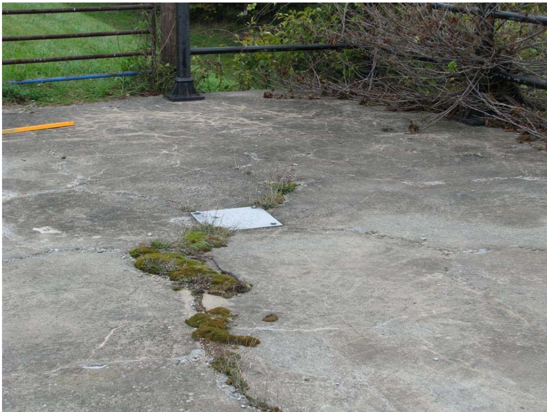
Photo No.18: Crack on crest near left embankment. Note weeds and moss growing in the crack.
