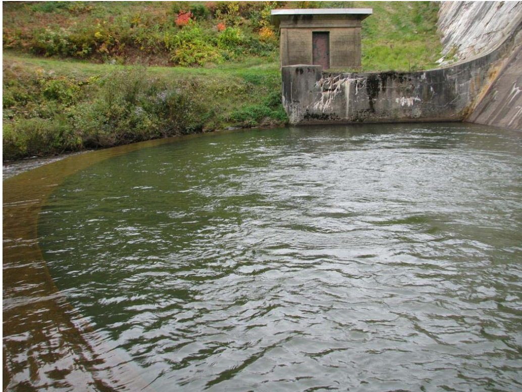
Photo No. 32: Cracking, spalling, and efflorescence on right training wall at stilling basin.
