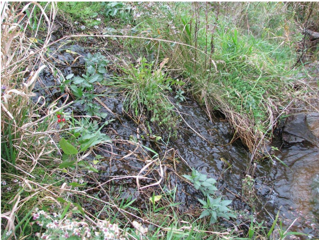
Photo No. 30: Outlet from drainage gallery clogged and overgrown. Water overflowing from manhole cover above.
