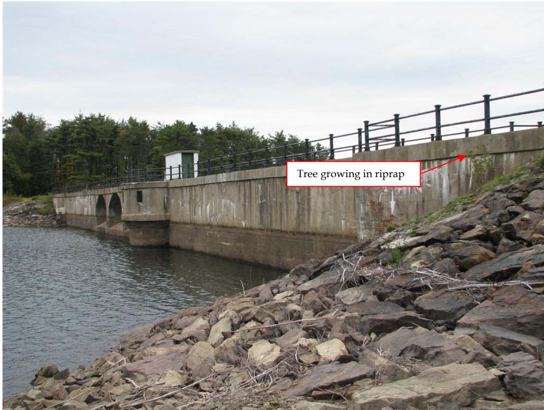
Photo No. 1: Overview of dam and upstream face from right abutment. Note brush on riprap near concrete dam contact.
