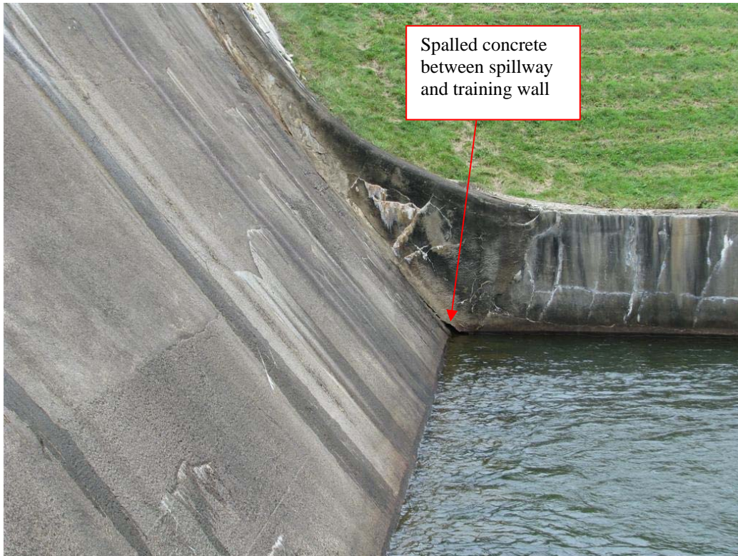
Photo No. 31: Concrete spalled between spillway and training wall at stilling basin. Cracking, spalling, and efflorescence on left training wall.
