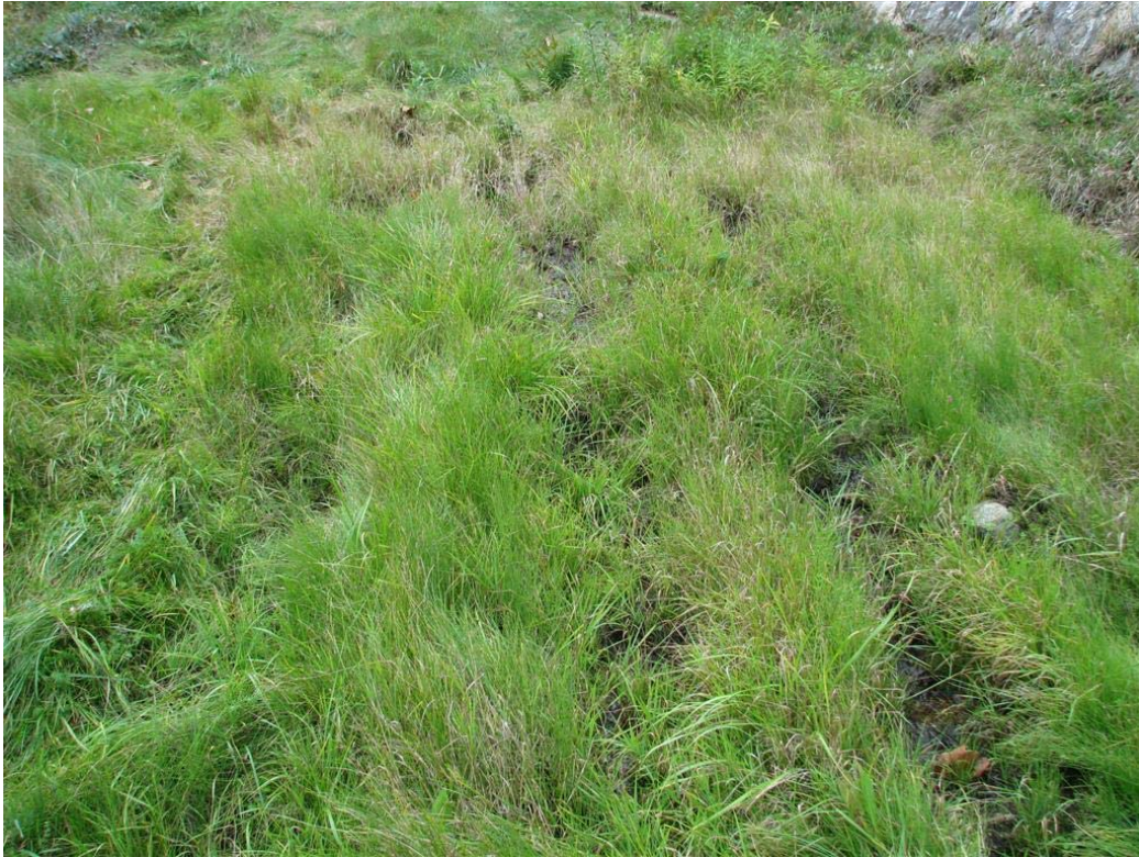
Photo No. 33: Wet area on right slope between dam face and outlet gatehouse.
