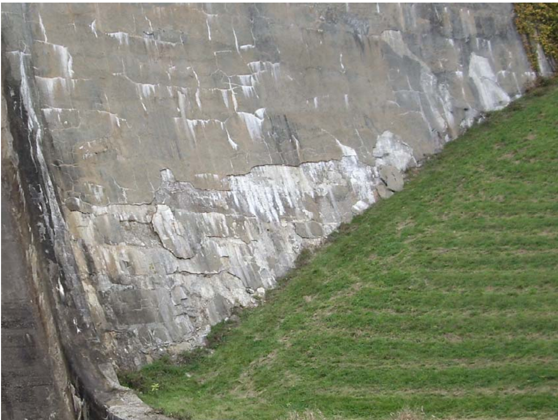
Photo No. 22: Spalling of shotcrete left of the spillway (downstream face).
