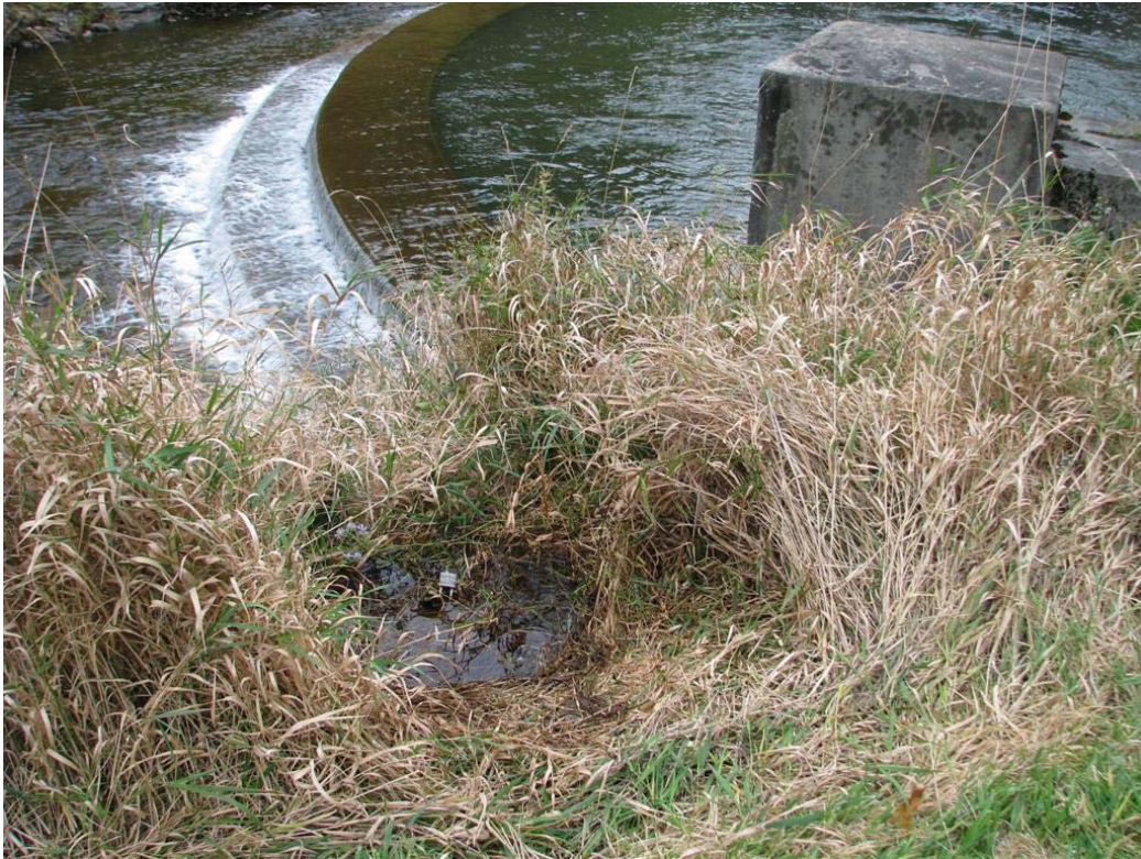
Photo No. 29: Entrance to the gallery under the dam. Note the manhole cover is locked and water is flowing out of holes in cover.
