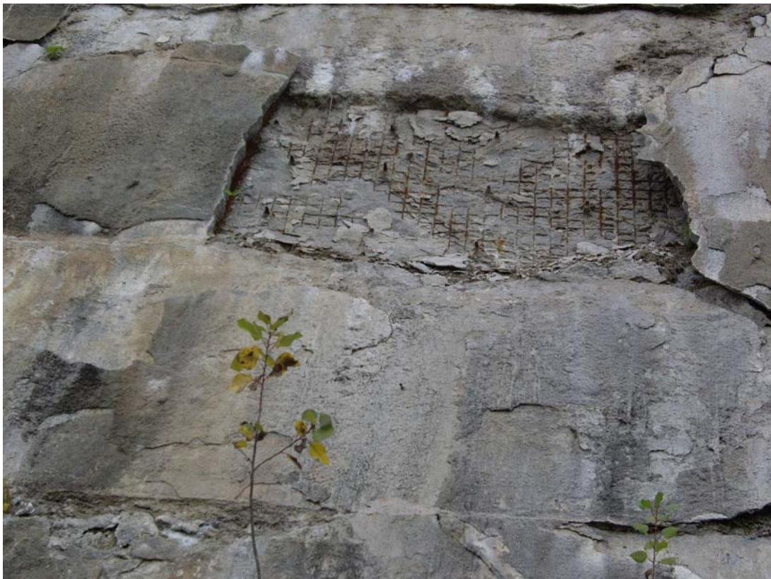
Photo No. 26: A large piece of shotcrete spalled exposing wire mesh in downstream face of dam next to left training wall. Weeds growing in cracks.
