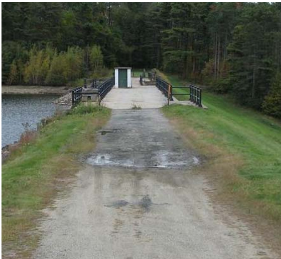
Photo No. 19: Pavement eroded, rutted, and cracked on right crest.
