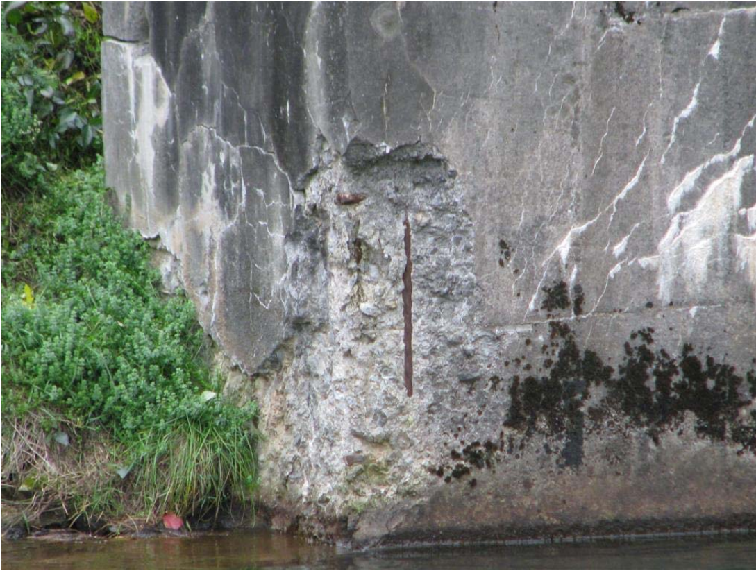
Photo No. 25: Exposed rebar at the end of the right training wall.
