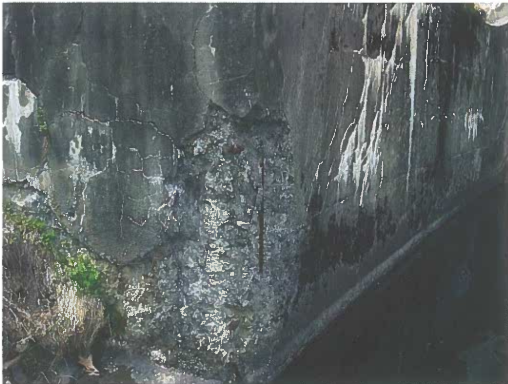
Photo No. 32: Concrete spalling and exposed rebar at the end of the right training wall.
