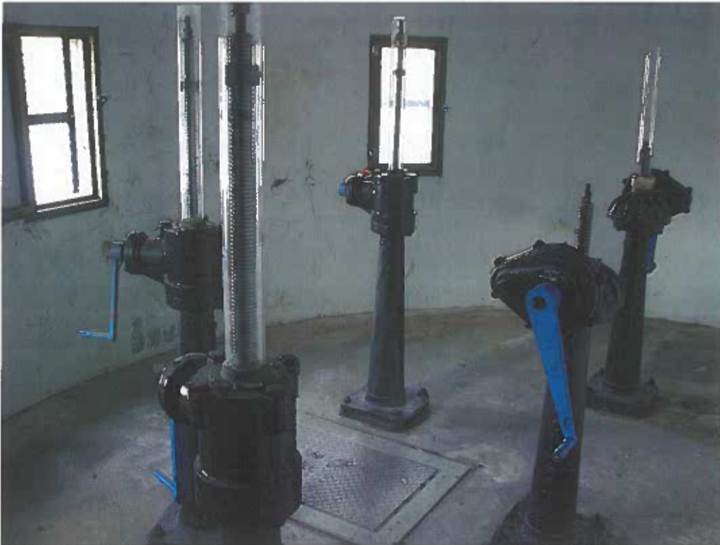
Photo No. 15: Overview of upper gatehouse interior and gate operators – mudgate, 24" x 26" sluice gate low-level outlet, 3 different level gates at reservoir.
