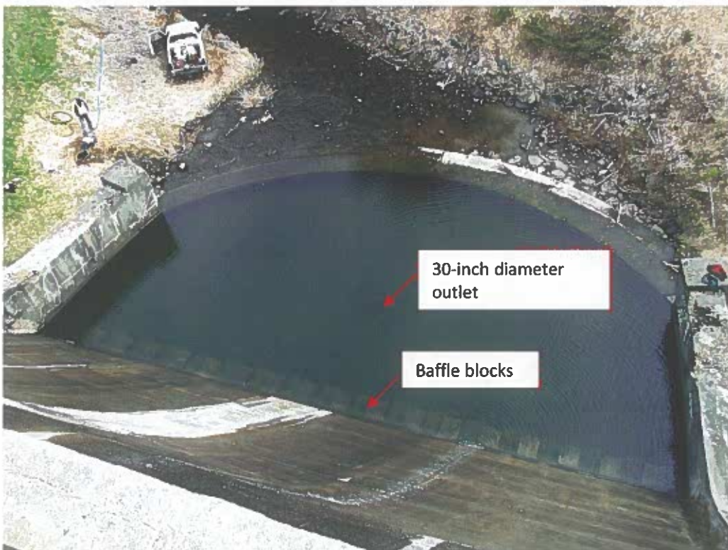
Photo No. 12: Overview of stilling basin looking downstream from the crest. Note variation in elevation of the top of the downstream basin overflow weir.
