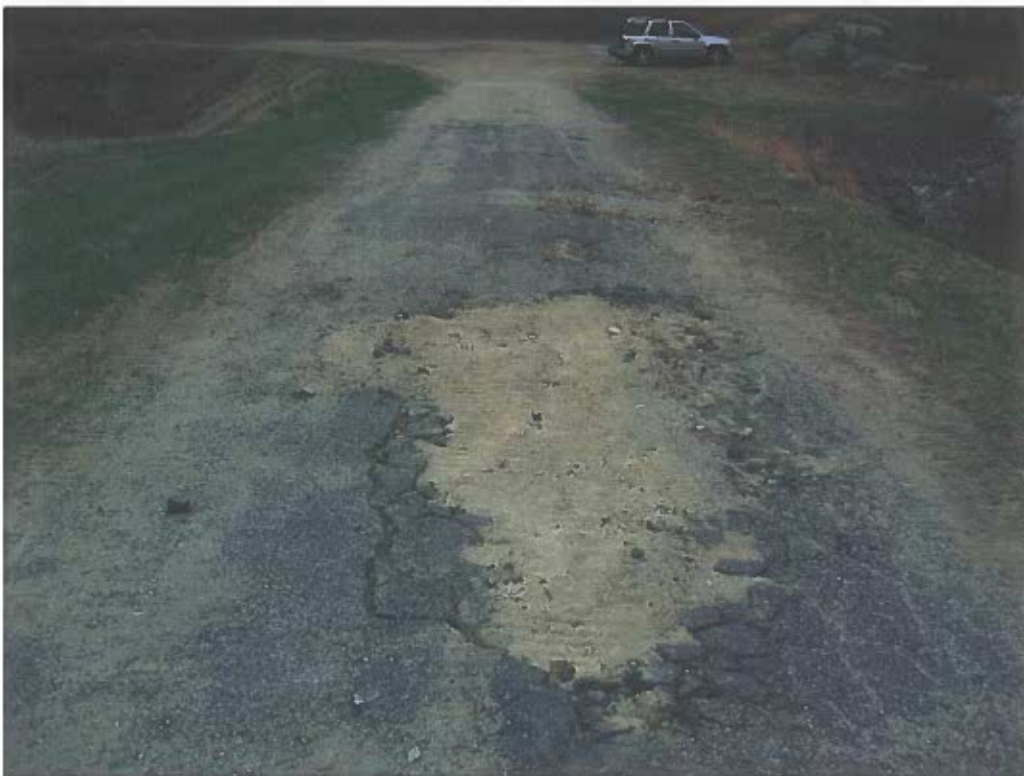
Photo No. 22: Pavement eroded, rutted, and cracked on right crest (looking towards right abutment).
