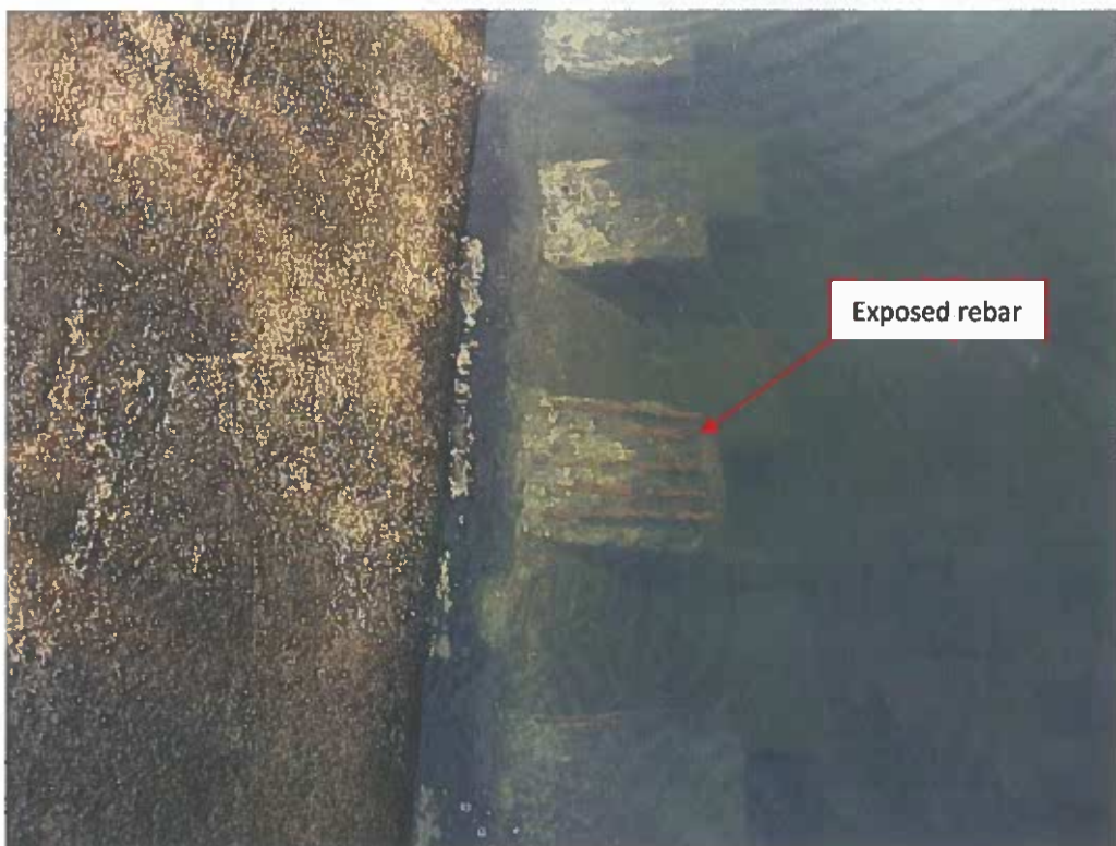
Photo No. 62: Exposed rebar on baffle blocks in stilling basin.
