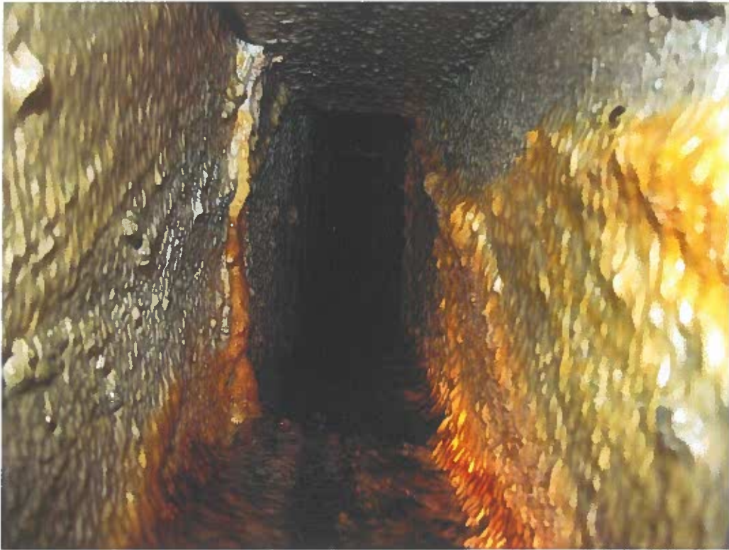
Photo No. 51: Overview interior of typical, rectangular, drainage well (looking up toward dam crest from inspection gallery).
