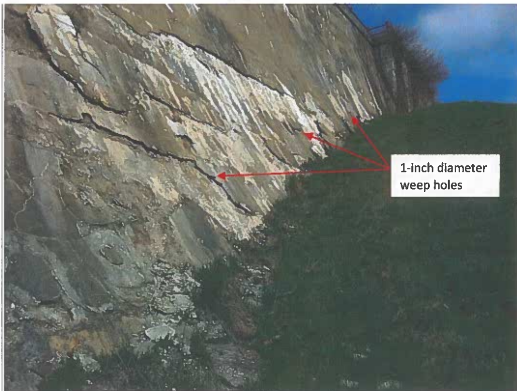
Photo No. 36: PVC weep holes on the downstream face of the dam to left of spillway. Weep holes were installed when dam face was sandblasted and shotcrete-covered in 1981 to 1982.
