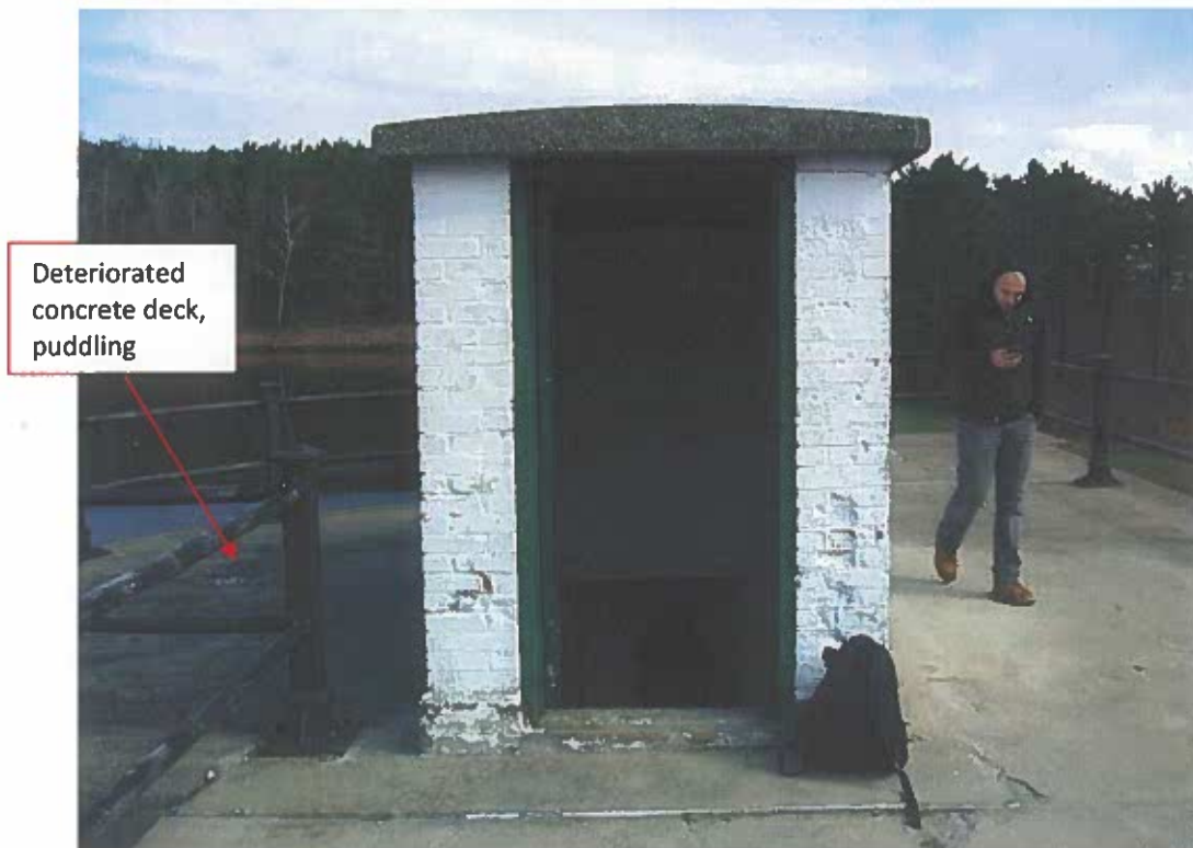
Photo No. 14: Overview of upper gatehouse exterior. Note cracking, spalling, and puddling along concrete deck.
