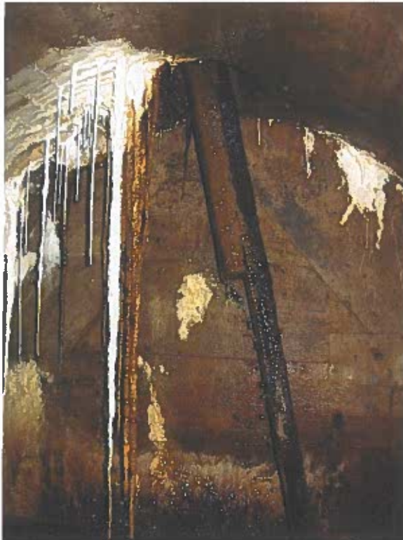
Photo No. 53: Two 2"x4" wood lumber pieces apparently inserted inside left-most drainage well at left end of gallery.
