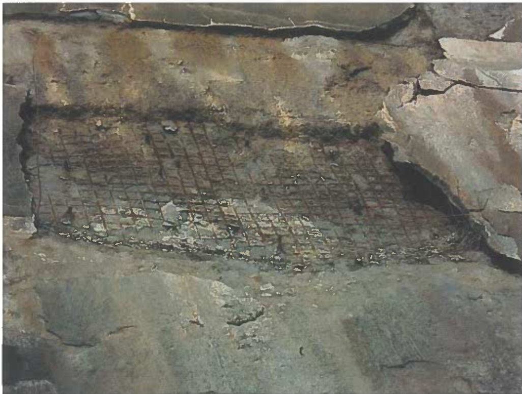
Photo No. 30: A large section of shotcrete spalled exposing wire mesh on the downstream face of dam next to left training wall.
