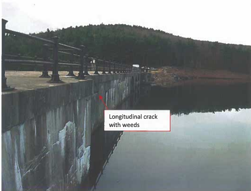
Photo No. 20: Cracks and efflorescence on upstream face of dam. Note that some weeds are growing in the cracks.
