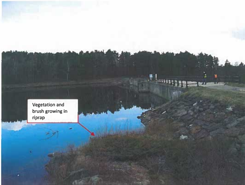
Photo No. 1: Overview of dam and upstream face from right abutment. Note vegetation and brush growing in upstream slope riprap.
