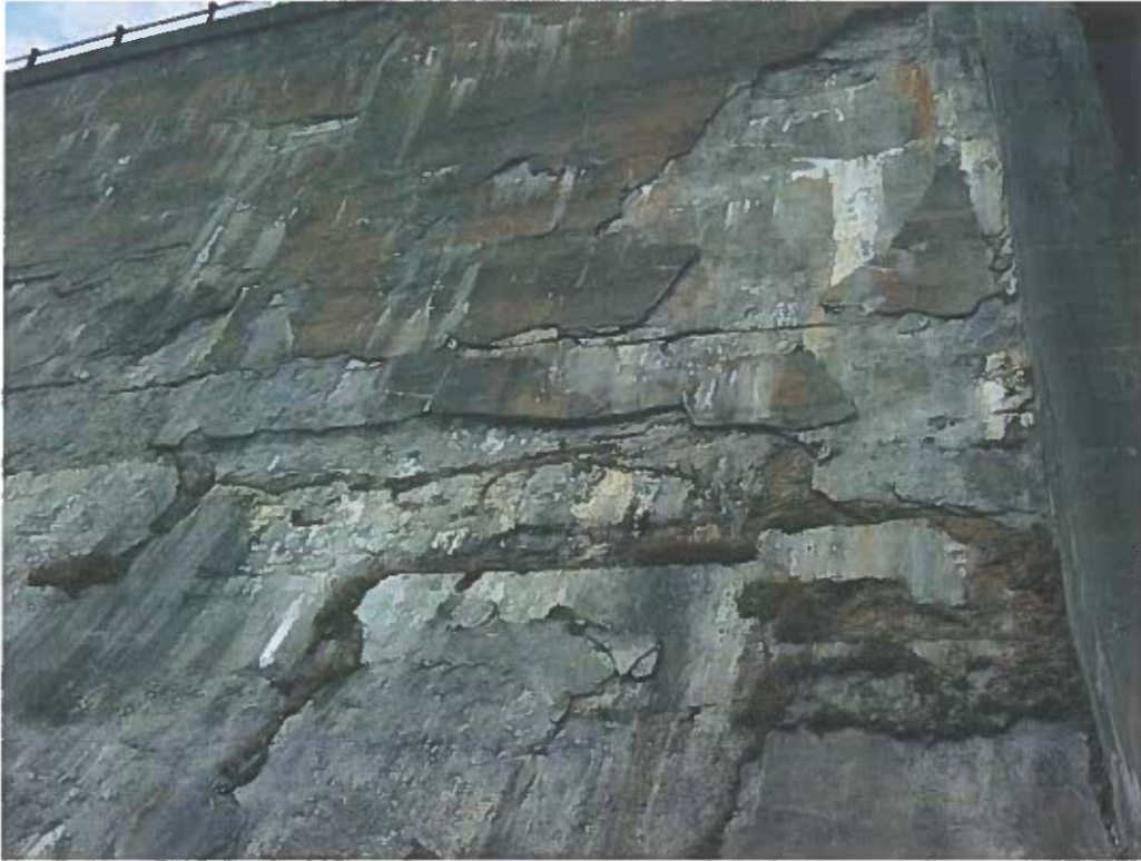
Photo No. 27: A large piece of shotcrete spalled next to the right training wall on the right downstream face. Note weeds growing in the cracks.
