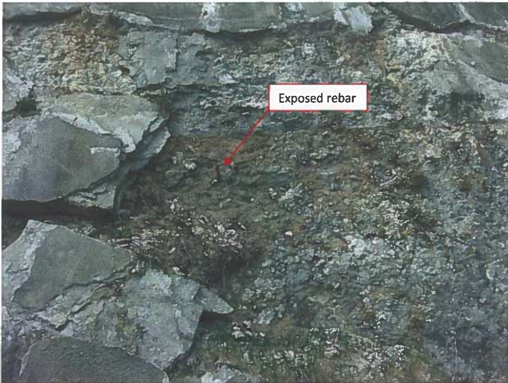
Photo No. 35: Exposed rebar intended to provide anchorage for shotcrete on the downstream face of the dam to right of spillway.
