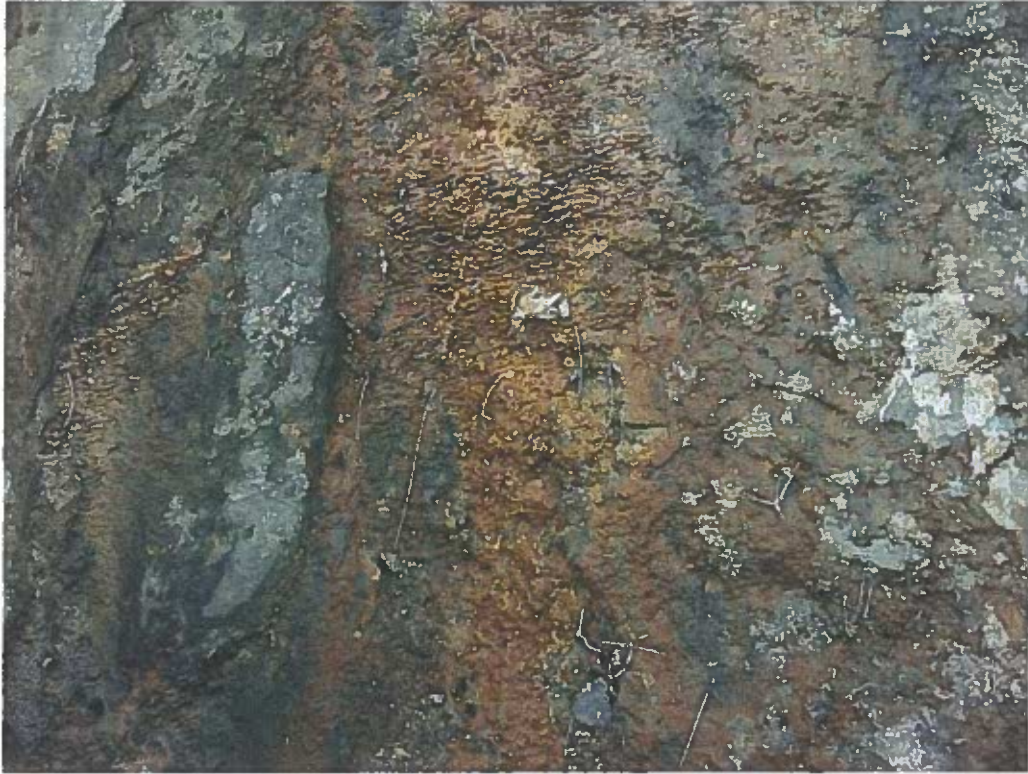
Photo No. 29: Calcium deposits forming to the left of the left training wall.
