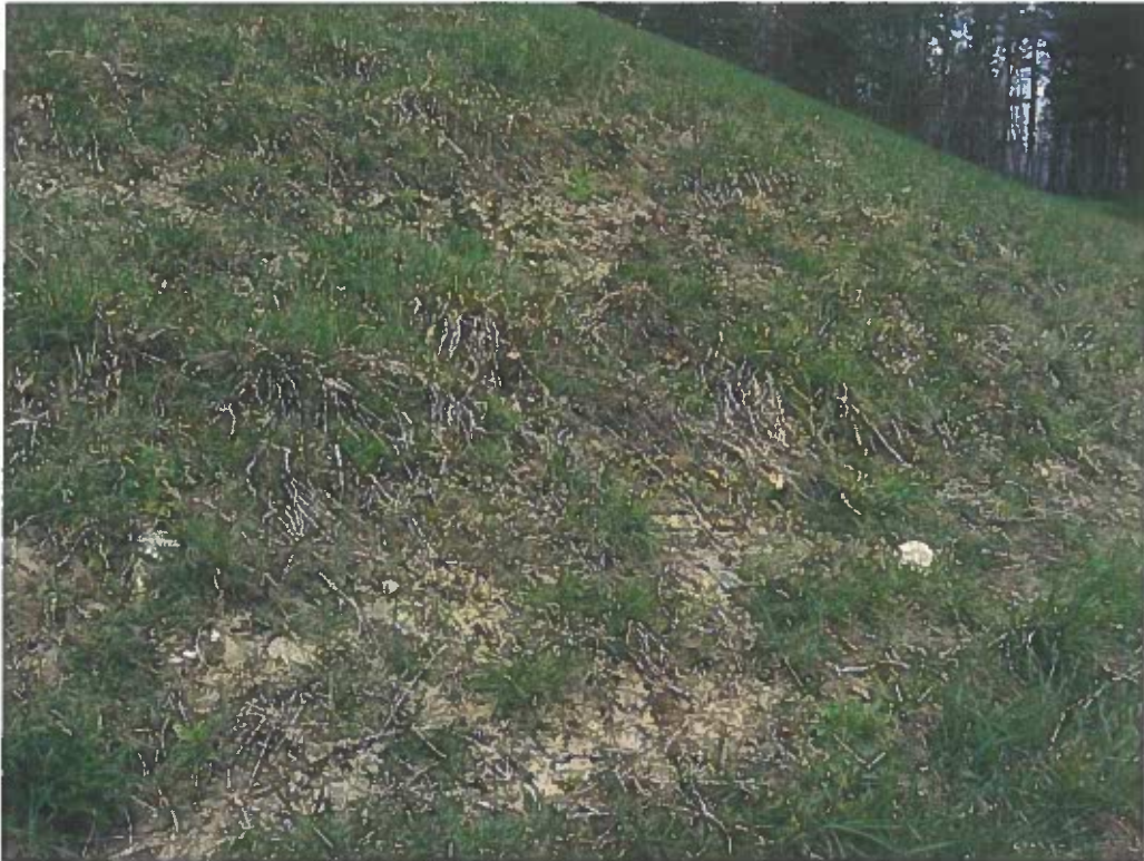
Photo No. 59: Tractor ruts and bare spots on left embankment downstream slope from mowing.
