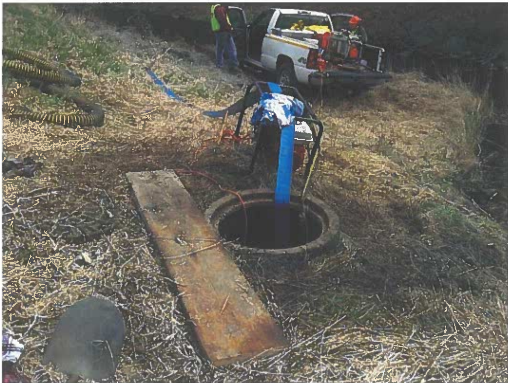
Photo No. 38: Manhole entrance to the inspection gallery under the dam. Water in gallery is pumped out to prepare for access.
