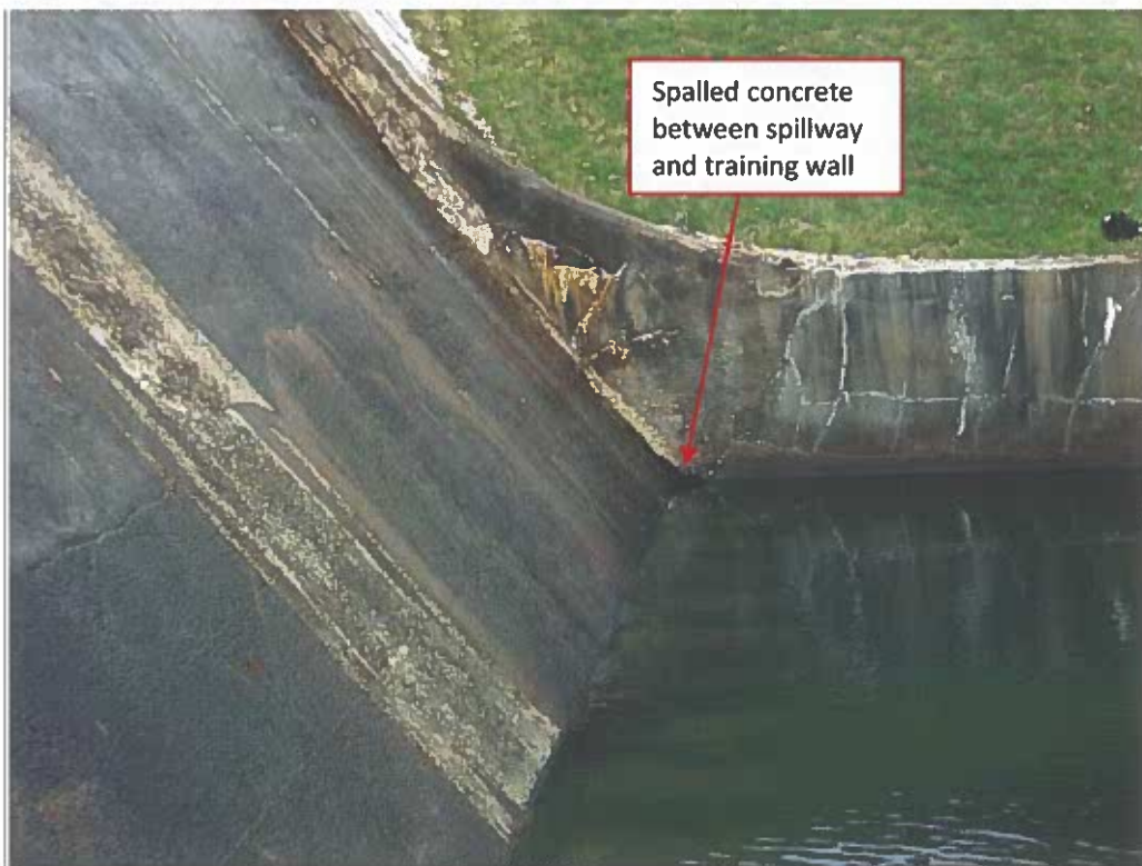
Photo No. 56: Concrete spalled between spillway and training wall at stilling basin. Cracking, spalling, and efflorescence on left training wall.
