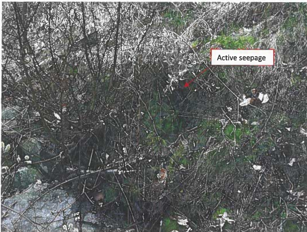
Photo No. 33: Seepage occurring in embankment directly downstream from right training wall.
