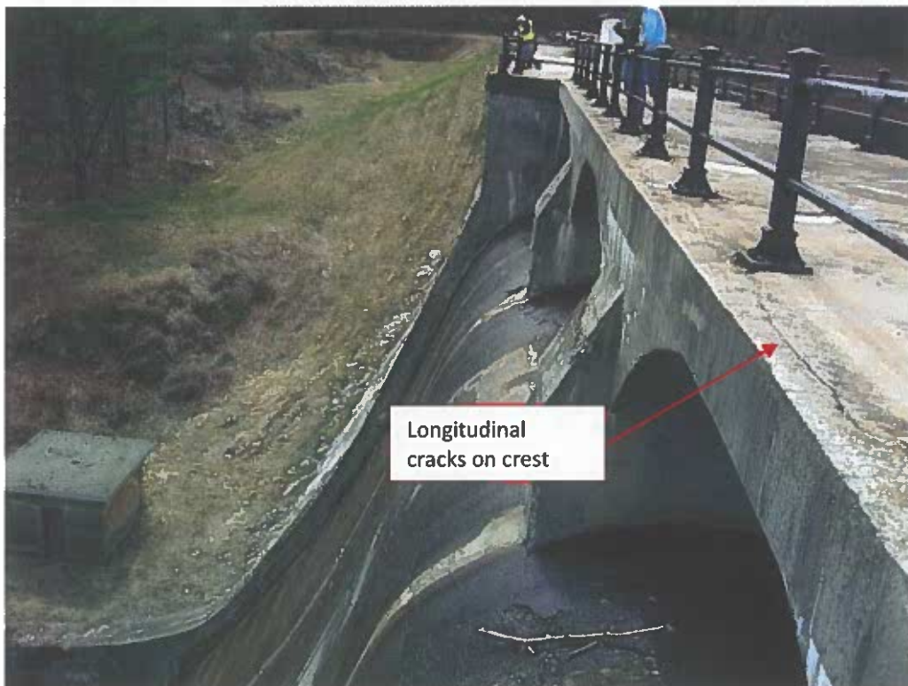
Photo No. 60: Longitudinal cracks along railing. Spalling, cracking, and efflorescence on concrete arch bridge over spillway. Weeds growing in cracks.
