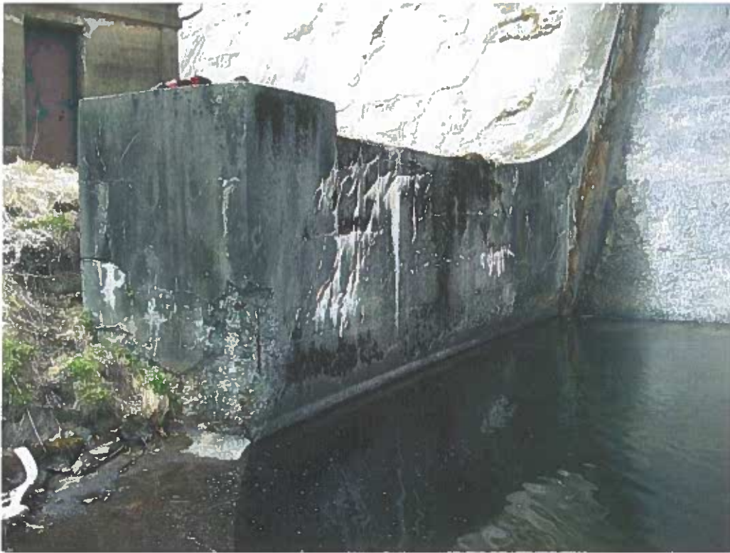
Photo No. 57: Cracking, spalling, and efflorescence on right training wall at stilling basin.
