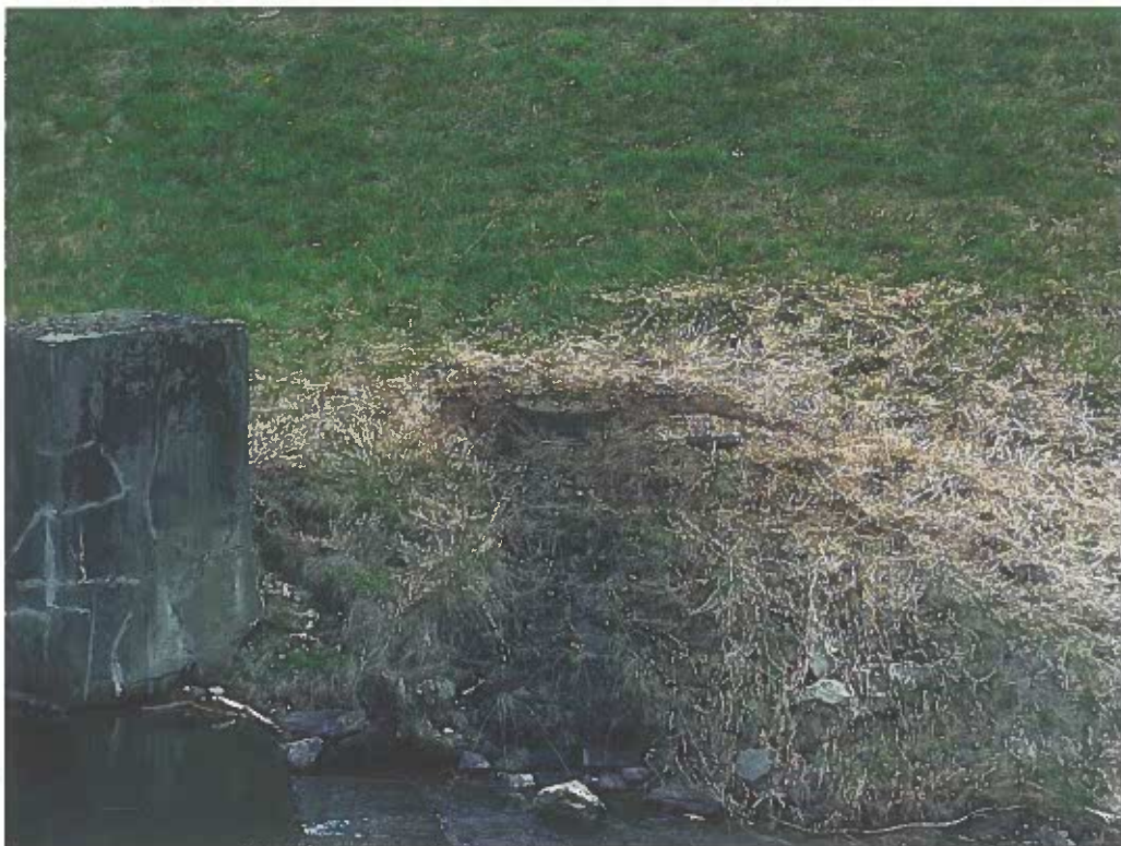
Photo No. 54: Downstream manhole access to drainage gallery. Note that water draining from the top of the drainage gallery manhole is causing erosion of the downstream bank.
