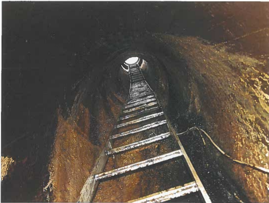
Photo No. 43: Overview of entrance to the inspection gallery from dam crest (looking from the inspection gallery up to the dam crest).
