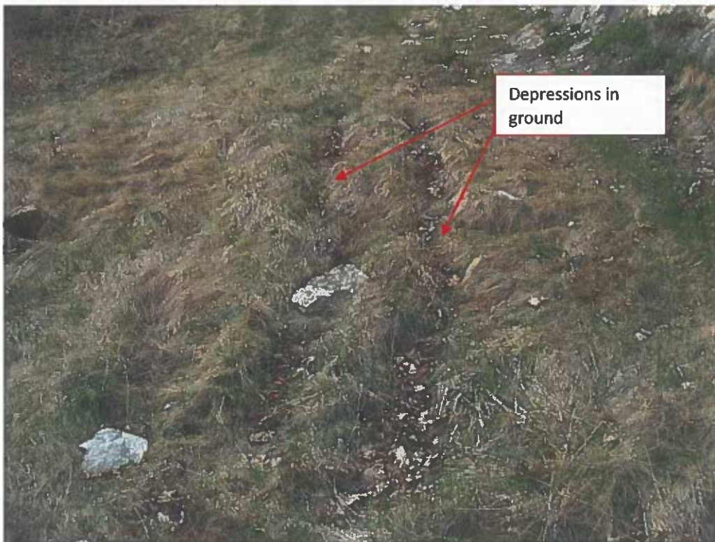
Photo No. 58: Tire ruts on soft, damp ground on right slope between dam face and outlet gatehouse.
