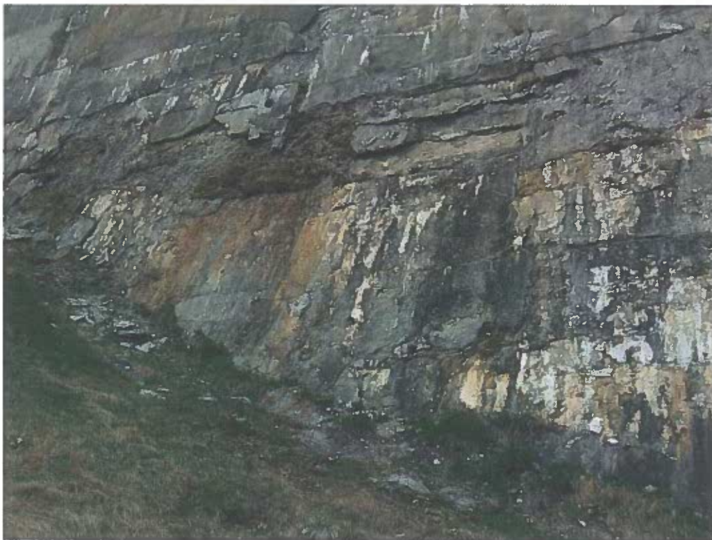
Photo No. 34: Efflorescence, cracking, spalling and weeds growing in the cracks on the downstream face of the dam to right of spillway.
