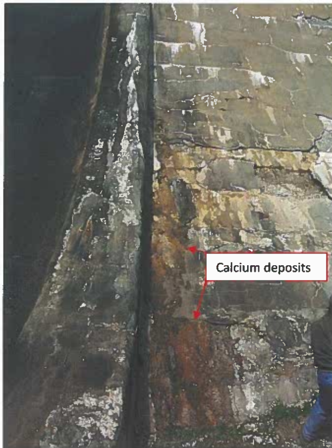
Photo No. 31: Efflorescence and spalling of concrete at toe of left training wall. Note calcium deposits on left downstream face.
