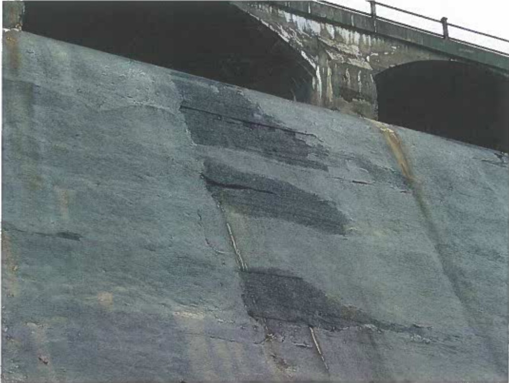
Photo No. 25: Cracks/spalling and efflorescence on the spillway surface (view from downstream).
