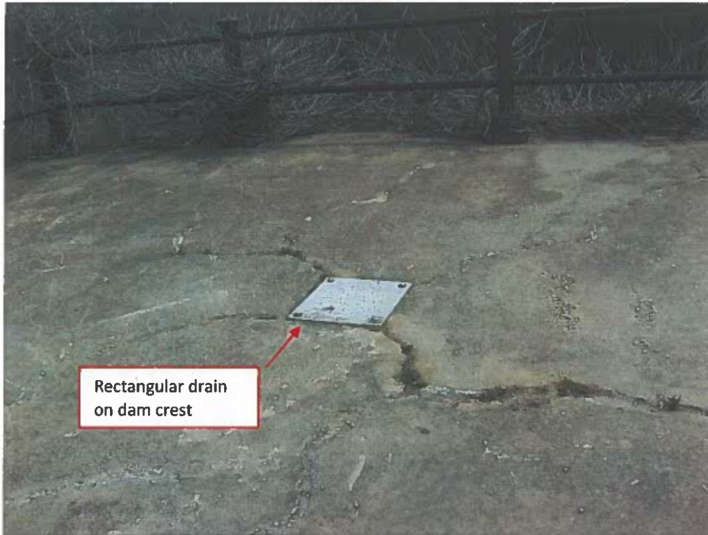
Photo No. 21: Cracks on crest near left embankment. Note minor weeds and moss growing in the cracks. Rectangular drain leads directly to left-most inspection gallery drainage well.
