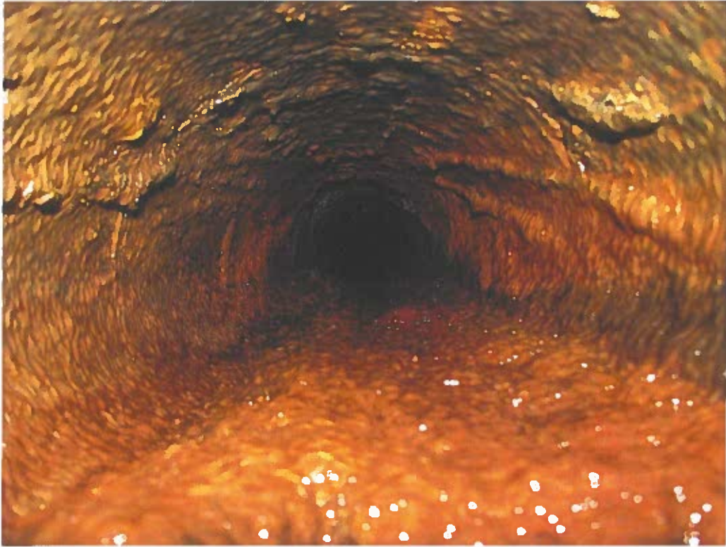
Photo No. 49: Overview interior of typical, round, drainage well (looking up toward dam crest from inspection gallery).
