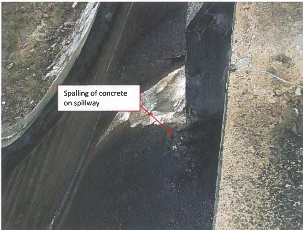
Photo No. 26: Spalling on the spillway surface (view from the crest).
