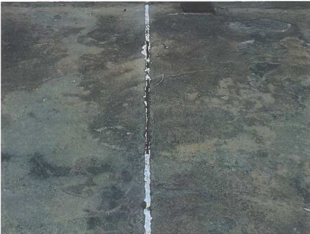
Photo No. 24: Moss and vegetation growing in expansion joints along dam crest.
