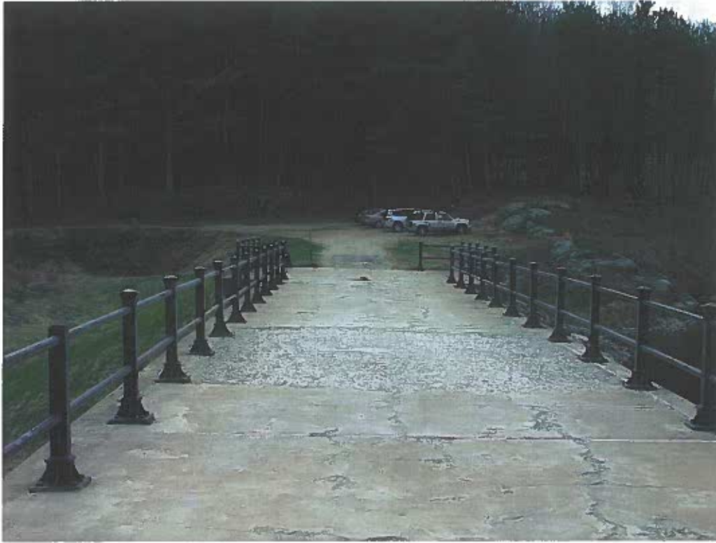
Photo No. 23: Concrete spalled and cracked on right crest (looking towards right abutment).
