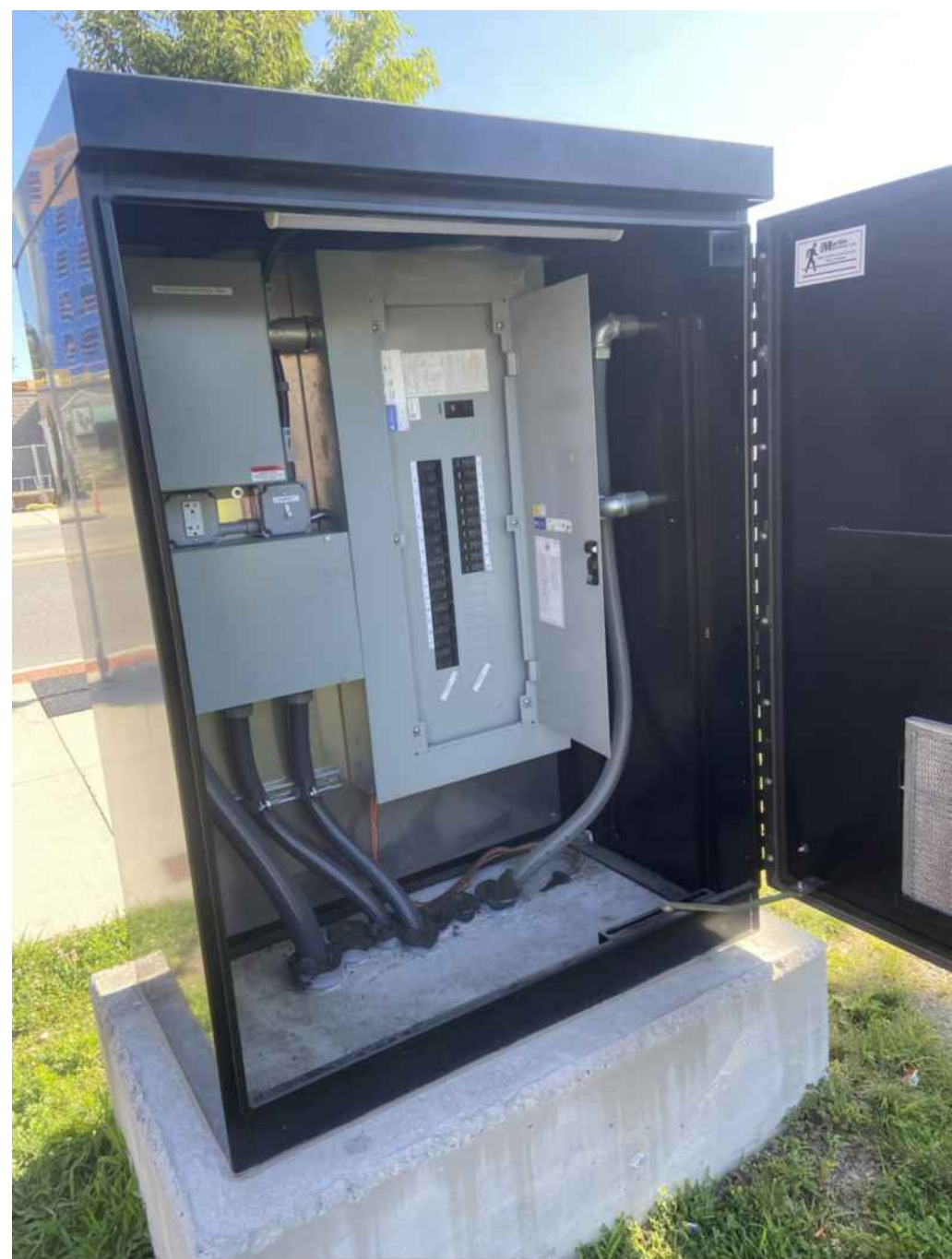
3 PHOTO 2: EXISTING LOAD CENTER IN EXISTING ELECTRICAL ENCLOSURE NOT TO SCALE
