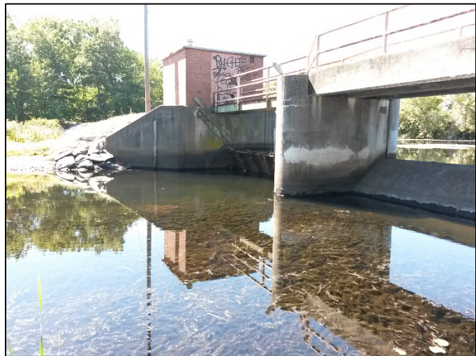
The level of ponded water directly downstream of spillway indicates drawdown beyond three feet will be difficult to achieve
