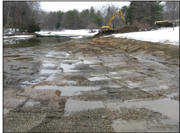
Dredging "in the dry" is usually completed in the winter to simplify sediment management.
