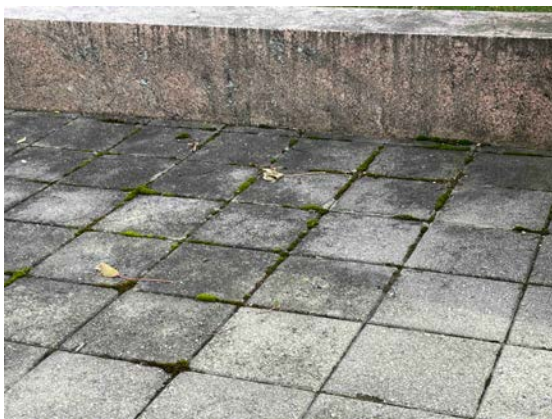
Left: Biomatter in the form of moss has grown between the pavers, and black stains on the pavers and granite wall are the result of carbonaceous staining. Both can be removed with the appropriate cleaners.
