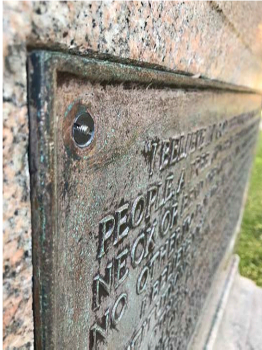
Left: Detail of Plaque 2, showing bare metal from previous blasting, a parched surface, recent formation of corrosion, and missing bronze cap rosettes.
