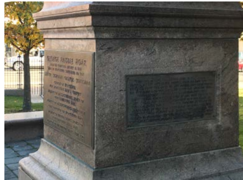
Left: Overall, from the front right corner. Above Right: Granite base from front proper left corner showing dirt, grime, and carbonaceous staining.
