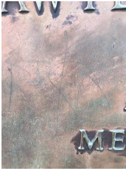
Above: additional details of Plaque 1. Left: the previous blasting to bare copper alloy metal. Right: recent corrosion (drips of copper chloride and black copper sulfate corrosion.)
