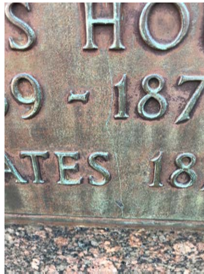
Above: additional details of Plaque 1. Left: the previous blasting to bare copper alloy metal. Right: recent corrosion (drips of copper chloride and black copper sulfate corrosion.)
