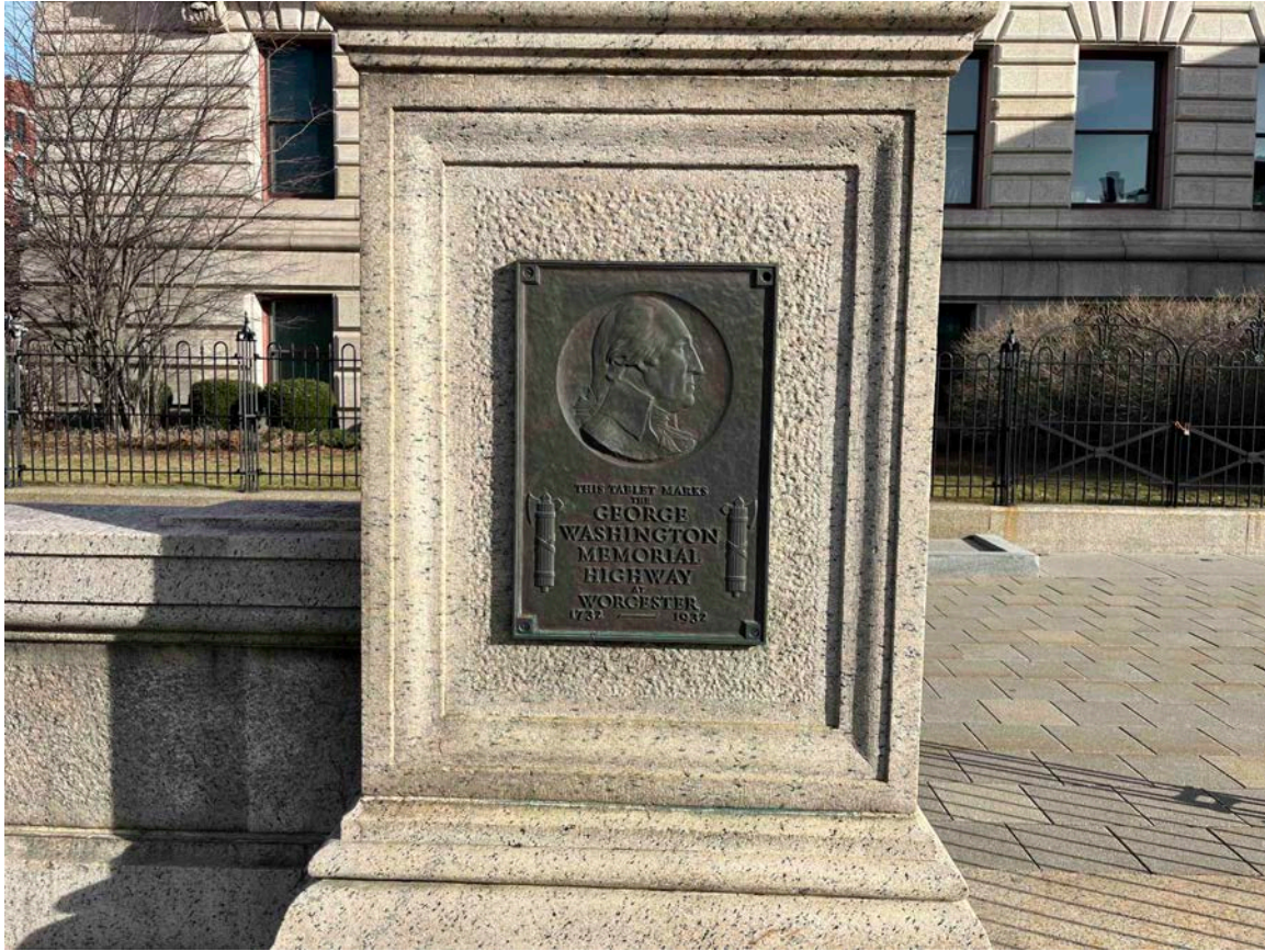
Above: Overall of plaque at the front of City Hall. The plaque is well attached to the granite plinth, and the patina color is accurate. There are some isolated areas of minor abrasions and some green copper corrosion on the front and sides of the plaque.
