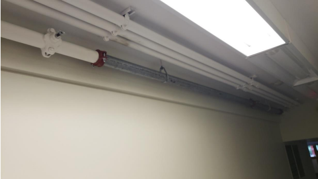
FIGURE 5: REPAIR WITH GALVANIZED PIPE
