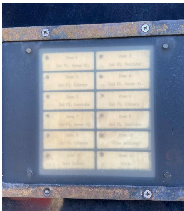
FIGURE 2: REMOTE ANNUNCIATOR PANEL
