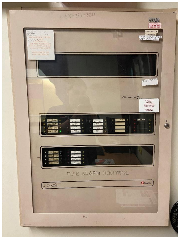
FIGURE 1: MAIN FIRE ALARM CONTROL UNIT (FACU)
