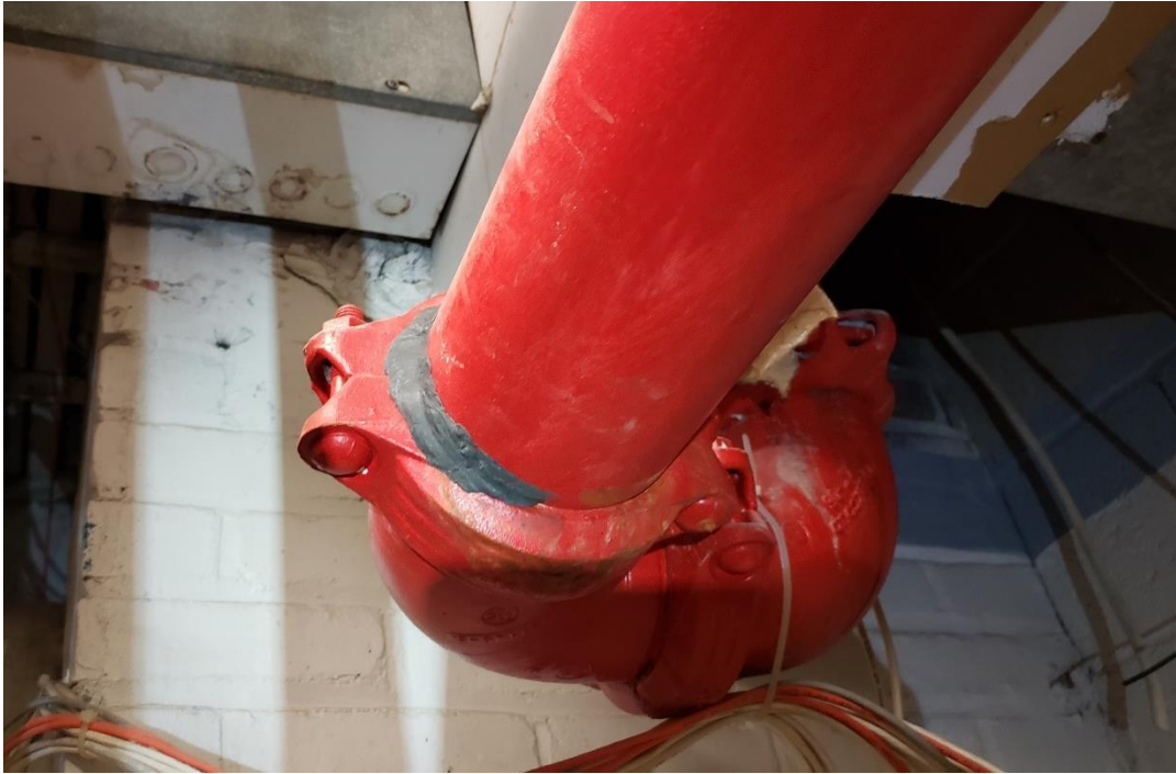
FIGURE 7: EPOXY ON GROOVE-LOCK COUPLING TO REPAIR LEAK
