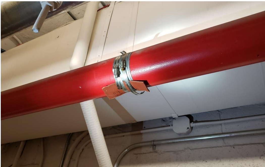
FIGURE 6: CARDBOARD AND HOSE CLAMPS USED TO REPAIR LEAK
