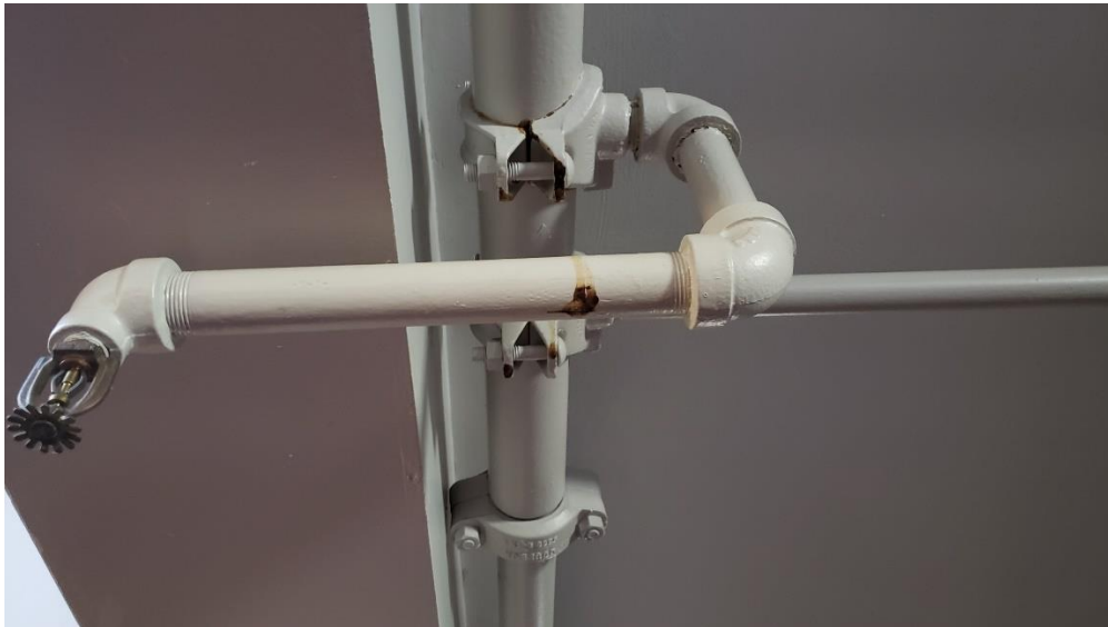
FIGURE 4: PIPING SEGMENT TRAPPING WATER (TYPICAL)
