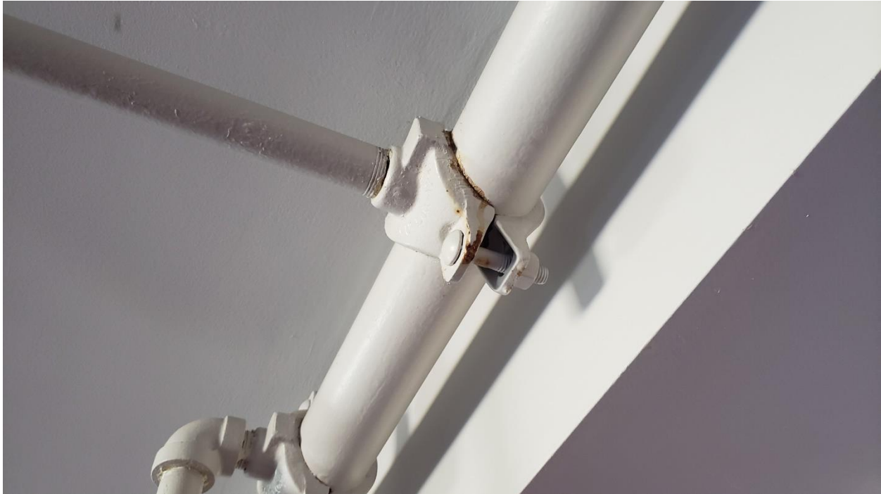
FIGURE 8: CORROSION AT MECHANICAL TEE
