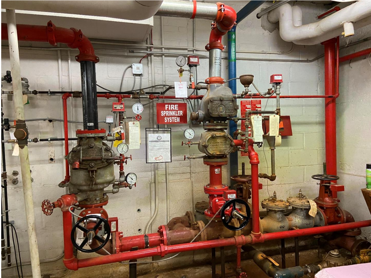
FIGURE 3: SPRINKLER SYSTEM RISERS
