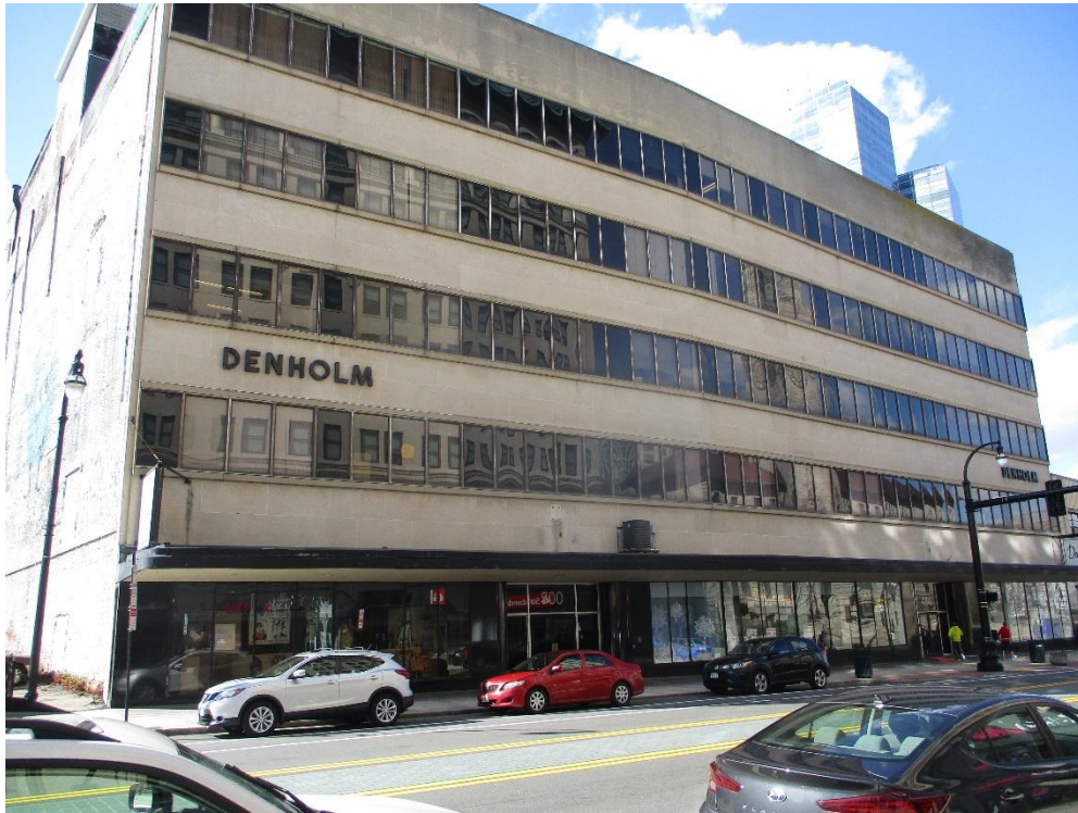
Front of the Building on Parcel 1
