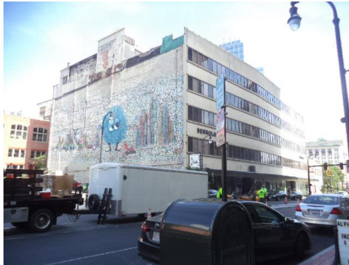
REPRESENTATIVE VIEW OF SUBJECT PROPERTY
