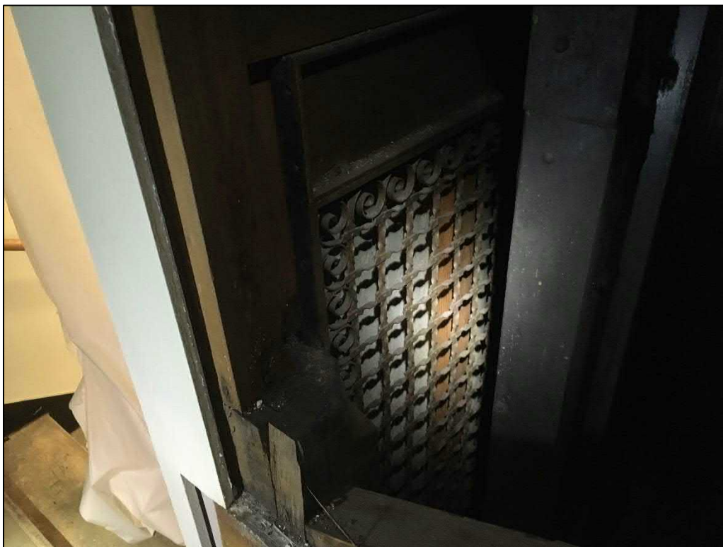
Possible transite panel in freight elevator shaft
