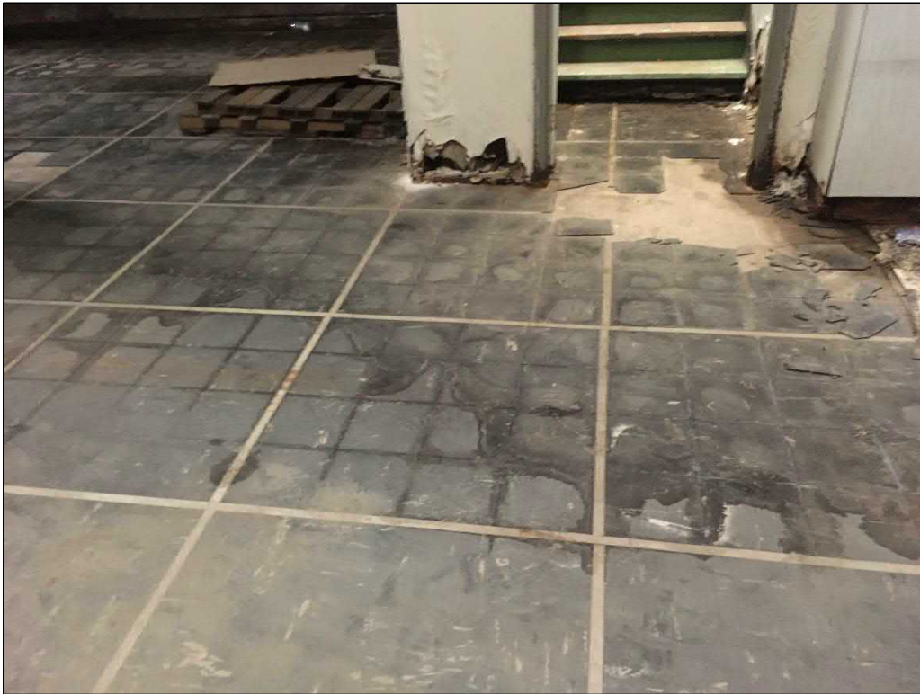
Black 9"x9" floor tiles in basement; 3% asbestos
