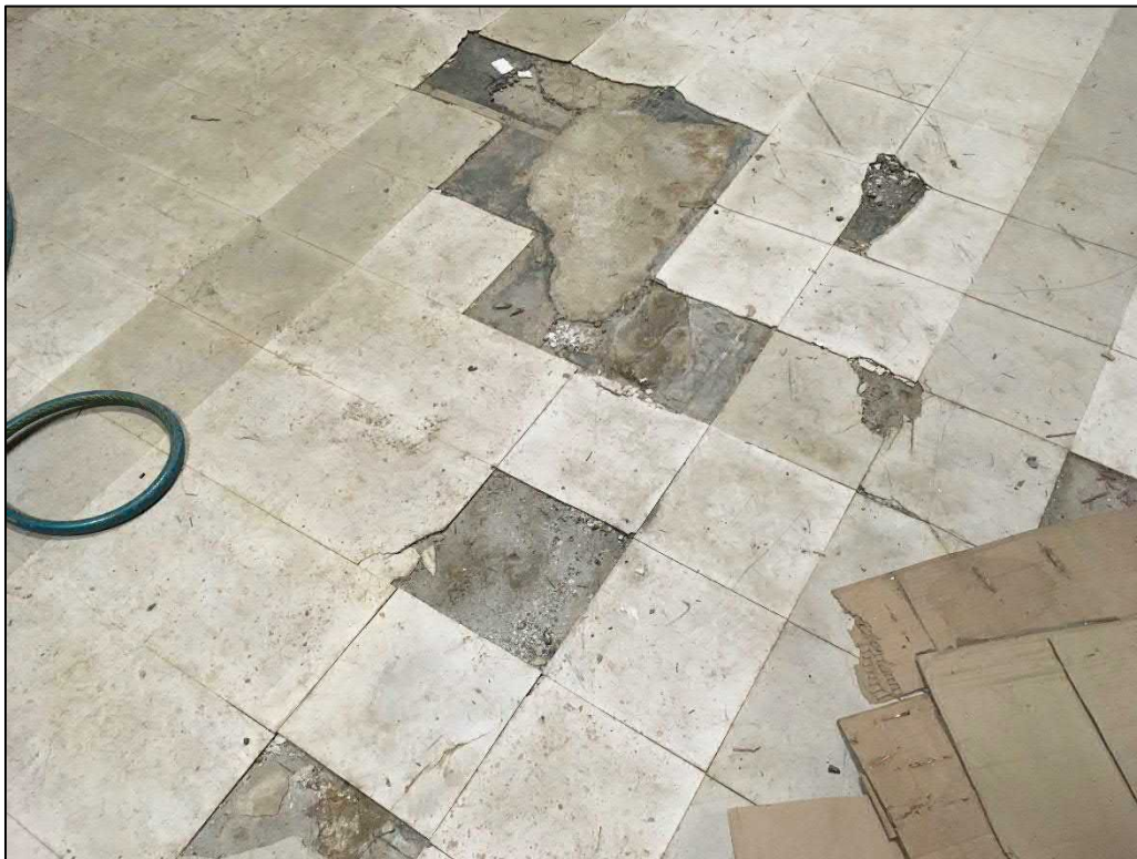
Beige 12"x12" tiles w. mastic (8% asbestos) over black 9"x9" tiles (3% asbestos) over gray leveler (10% asbestos)
