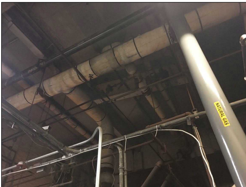
TSI on piping above boilers
