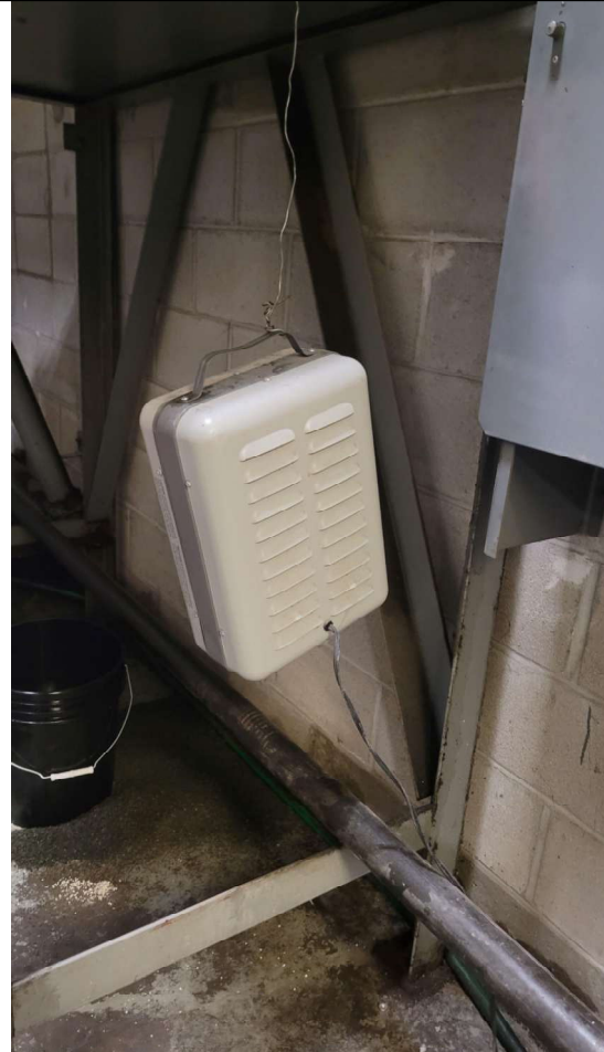
PHOTO 3 - EXISTING ELECTRIC UNIT HEATER IN ELEVATOR MACHINE ROOM
