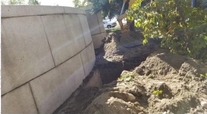
Photo 7 - TP-2 - Overall View
