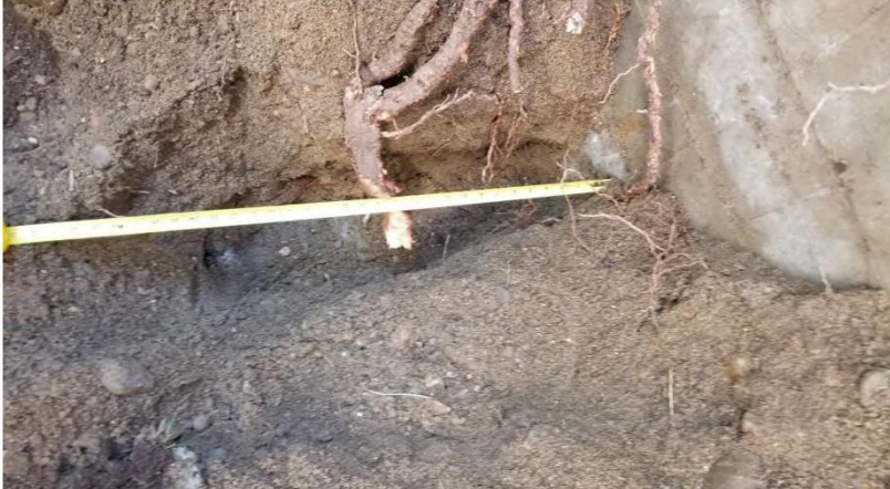
Photo 11 - TP-3 - View of Foundation
