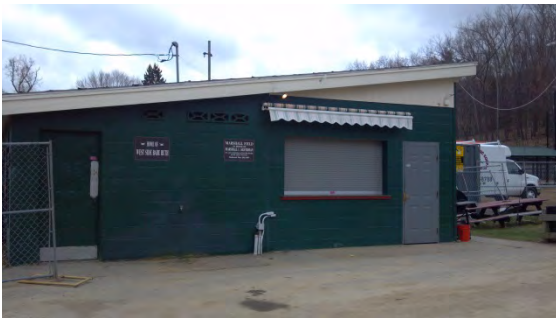
Existing Conditions Photo C
