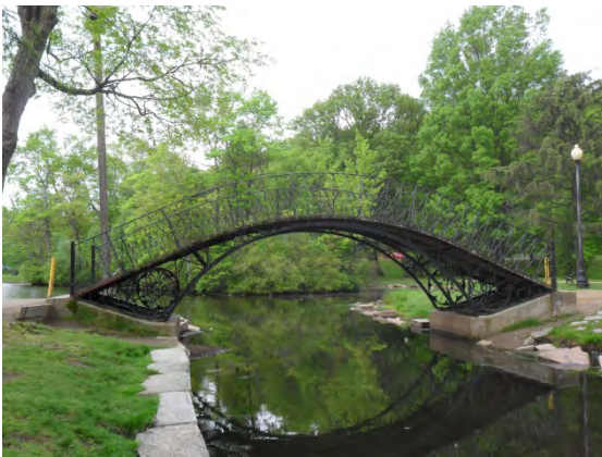
Existing Conditions Photo C
