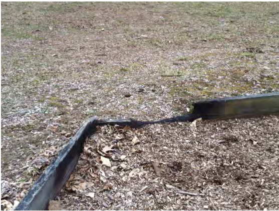
Existing Conditions Photo C
