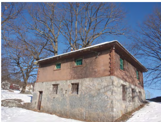
Existing Conditions Photo J
