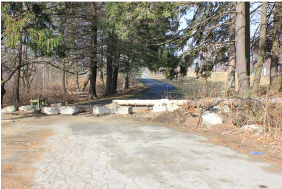
Existing Conditions Photo C
