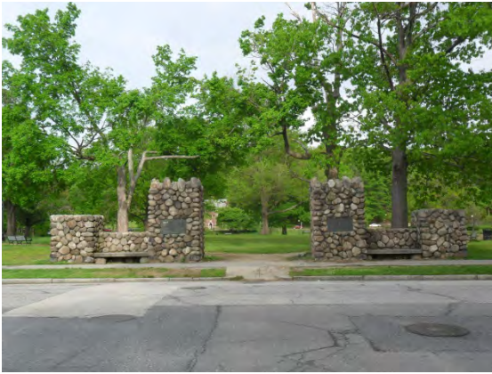
Existing Conditions Photo A
