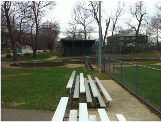
Existing Conditions Photo G
