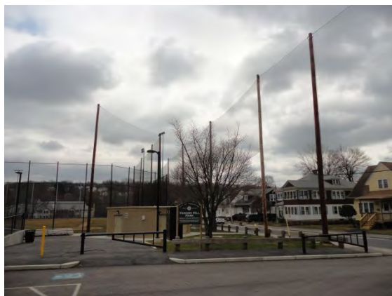
Existing Conditions Photo JJ
