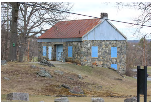
Existing Conditions Photo O
