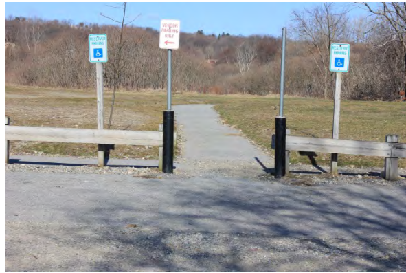
Existing Conditions Photo B
