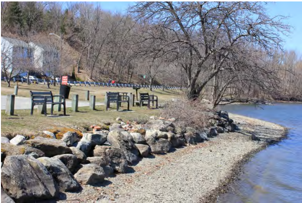
Existing Conditions Photo C
