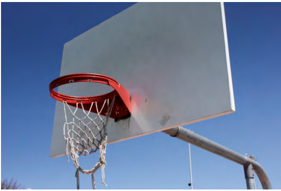
Existing Conditions Photo G
