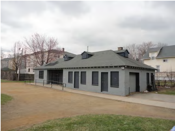
Existing Conditions Photo A
