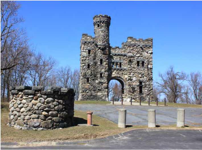
Existing Conditions Photo C
