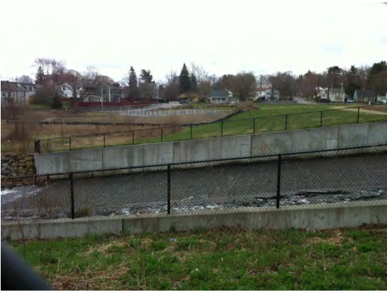
Existing Conditions Photo B
