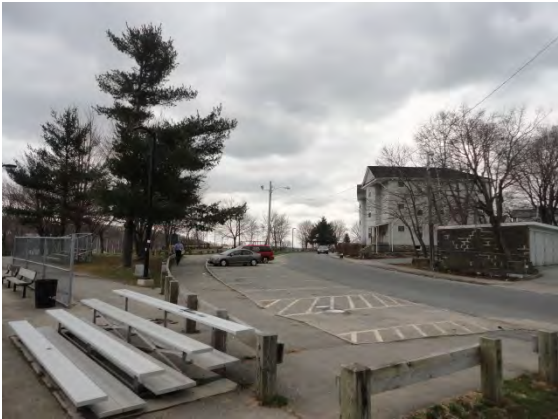
Existing Conditions Photo Z
