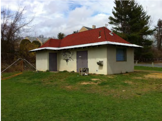
Existing Conditions Photo F
