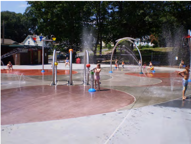
Existing Conditions Photo O
