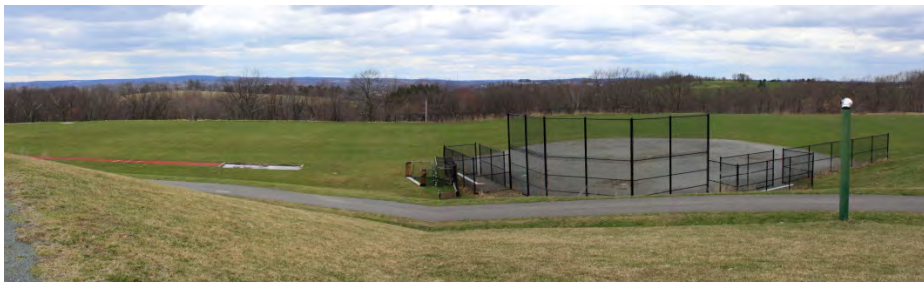
Existing Conditions Photo O
