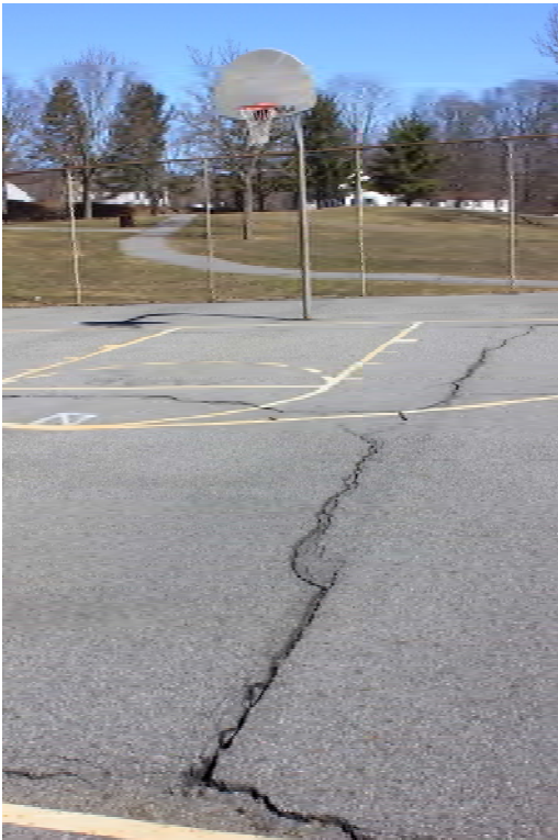
Existing Conditions Photo C
