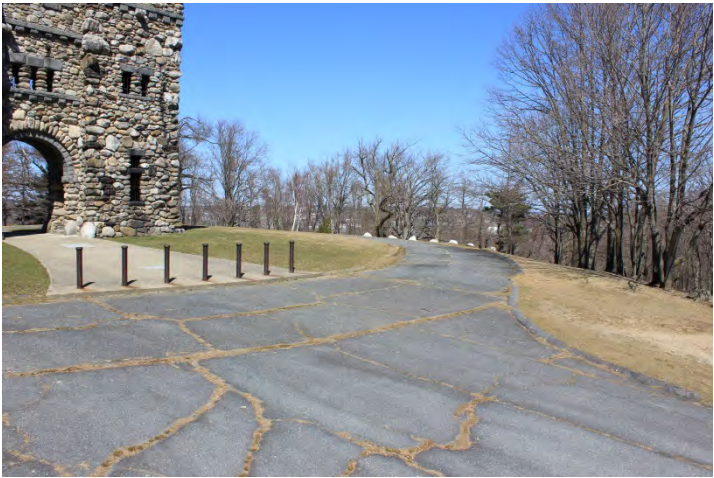
Existing Conditions Photo B
