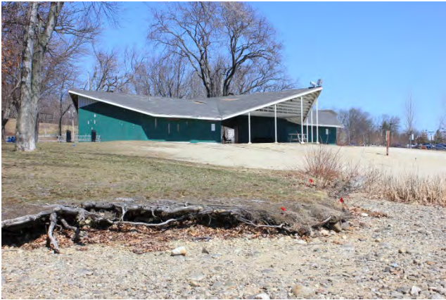
Existing Conditions Photo C
