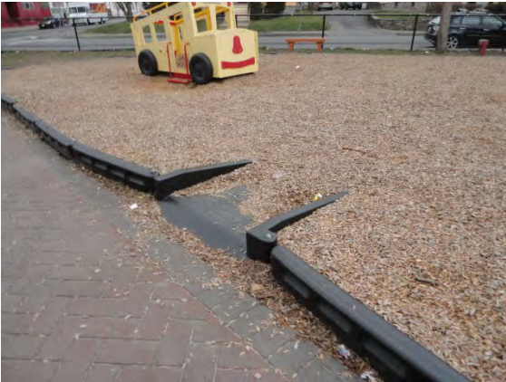
Existing Conditions Photo I
