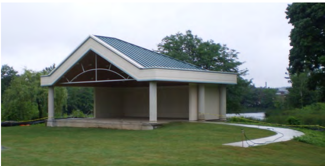
Existing Conditions Photo G
