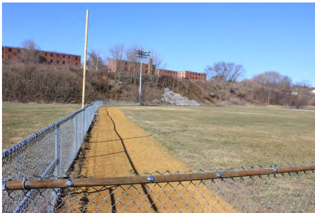
Existing Conditions Photo C
