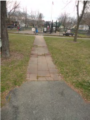
Existing Conditions Photo I
