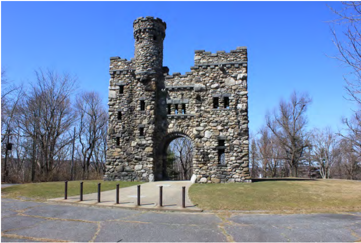
Existing Conditions Photo A
