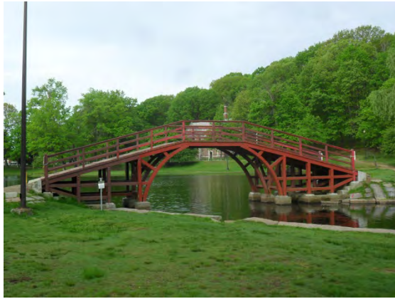
Existing Conditions Photo B
