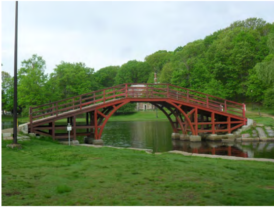
Existing Conditions Photo B
