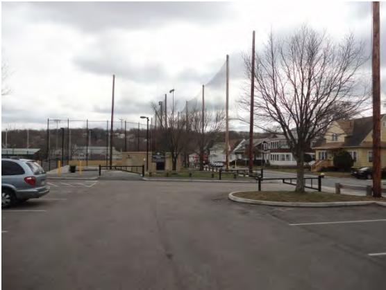
Existing Conditions Photo A
