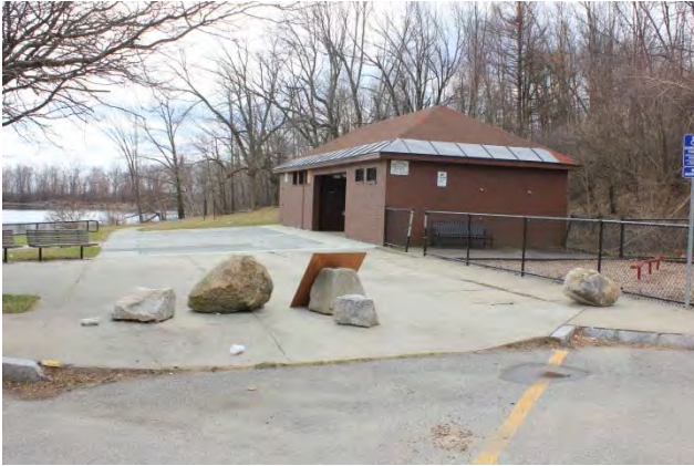
Existing Conditions Photo A
