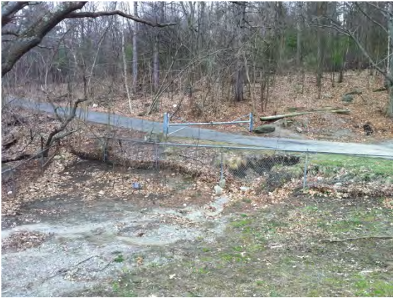
Existing Conditions Photo I
