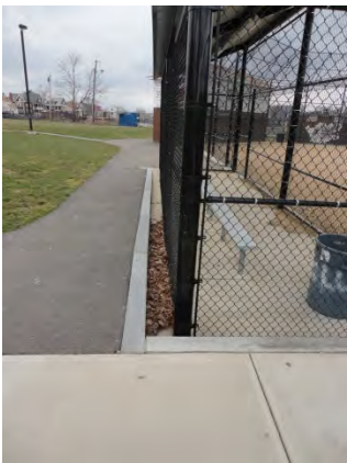
Existing Conditions Photo W
