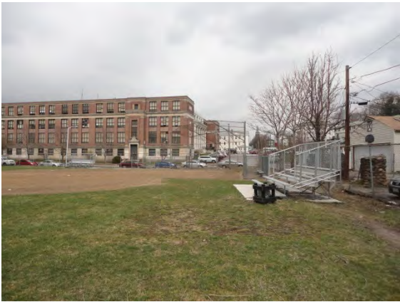
Existing Conditions Photo MM
