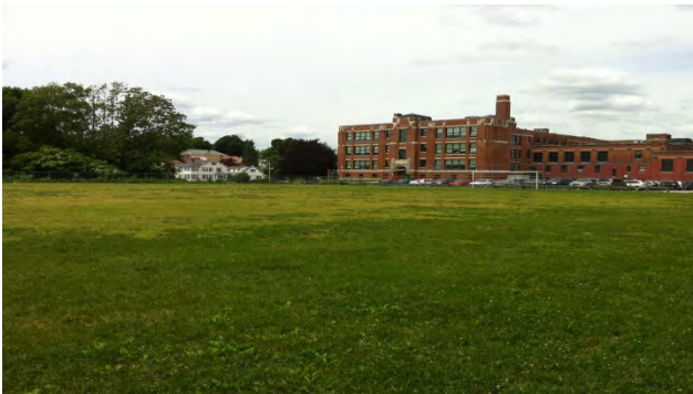
Existing Conditions Photo L
