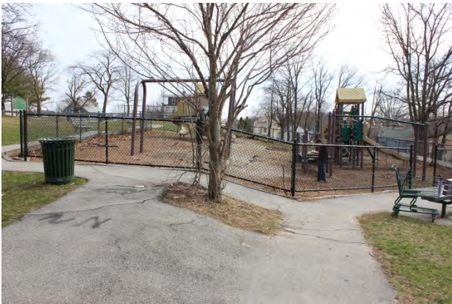
Existing Conditions Photo A
