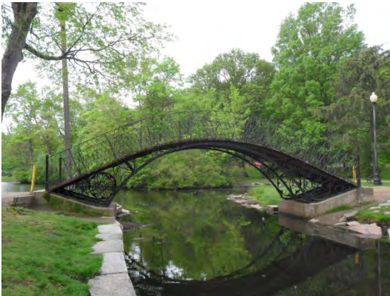
Existing Conditions Photo C
