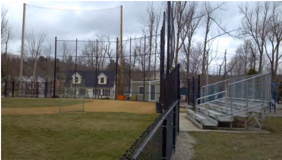
Existing Conditions Photo C
