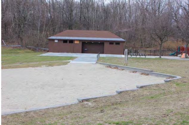
Existing Conditions Photo B
