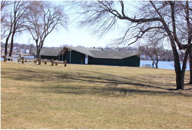
Existing Conditions Photo B
