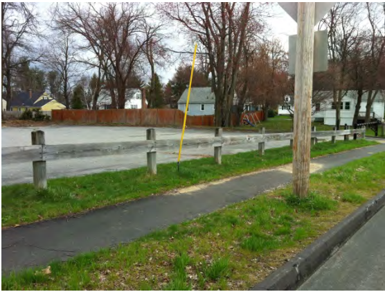
Existing Conditions Photo A
