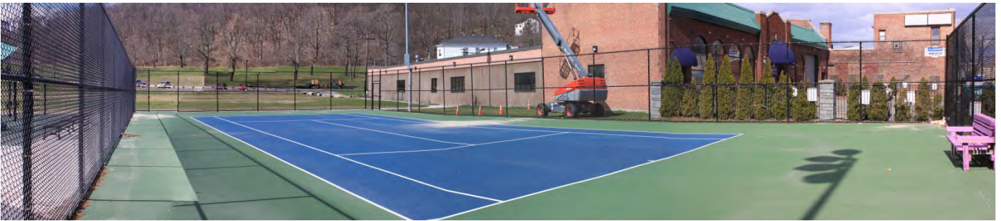
Existing Conditions Photo B
