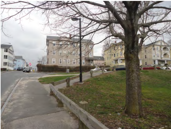
Existing Conditions Photo GG
