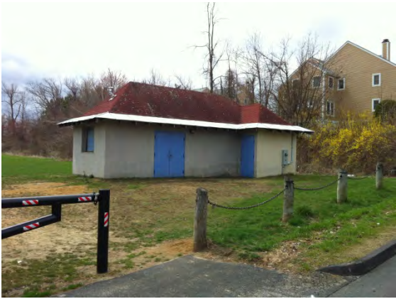
Existing Conditions Photo B
