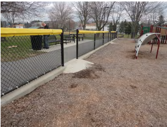
Existing Conditions Photo Q
