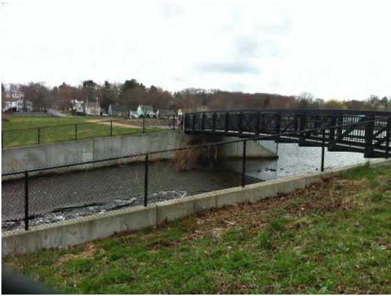
Existing Conditions Photo A
