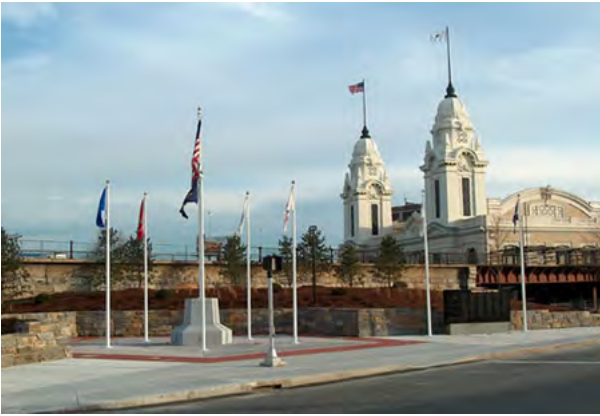
Existing Conditions Photo A
