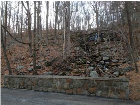
Existing Conditions Photo B
