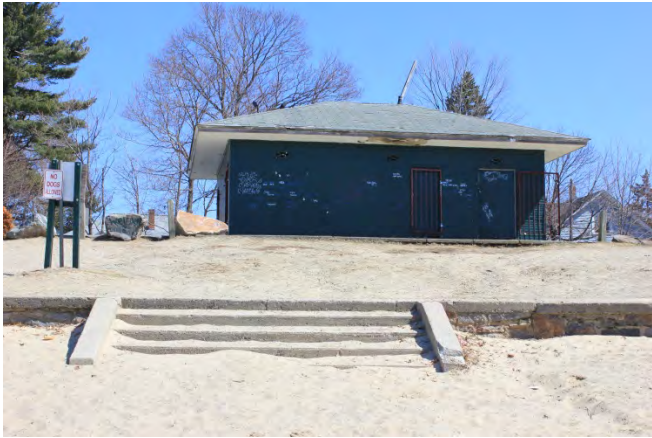
Existing Conditions Photo A
