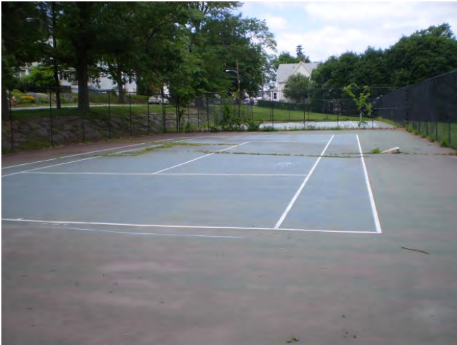
Existing Conditions Photo M
