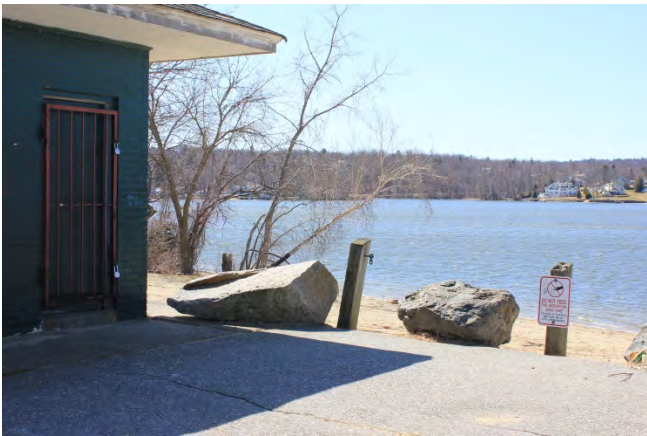
Existing Conditions Photo C
