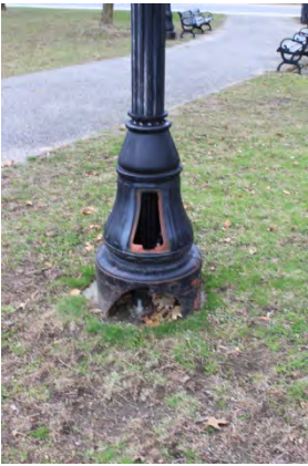
Existing Conditions Photo G
