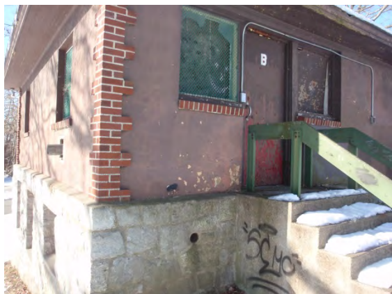
Existing Conditions Photo I
