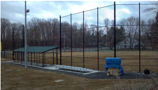
Existing Conditions Photo G
