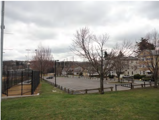
Existing Conditions Photo I
