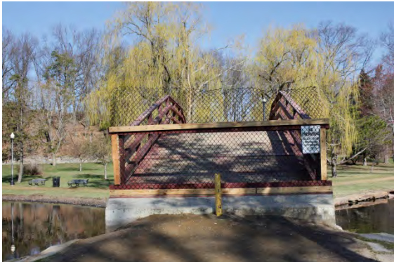
Existing Conditions Photo J
