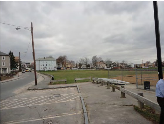
Existing Conditions Photo BB
