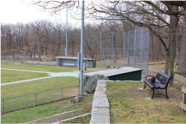
Existing Conditions Photo B
