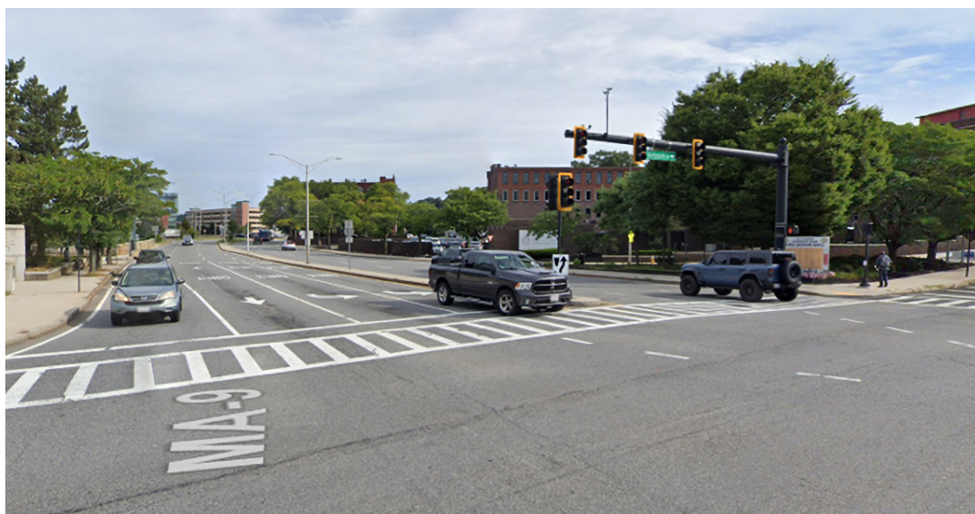
Figure 6 Wide roads, slip lanes, narrow sidewalks, and fast vehicle traffic create an uncomfortable walking and rolling environment along Lincoln Street at I-290
