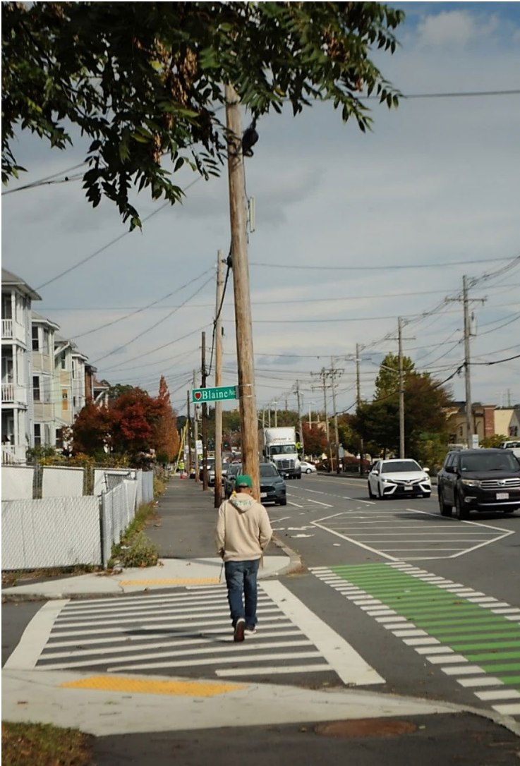
Figure 1: New lane marking treatments and American Disabilities Act (ADA) accessible curb ramps on Stafford Street.
