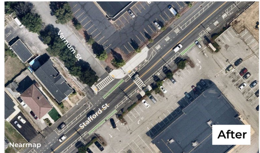
Figure 14: Stafford Street before and after roadway safety improvements including buffered bike lanes, bus stops, crosswalks, curb extension, and RRFBs.
