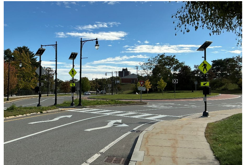
Figure 16: New RRFBs installed at the North Lake Avenue roundabout.
