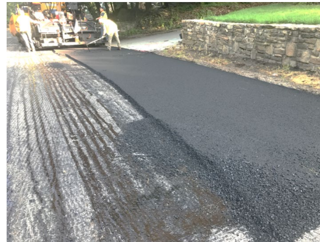
Figure 9: Mill and overlay pavement treatment.
