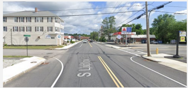
Figure 18: Intersection at Clover St and Ludlow St before improvements (Source: Google Maps 2023).
