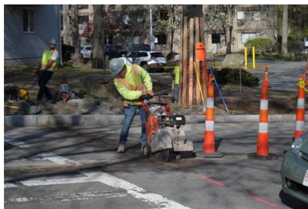
Figure 20: 2026 construction of raised crosswalks on Country Club Boulevard.
