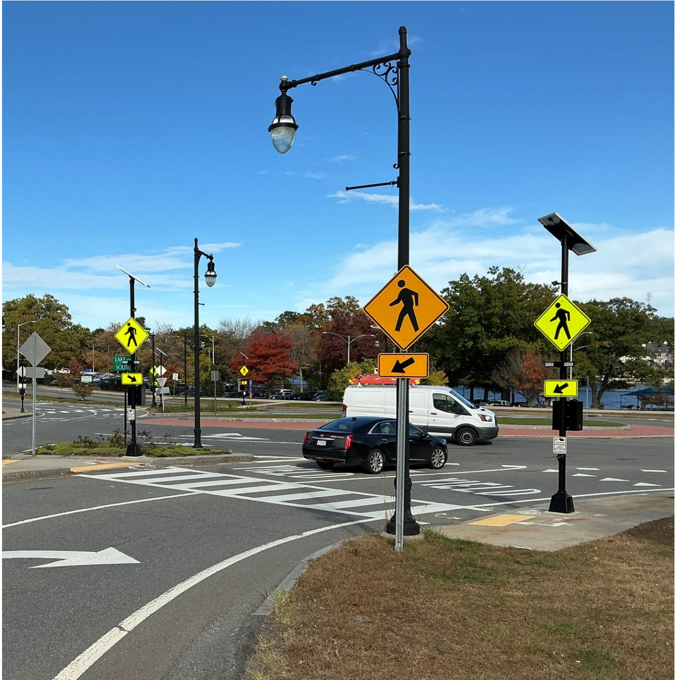
Figure 9: New Rectangular Reflective Flashing Beacon (RRFB) lights installed at the North Lake Ave roundabout
