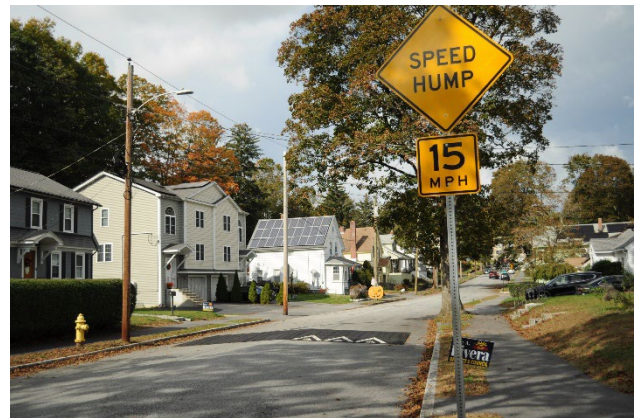
Figure 8: Permanent speed humps were installed on Beacon Street in 2025.
