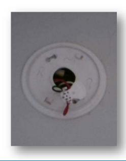
Smoke alarm is not installed inside each sleeping area, outside each sleeping area, and on each level.
