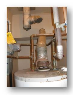
Chimney or flue piping is blocked, misaligned, or missing (i.e., evidence of prior installation, but now not present or is incomplete).
