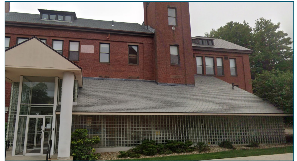
Example of a synthetic slate roof on Pleasant Street
