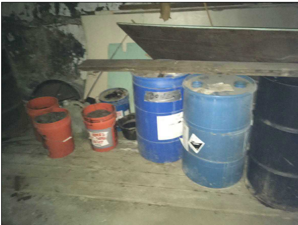
OHMs in boiler room
