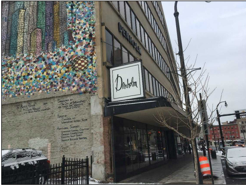
Site structure, looking north along Main Street
