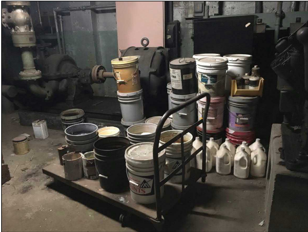
OHMs near generator room
