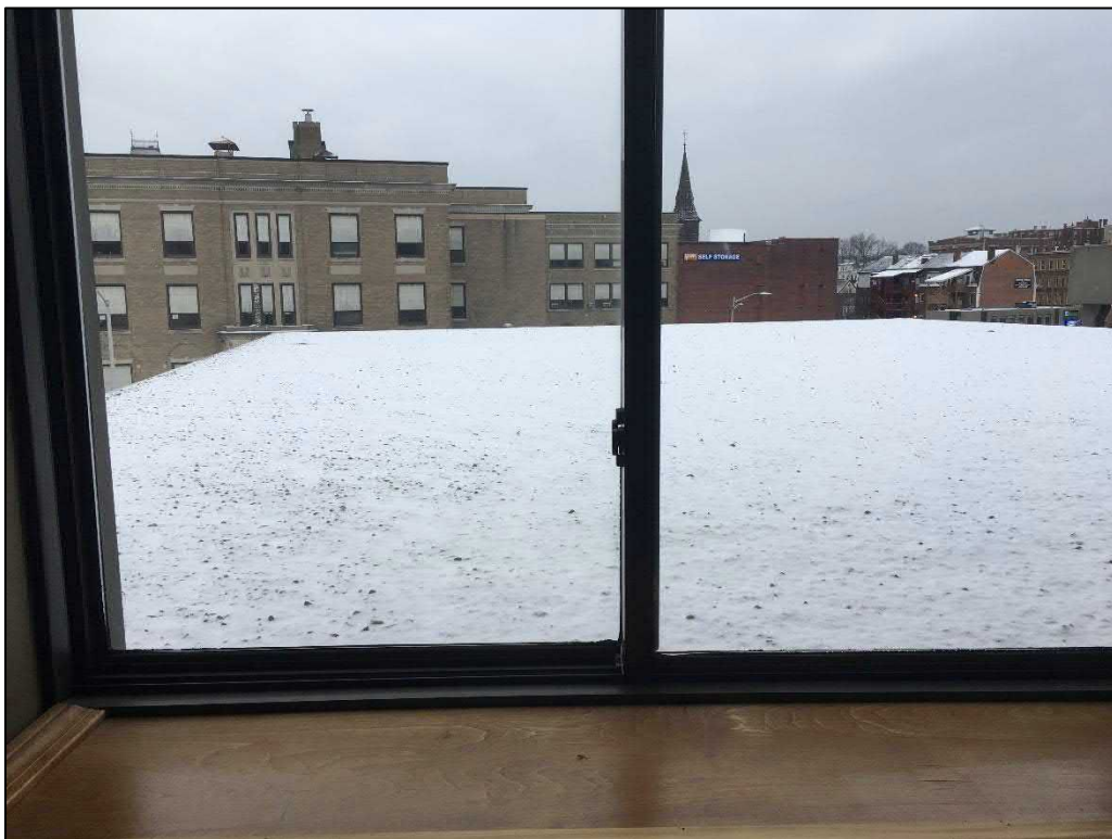
Portion of roof not recently replaced
