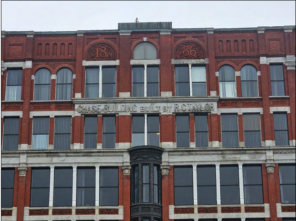
Figure 11. Detail of the Chase Building.
