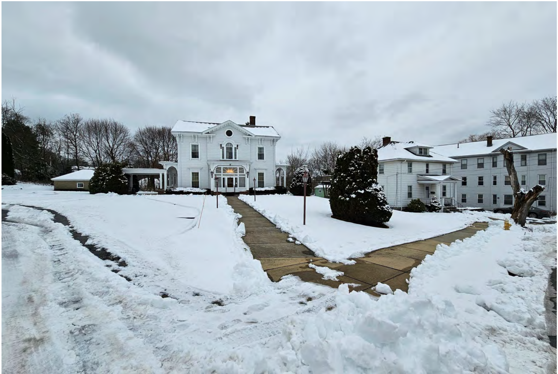
5. 36 (garage & house), 34 & 12 Butler Street (L-R), looking north.
