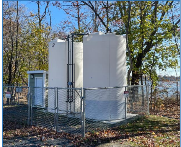
Figure 2 – In 2023, an “Alum Dosing Station” came on line at the lake’s main inlet, Ararat Brook. The station applies small amounts of the chemical, polyaluminum chloride to the mouth of the brook in small doses when it rains immobilizing phosphorous before it enters the lake.
