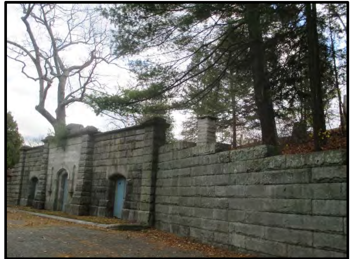
Figure 4.1.3.4 Stone Wall and Crypts Adjacent to Barn Area
