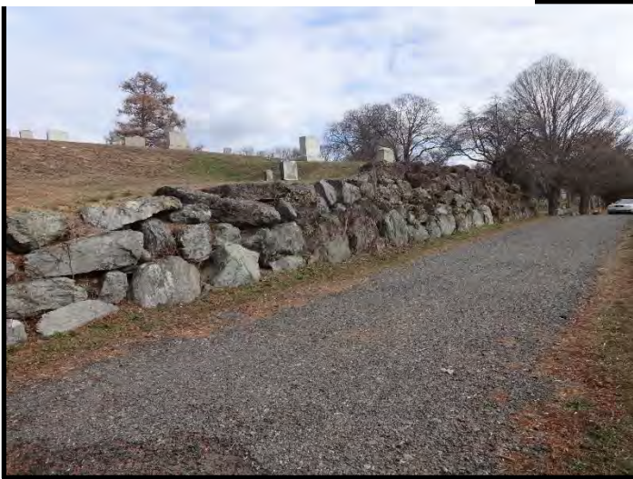
Figure 4.1.3.3 Stone Wall Along Chestnut Drive
