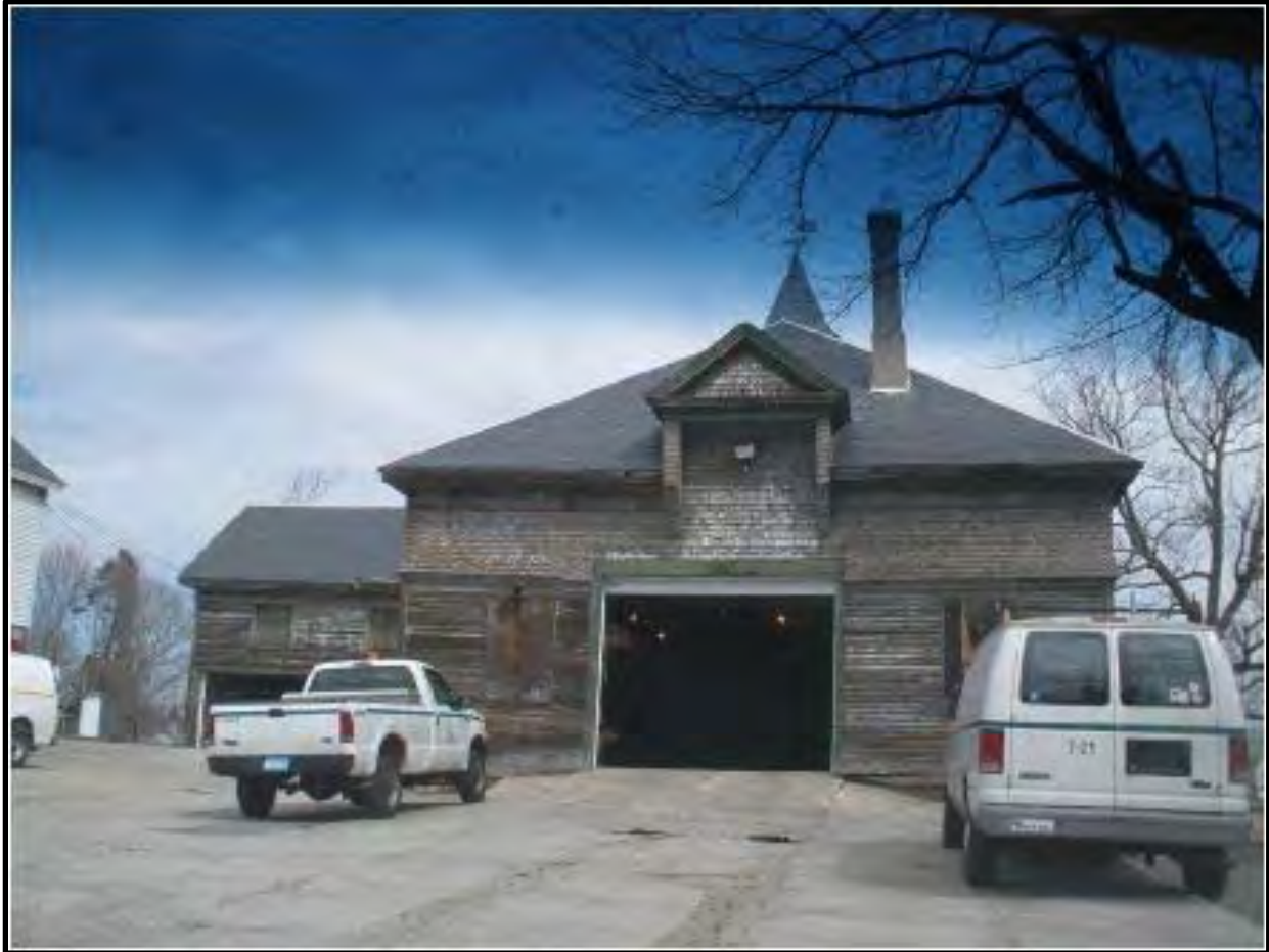
Figure 2.1.3 Wood Frame Equipment Garage & Warehouse
