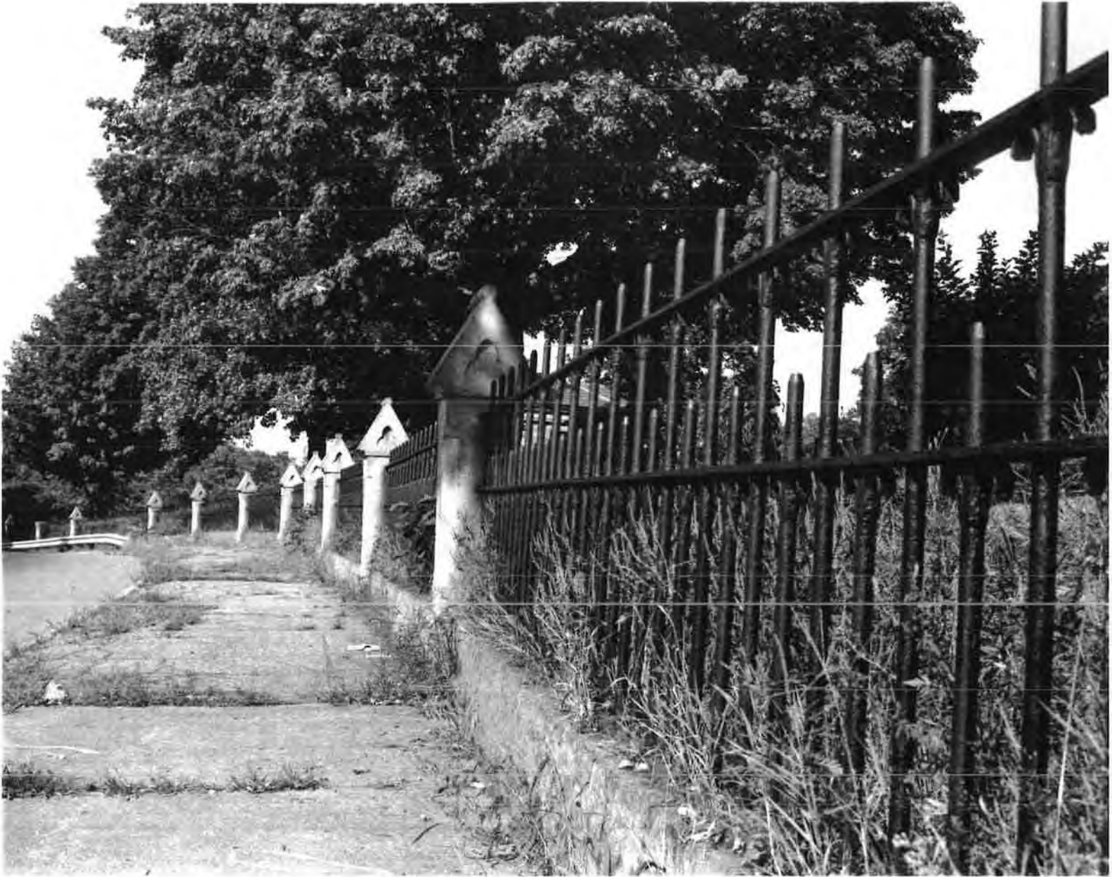
2. Original (1869) Gothic-style granite posts with incised trefoils and wrought-iron fence along Webster Street from northwest corner of the cemetery to Nixon Gates. Looking north. (Photograph: Monique B. Lehner, August 1996)
