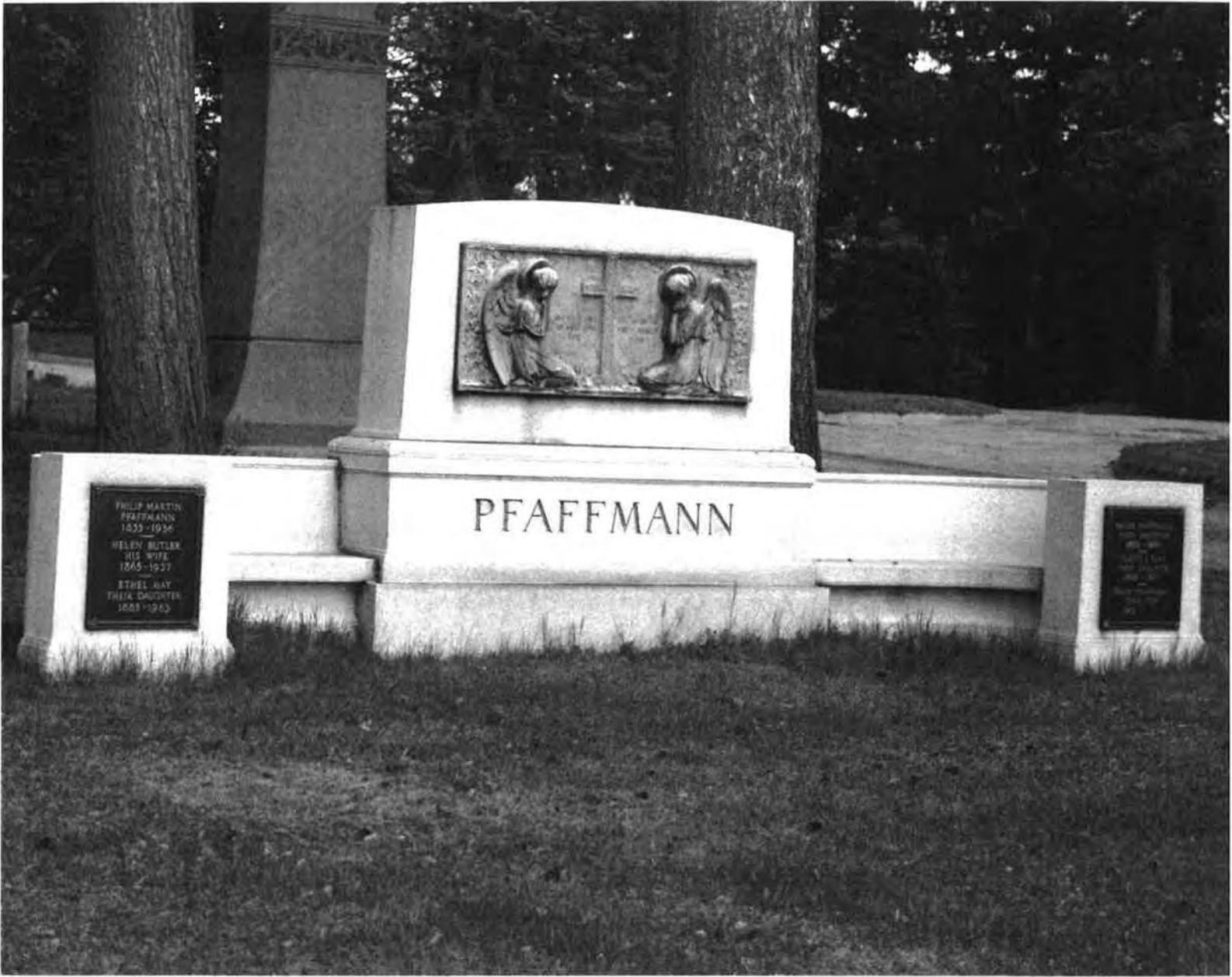
13. Pfaffman Monument (1927-1936), W.D. Kenneth, architect and J. Novelli, sculptor). The monument and exedra face west. Looking east. (Photograph: Monique B. Lehner, May 1995)
