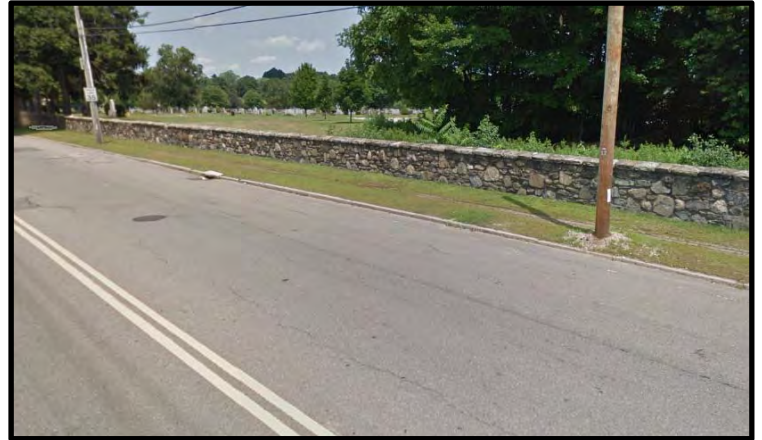
Figure 4.1.3.2 Stone Wall Along Webster Street
