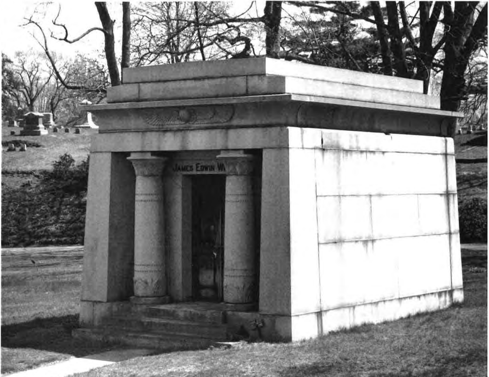
7. James Edwin Wesson, Egyptian Revival (1910), Section 12, north facade and west elevation. Looking southeast. (Photograph: Monique B. Lehner, May 1995)
