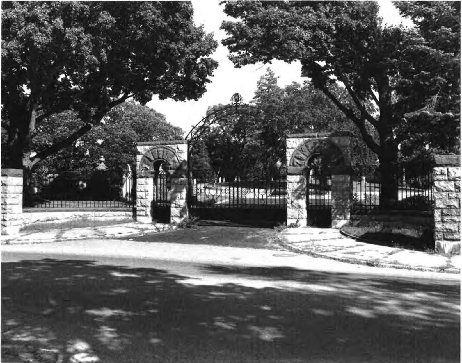
1. Wrought-iron Solomon Nixon Gates (1917; conserved 1995) located on Webster Street between Sections 1 and 39. Gates are flanked by granite arches trimmed with brownstone. Looking east. (Photograph: Monique B. Lehner, August 1996)
