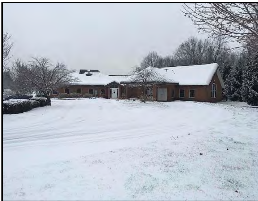
Figure 2.1.2 Main Office Building
