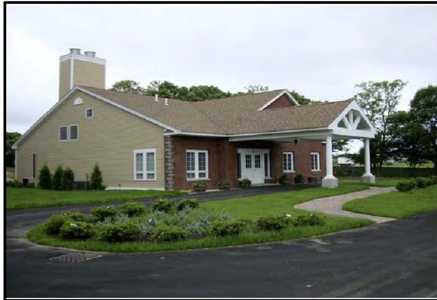
Figure 4.1.14.2 Recent Municipal Crematory Constructed in Plymouth, MA
