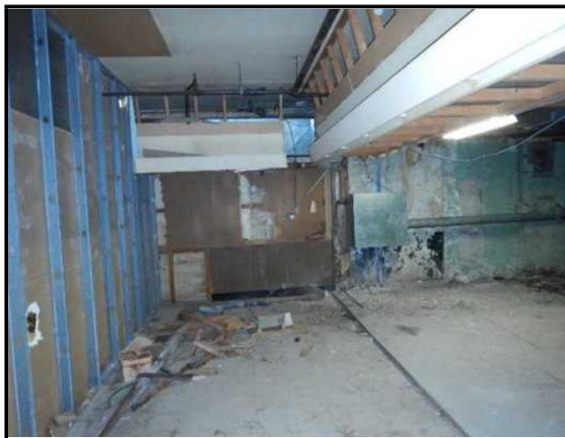
Stripped basement finishes
