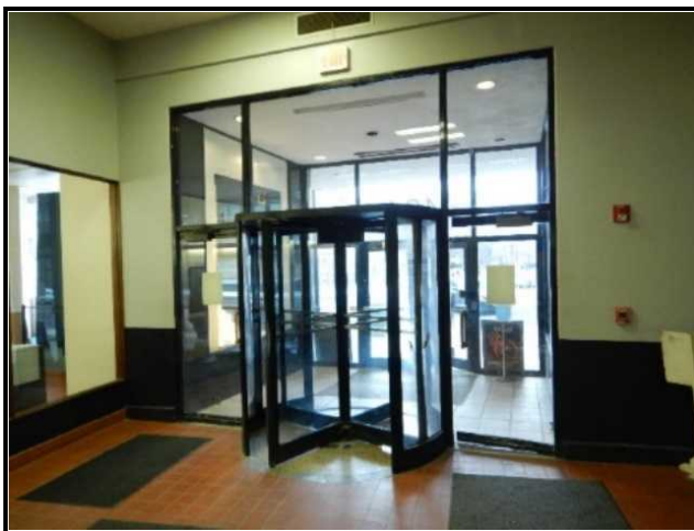
Revolving door vestibule entrance
