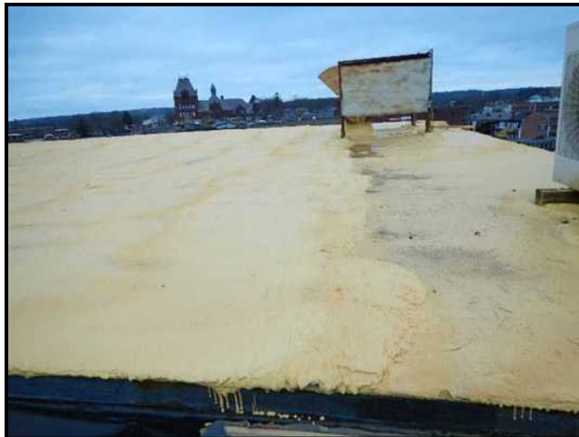
Unfinished polyurethane foam roof section E
