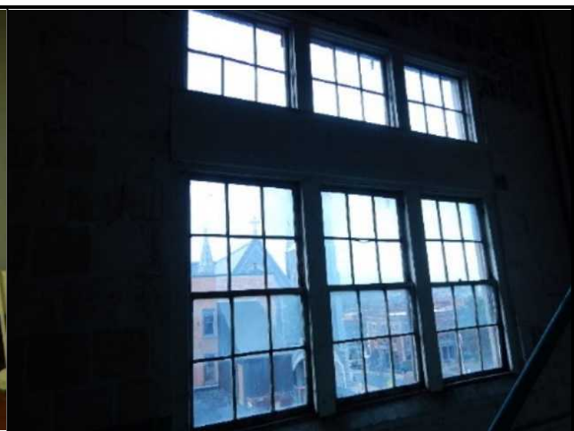
Single-pane stairwell original windows
