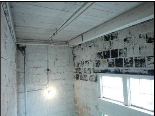
Stairwell structure showing wood roof sheathing
