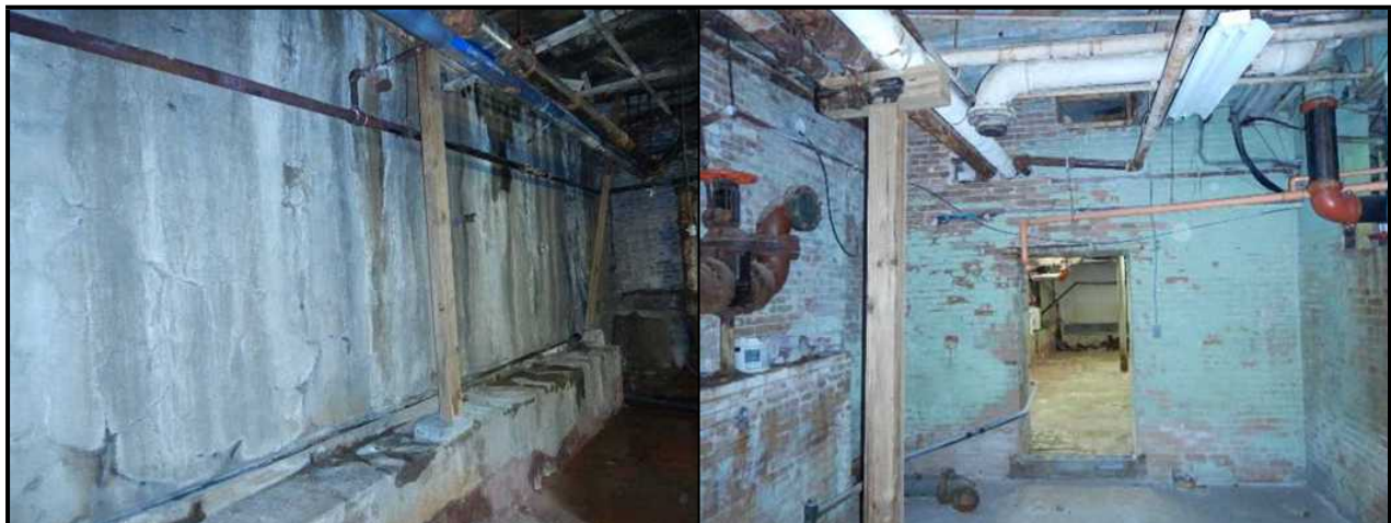
Stucco covered stone basement foundation wall at front of building
