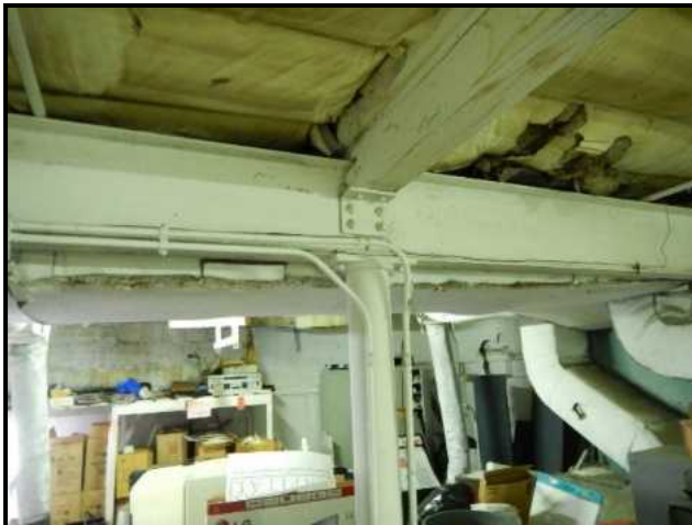
Steel and wood roof framing at 7 th floor storage space
