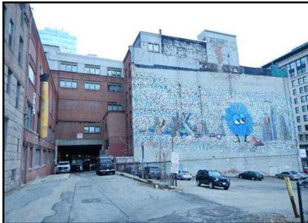
View of southern side of service alley
