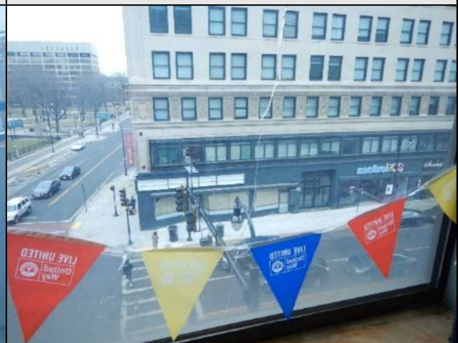
Cracked pane along eastern side of building
