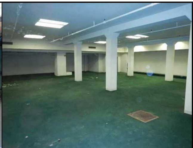
Remaining basement finishes
