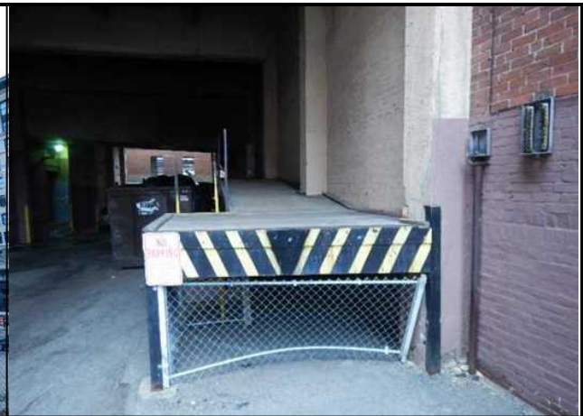
View of loading dock within service alley
