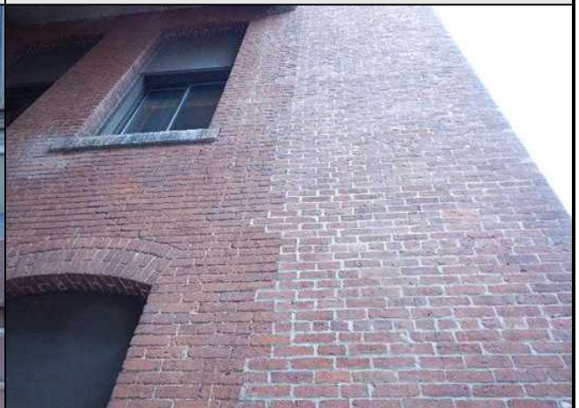
Previous mortar repointing along northern side of building
