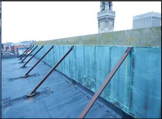
Front roof parapet wall with copper facing and steel struts
