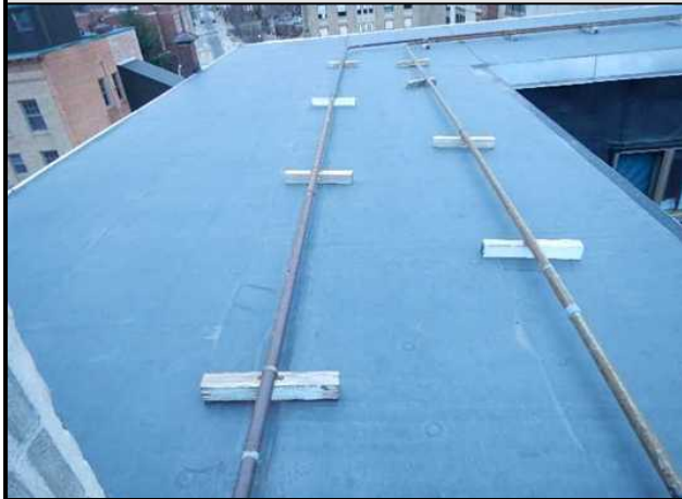
New EPDM roofing over 7 th floor entrance corridor
