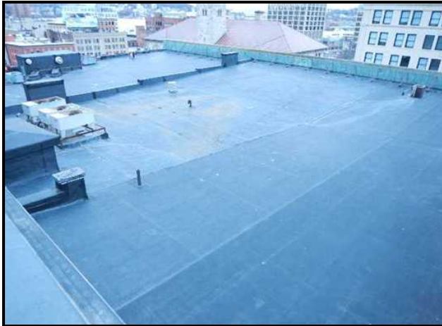
Front EPDM membrane roofing designated section A and B
