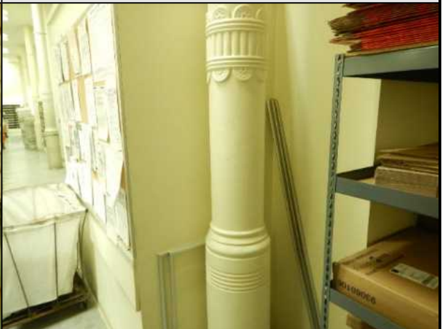
Ornamental cast iron building column visible in Post Office space
