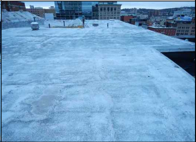
View of polyurethane foam roofing section C
