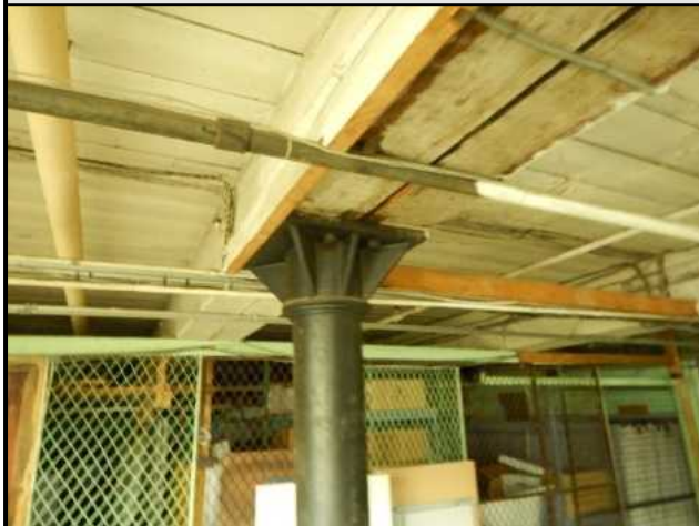
Cast iron column supporting wood framing
